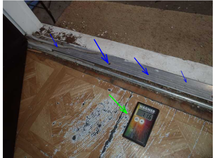
front door is noted operable..floor is noted low in moisture...appears threshold is damaged with weather stripping
