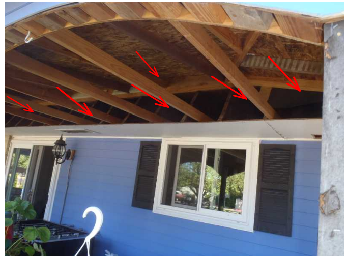
main attic at same patio covered area is noted wide open for bats and birds and critter entry..close up ASAP
