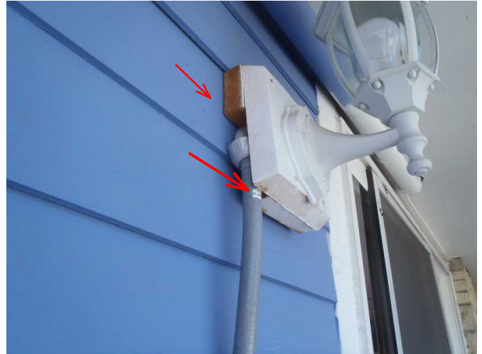
fixtures are noted tapped for exterior outlets at both sides and not recommended...correct...
