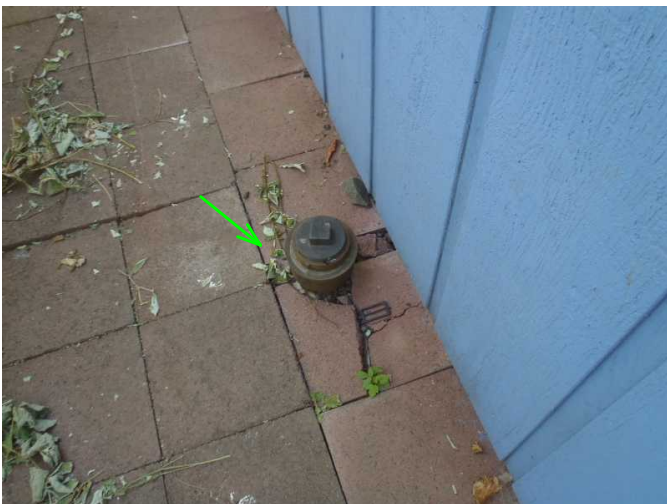
main sewer clean out for entire structure is noted at back center area by bedrooms..
