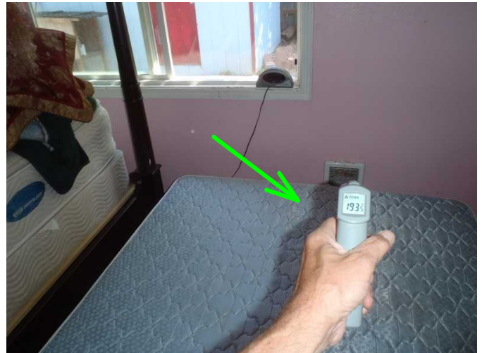
Cadet wall heater is noted operable..breaker was shut off due to bed to close to heater...
