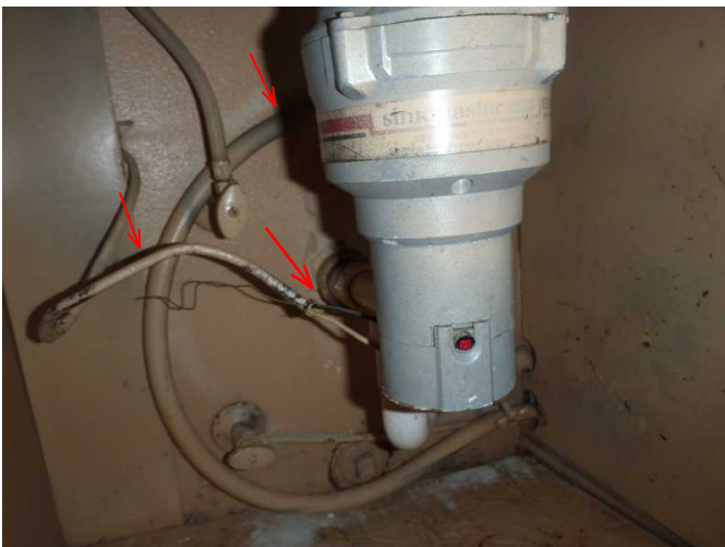
garbage disposal is noted operable..but needs armoured cable electric line...dishwasher needs high loop...
