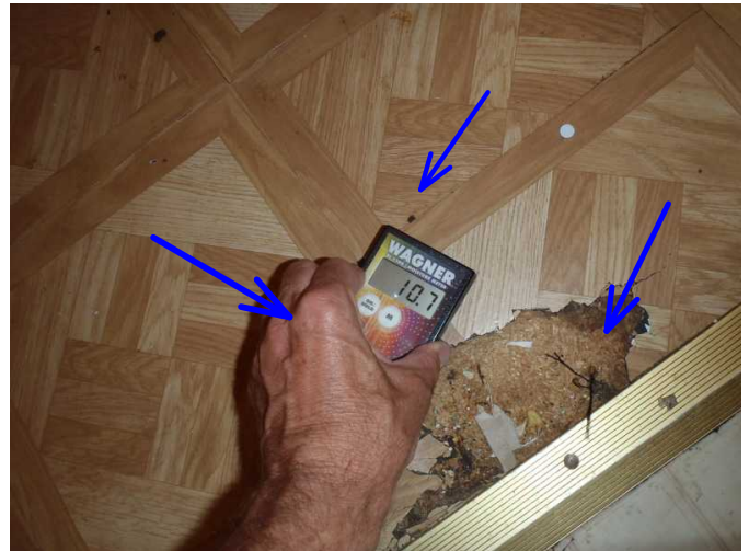
floor in dining room area is noted damaged...appears to be cosmetic...no high moisture at this time...
