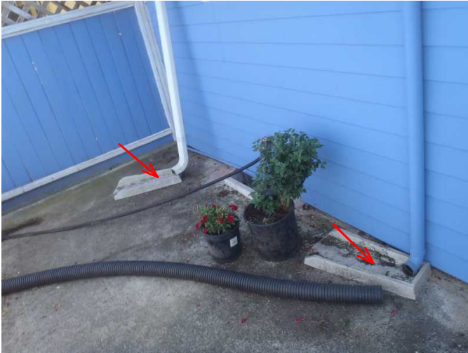
water exits are noted to close to structure..extend away from foundation....
