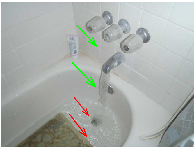
tub faucet and shower control are noted operable...but drain and drain stop are noted not operable..
