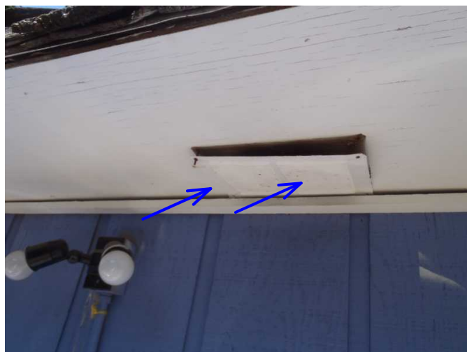
many vents are noted loose to soffits and will need secured...
