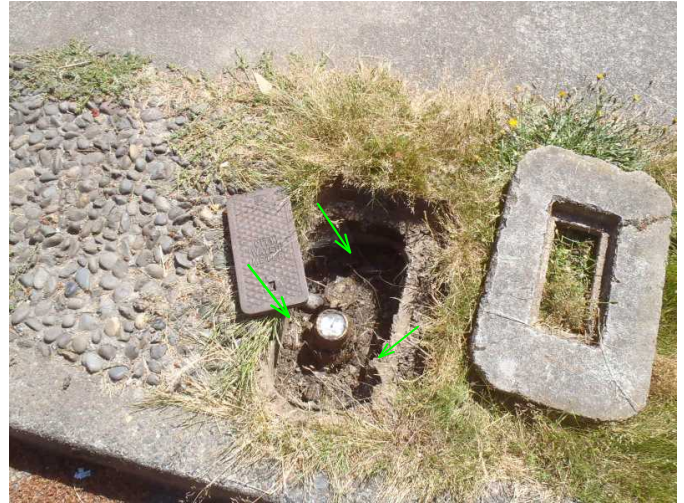
front water main and meter are noted at right of property line and main shut off is noted at meter...
