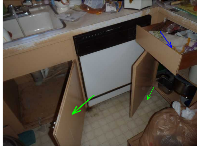
lower cabinet doors are noted operable..drawers are noted damaged...
