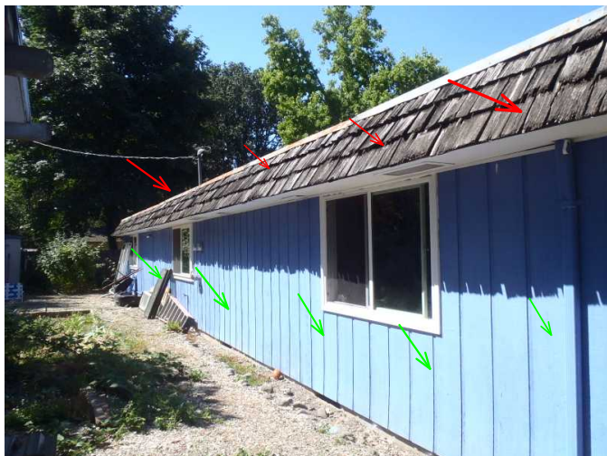
back view of T 1-11 siding is noted solid...mansard roof is noted rotted shakes...replace...
