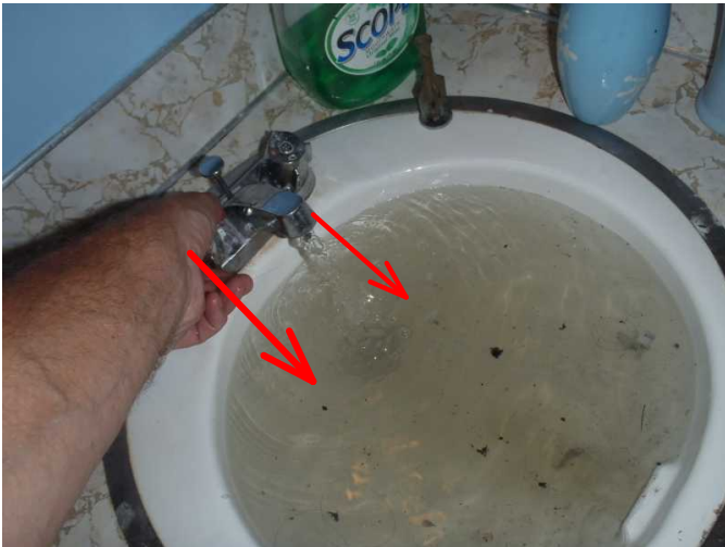
sink drain and drain stop are noted not operable..
