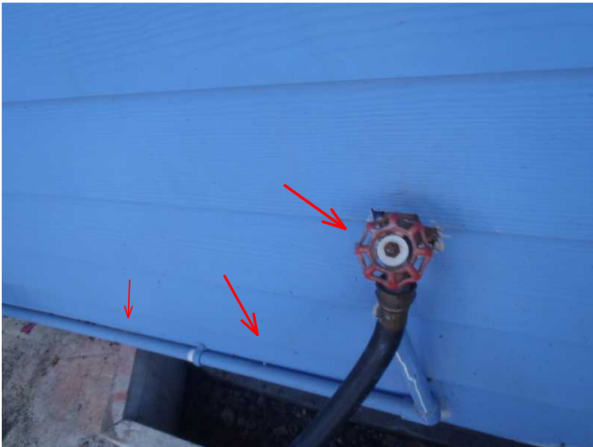
open gaps noted at hose bib and hose bib was noted not operable...some PVC tapped water lines broken...
