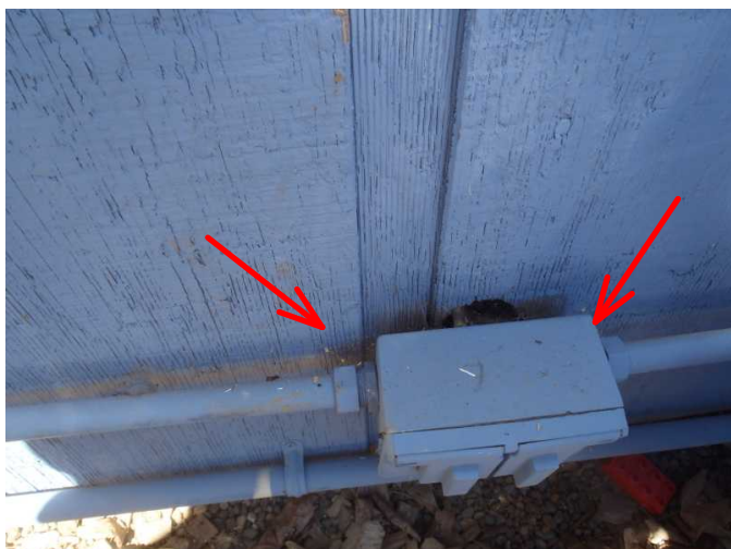
loose and open junction box is noted at back area by 11920 bedroom area...outlet is operable..secure to siding..
