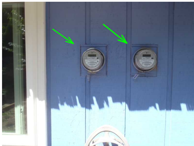
main electric meters are noted solid to siding...
