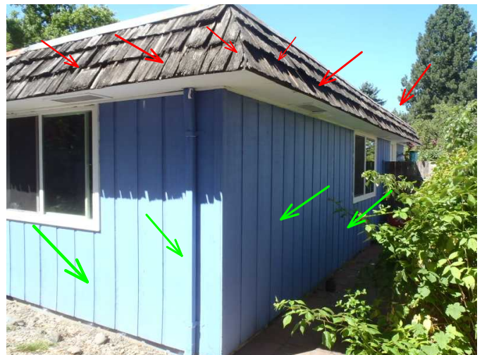
T 1-11 siding is overall solid...just needs paint...all the mansard roof shakes are noted rotted...replace, expect rot
