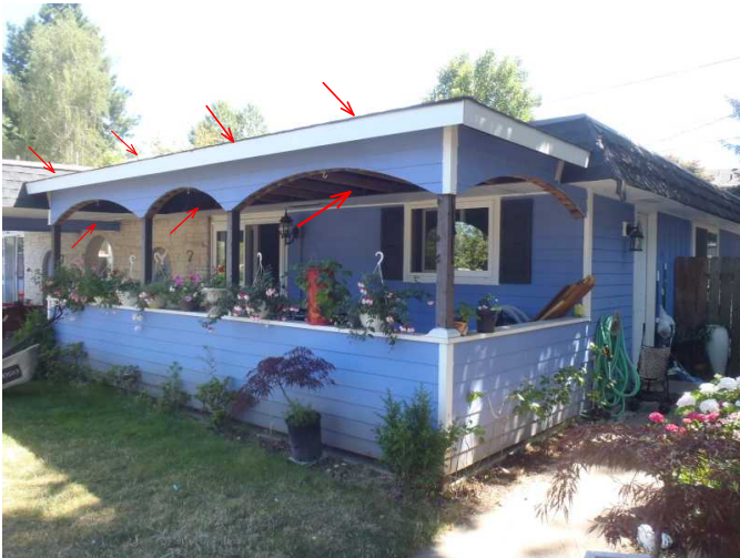
front patio is noted with added covered area...close off all open areas and add gutter and downspout to end...
