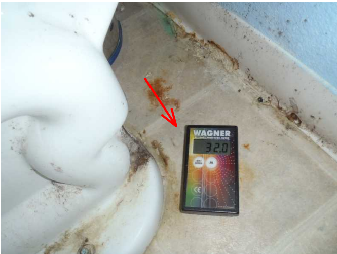
floor behind toilet is noted saturated as well...expect damages...
