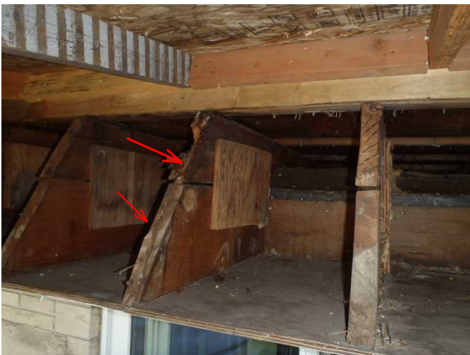
open area is also noted with random dry rot from past damage...expect added repairs at mansard roof areas...
