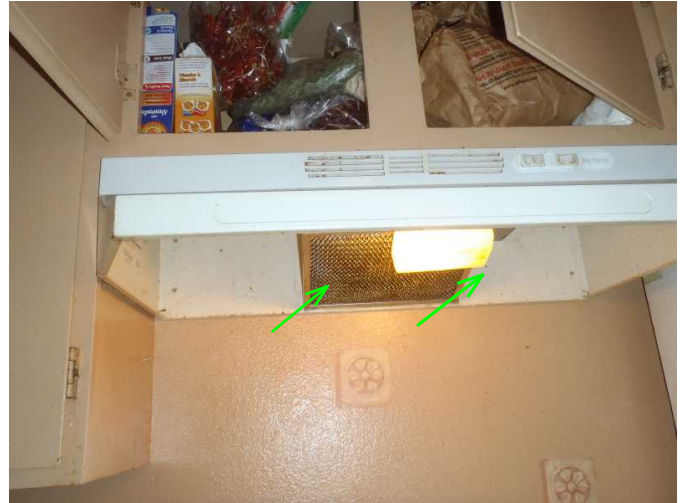
opver stove fan is recylcing...fine..exit fan is to left at wall and is operable...use both...
