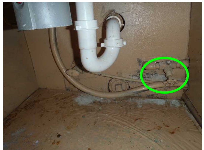
shut off for hose bib is noted in back area and has handle...
