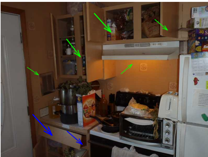
upper cabinets are noted solid to wall and operable...over stove fan is operable...as is side vent to outdoors...
