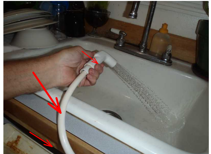
NO...the sprayer arm is not allowed to be set up as noted...will leak and cause damage..remove...
