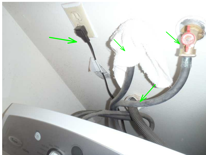
washer connections are noted drip free...
