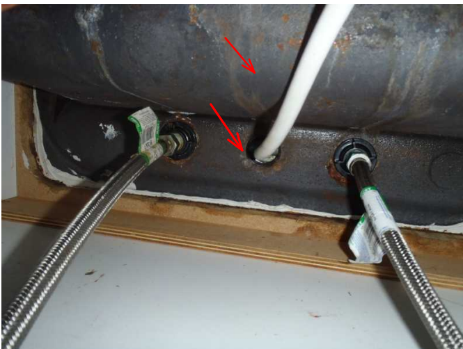
feeds off the main faucet and can at any time burst and cause massive water damage...remove...
