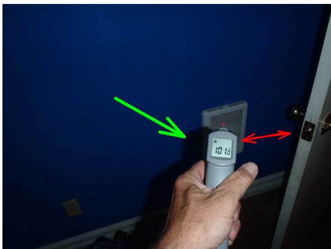
while Cadet wall heater is noted operable...it is too close to entry door and can be fire hazard...
