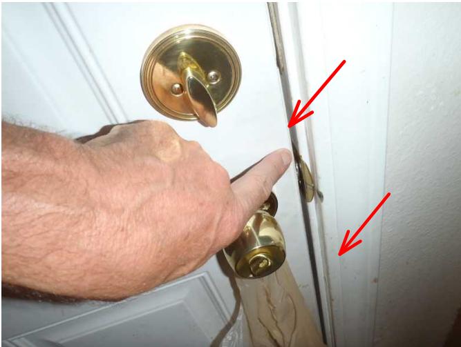
door does not latch secure and can leak cold winter air..correct...
