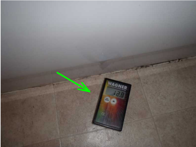
floor at tub area center at master is noted low...caulk is needed at rim areas of flooring..
