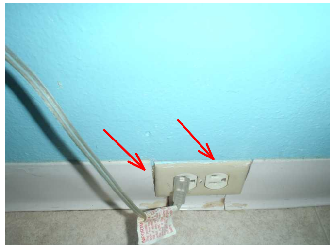
plug in main bath is at floor and not GFCI...correct...
