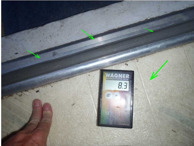
threshold is noted solid to floor and floor moisture is noted low..at front door area...
