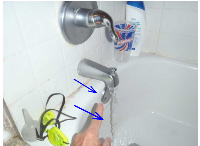
hot water is noted slow flow at master tub area...
