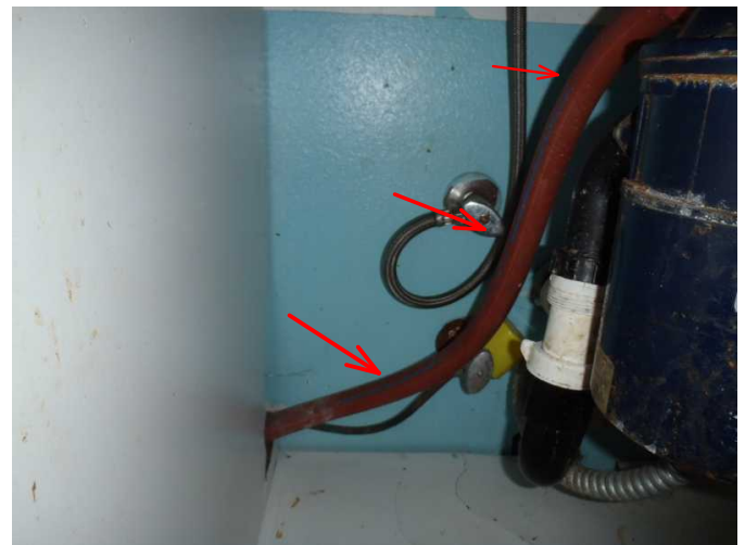
high loop is when the dishwasher drain is secured to under cabinet to not allow back flow of garbage disposal...add
