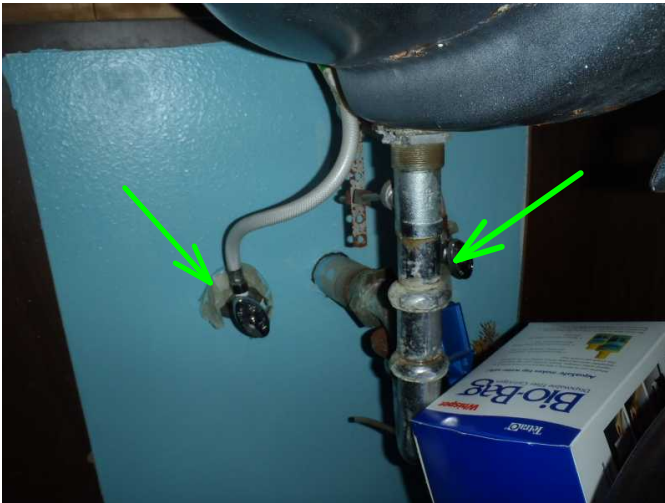
trap and connections under sink area are noted drip free...
