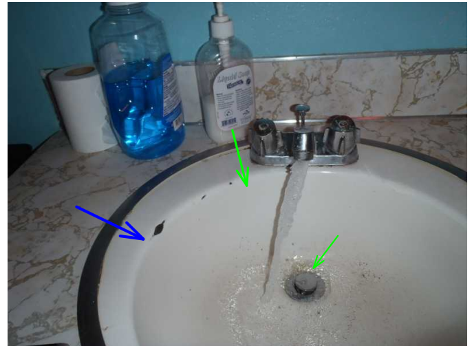
faucet needs repairs and sink has surface damage...drain is operable...but drain stop is noted not operable..
