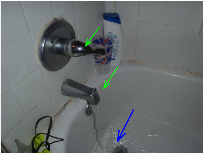
faucet is noted operable...but drain stop not operable...
