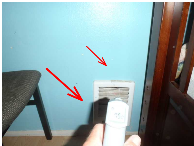
Cadet wall heater in this room is noted not operable...replace...
