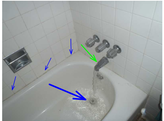
tub faucet is noted operable..drain stop not operable...monitor grout at tile walls...
