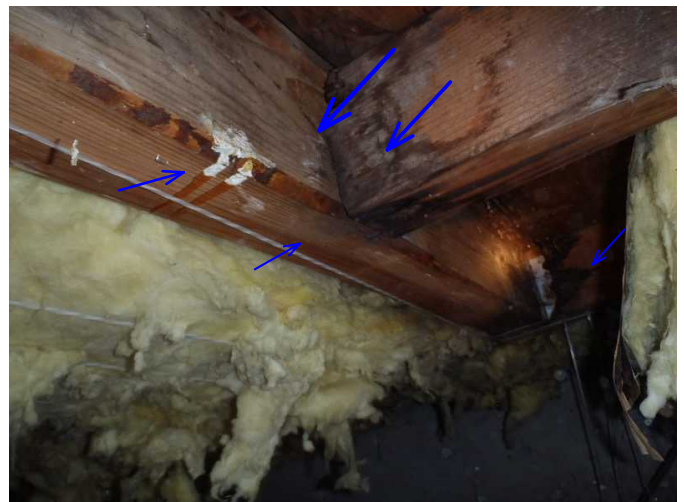
some beams are noted with staining and are noted solid...repairs were performed...
