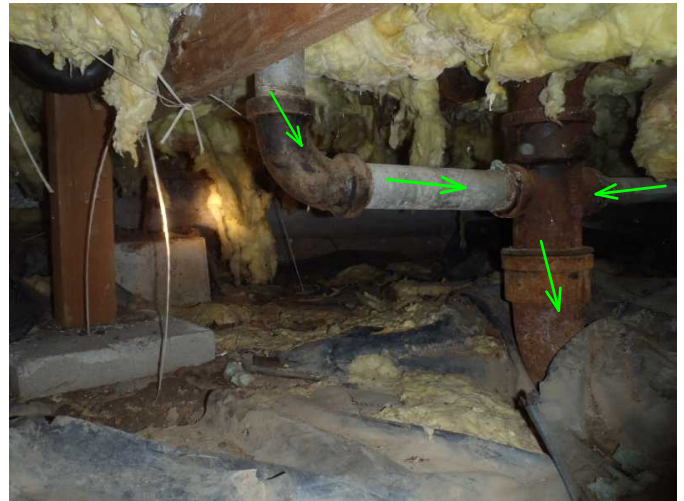
11920 bath exit drains are original and noted no drips or leaks below as well as in area...
