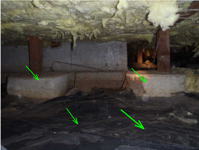
all of crawl is noted with vapor barrier and posts are raised and dry...and solid on piers....
