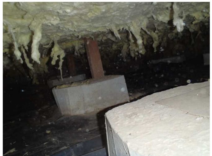
more downed insulation noted...appears was past issue...and vents were closed up, but repairs not performed...
