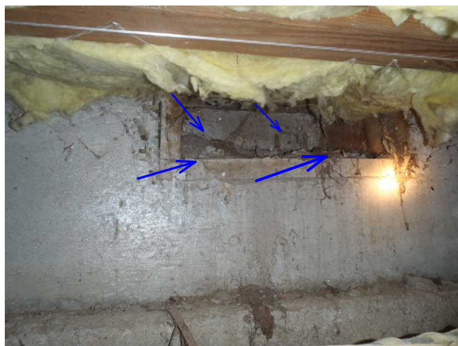
here is vent in front of home that needs screen...is covered with wood..but is recommended to be kept open to vent air...
