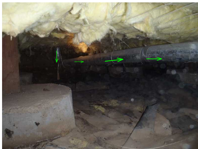
dryer vent is noted with no lint leaks and solid from laundry to exiting area at back of home...
