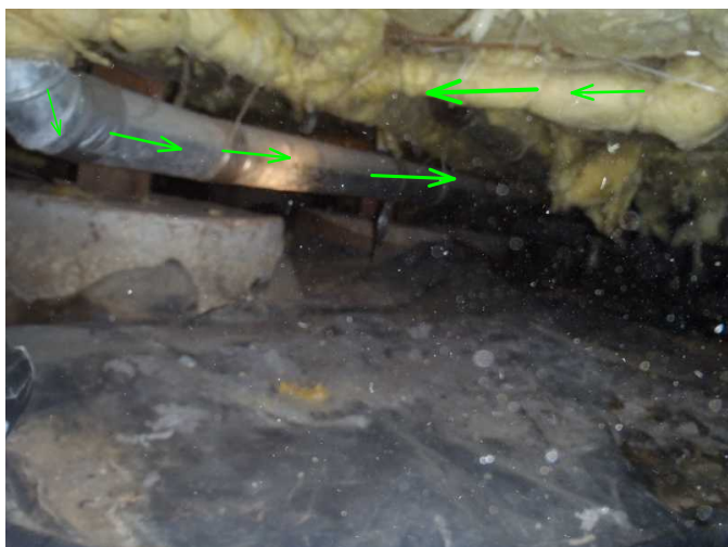
most all water pipes are noted here insulated...and 11900 dryer vent duct is noted solid to exit as well..
