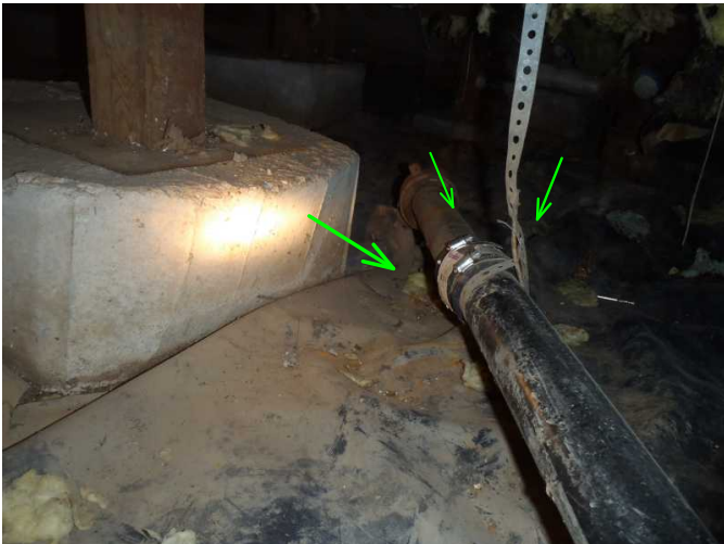
ABS meets original sewer exit drain and is noted clamped as needed...good...no drips or leaks...
