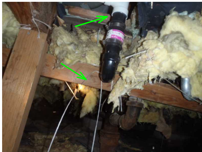
here is same area under 11920 tub area and has new ABS trap as well...
