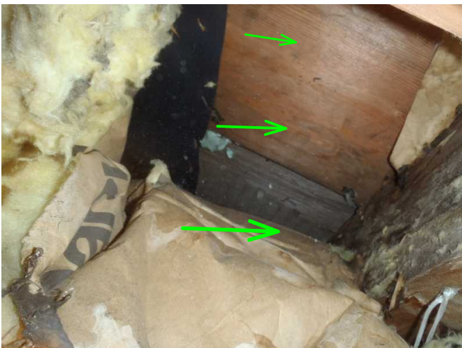
some areas are noted with flooring replaced with plywood under bath areas in 11920 sub floor area where insulation down...
