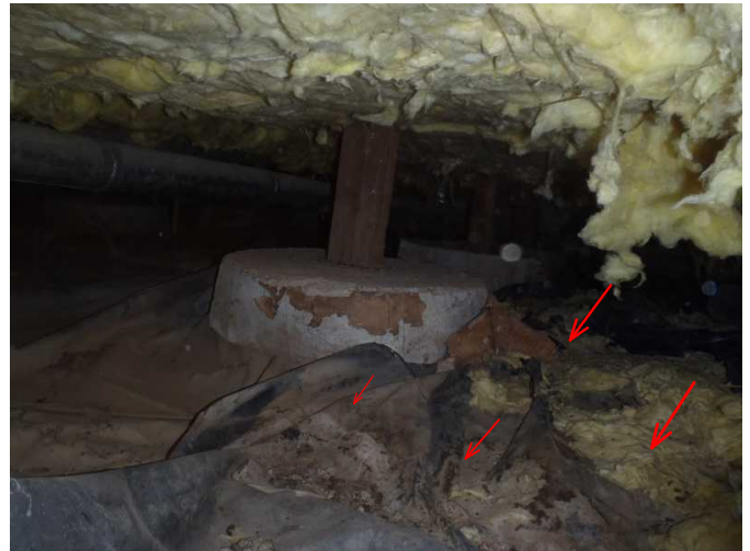
more downed insulation noted...appears was past issue...and vents were closed up, but repairs not performed...
