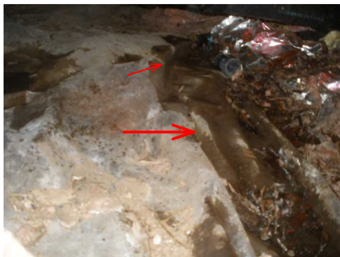
vapor barrier is noted with standing water at leaks under floor at bath and at foundation areas...
