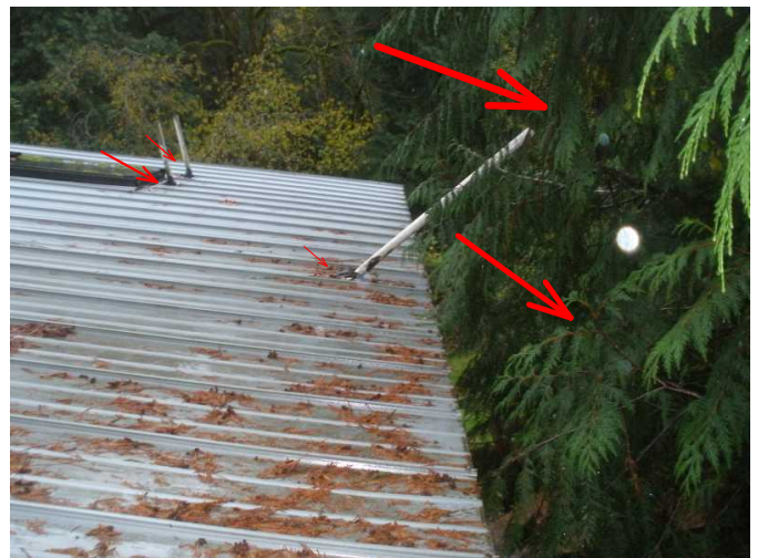
assess flashing at all sewer vents...appears damaged...cut back tree branches 6- 8 feet from structure...
