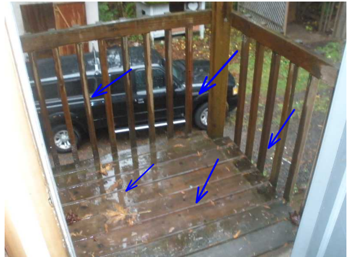
mini balcony appears solid. but needs cleaned and sealed...monitor at all cantalevered beams
