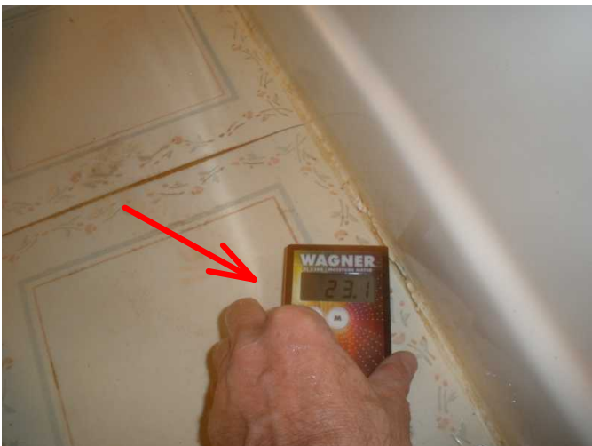
high moisture noted at tub floor...may be from tub or from siding issues...
