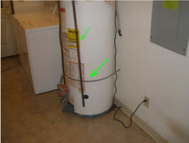
unit is strapped to wall and solid...
