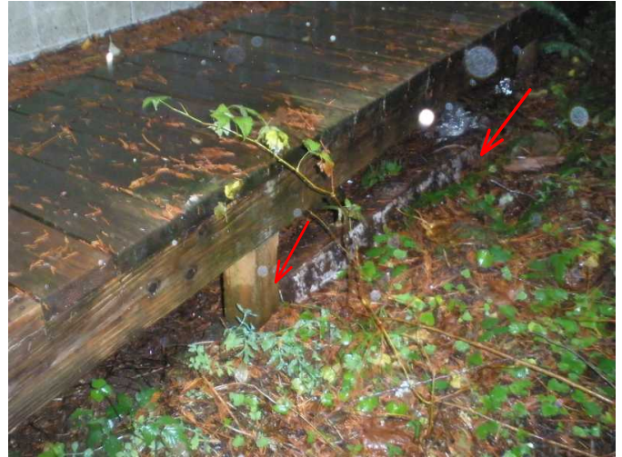
most posts at deck are noted rotted and have earth to wood contact...
