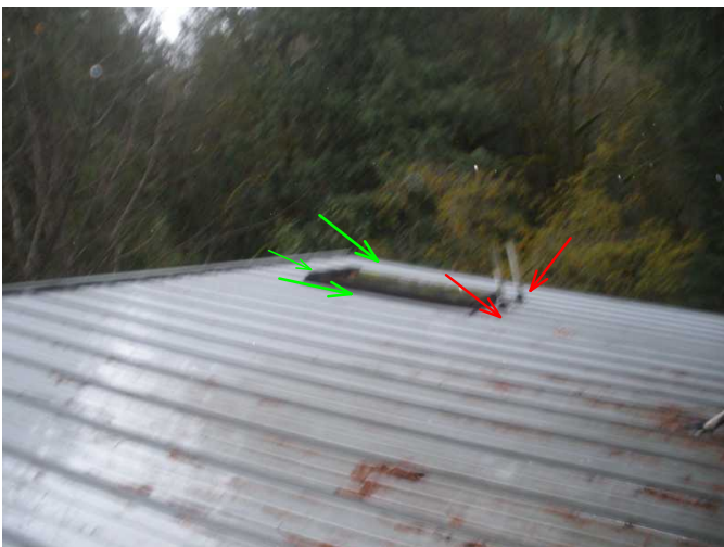
skylight flashing appears fine at south roof area over bath..and upper sewer flashing need assessed with lower damaged..
