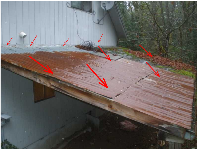
back roof area needs replaced and recommend adding flashing at roof to siding to avoid added rot...
