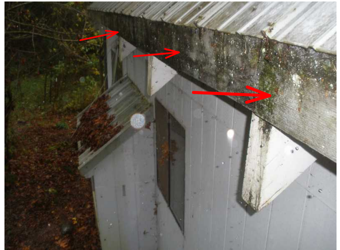
fascia board noted rotted and will need gutters installed...north side...
