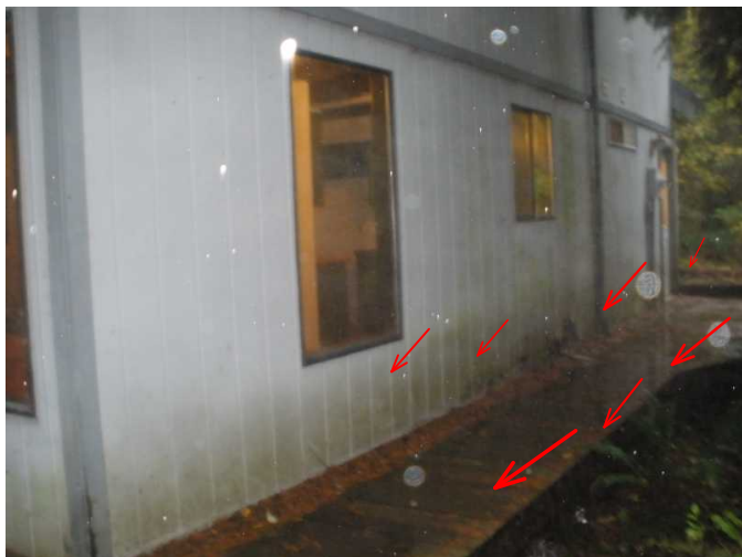
south deck and siding noted rotted and will need extensive assessment and repairs...
