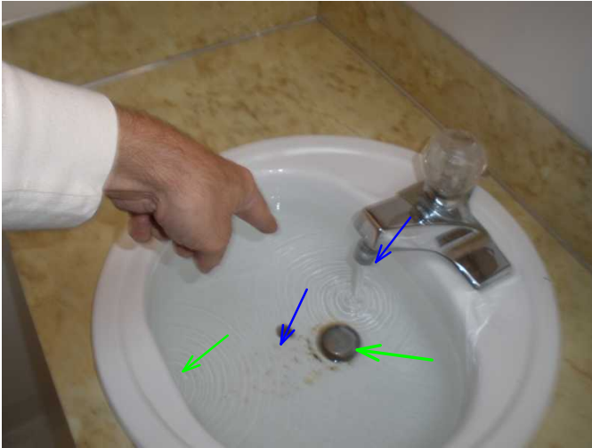
low flow noted at faucet and drain and overflow are noted operable..and surface damage noted at sink...
