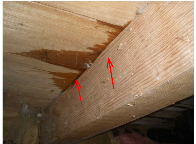
beam and sub floor are noted wet here under laundry area...
