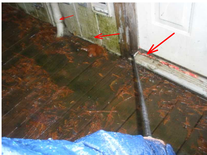
rot noted at base of back laundry door frame is noted...
