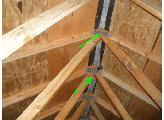
roof has ridge vent system..and is screened...good...
