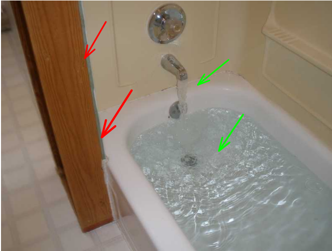
upper bath tub faucet and overflow and drain are noted operable...recommend removal of untreated wall area..
