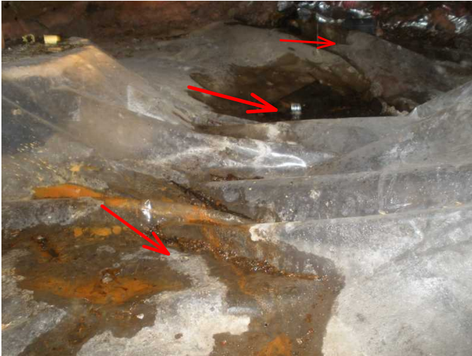
vapor barrier is noted wet....
