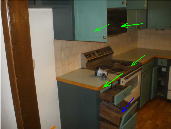
upper cabinets noted operable...lower cabinets noted loose at drawers...
