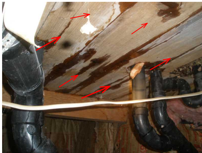
this is under bath and laundry room area....the sub flooring is noted damaged and wet and mold has started...
