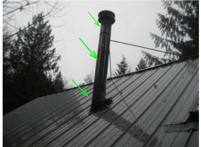
chimney at roof at north side is noted fine...monitor and assess flashing every fall before winter...appears fine
