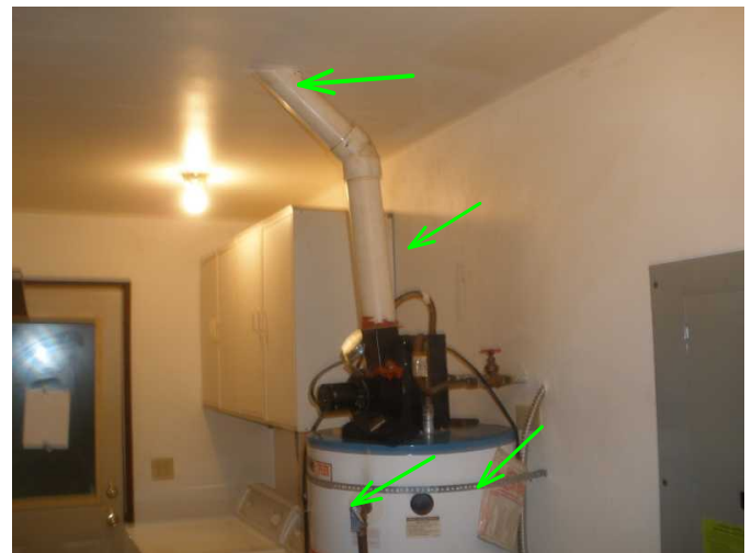
water heater flue is noted PVC and is high efficiency unit..did not test...no gas...
