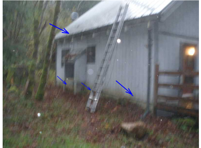
lower area at north side noted stained, but no rot noted at this time..add gutters and then paint
