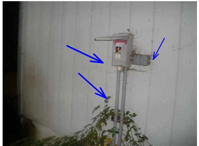
spa tub disconnect is noted here and outlet noted not operable...
