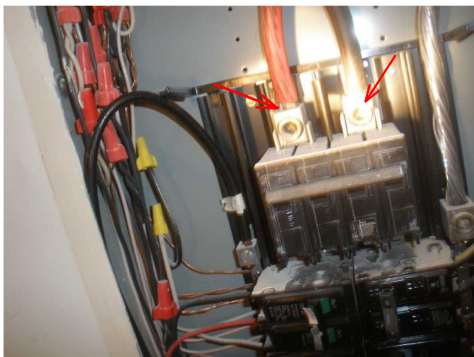
add anti oxident paste to service entry conductors...
