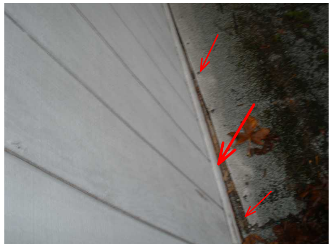
this is looking out window at back roof...add flashing and new roof...
