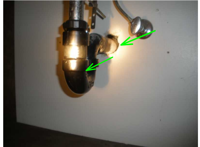
no drips or leaks noted at sink trap and connections...good...
