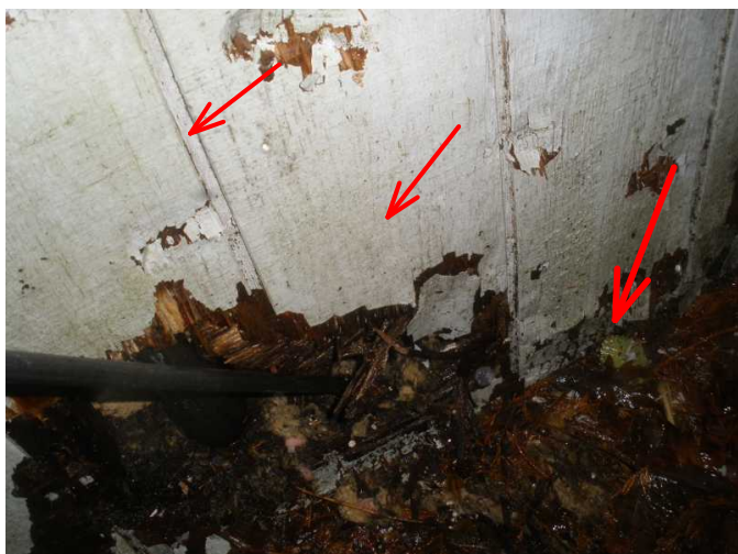
open gaps are allowing water entry and the gutters missing at upper eaves appears to be the cause....massive water falls
