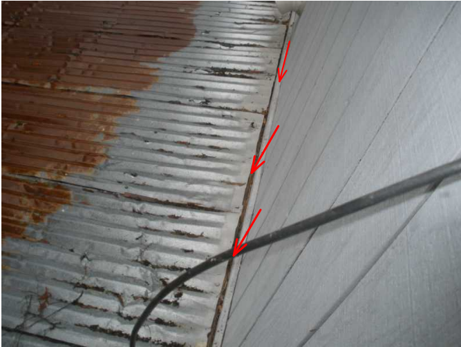
no flashing noted at back roof area...add...
