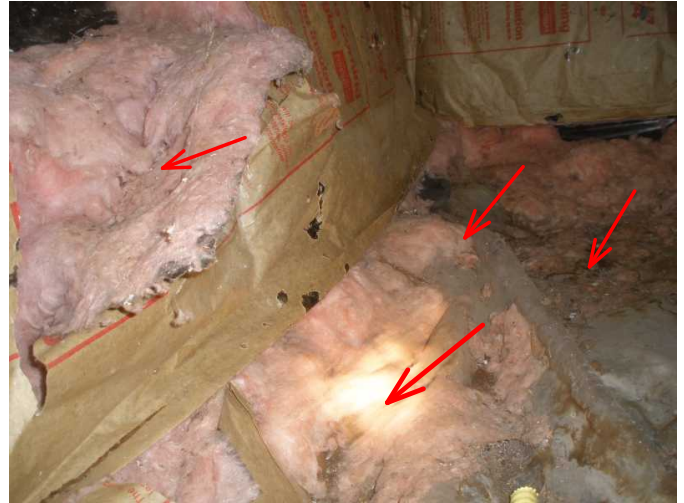
downed insulation is noted under corner area and has nesting noted as well...rats most likely...
