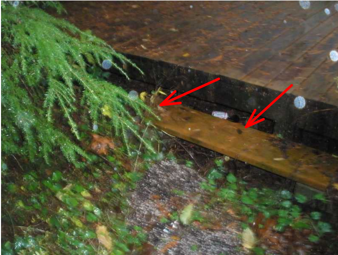
stairs at side to yard are rotted..replace...
