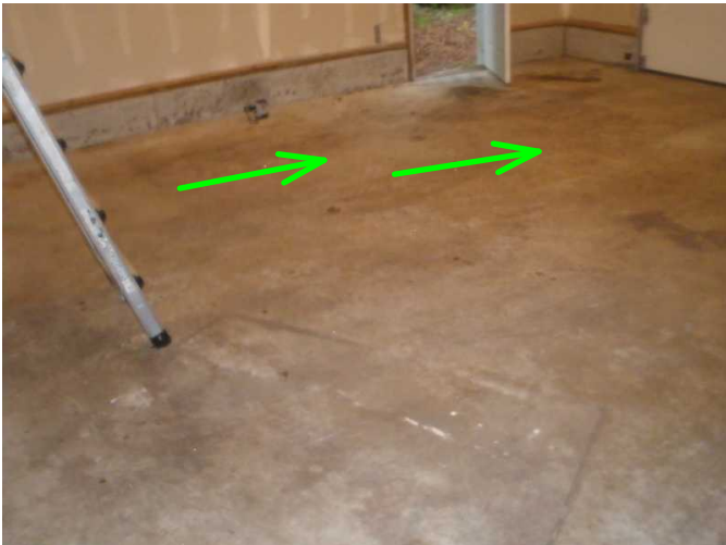
poured garage floor is noted sloped well for drainage toward overhead door area...
