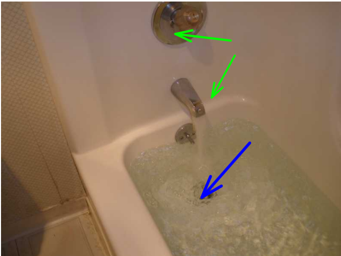
tub faucet and drain and drain stop are found operable..drain stop need repaired..does not drain well...drains slow....
