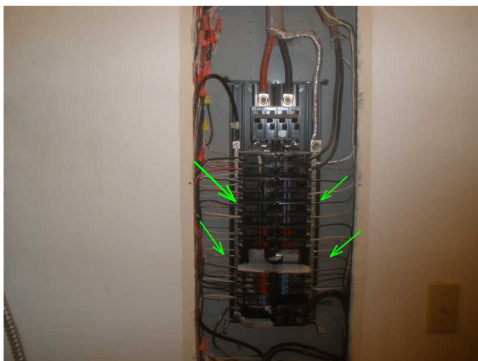
open view of panel is noted with 200 amp aluminum service and is original panel...
