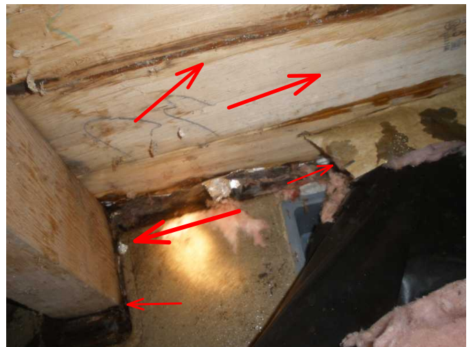
main beam into foundation here is wet and may need replaced...floor at foundation is soaked and rotted..
