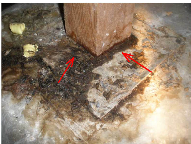
this is standing water at area below affected area with rat fecal matter in water at post...replace post and remove
