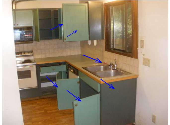
cabinets will need to be removed to assess damaged wall from moisture...
