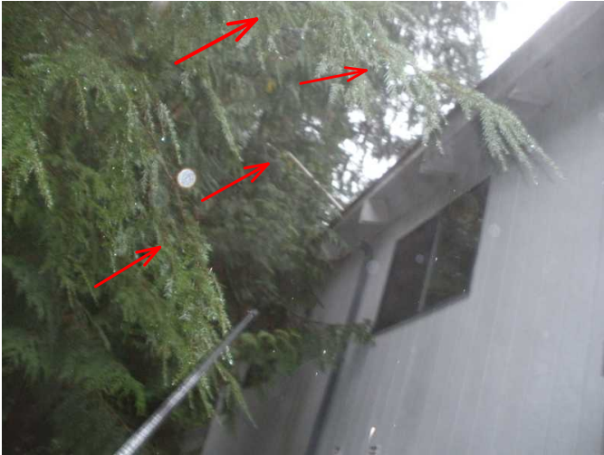
missing fascia boards at upper roof area...and cut back tree branches 6- 8 feet from structure to monitor home...
