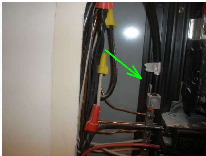
noted the ground to sub panel in neutral bar area...good..
