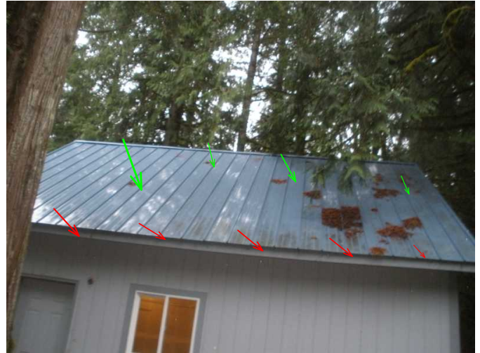
both sides of roof are noted fine, recommend cleaning.....add gutters for best water control at any structure...
