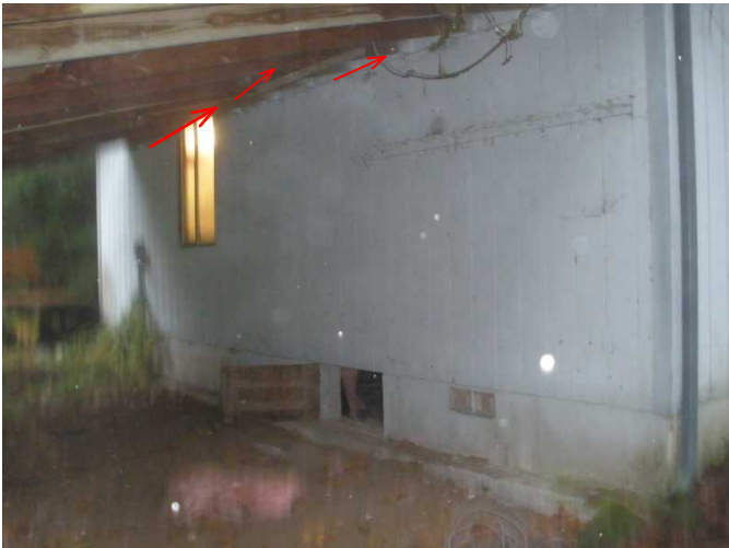
back roof extension is noted not flashed and needs lags to secure to structure...has roof rafter hangers...
