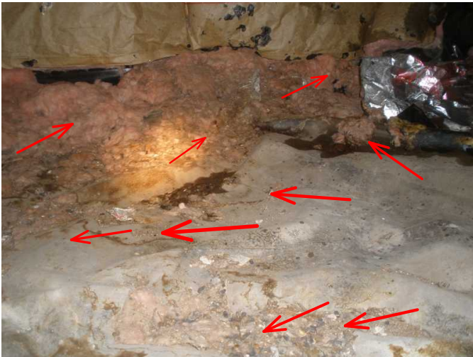
soaked insulation is breeding ground here for vermin and contamination...fecal droppings noted around flooring...
