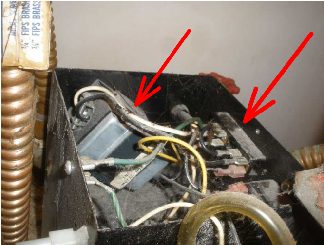
close top of water heater to contain electric connections...
