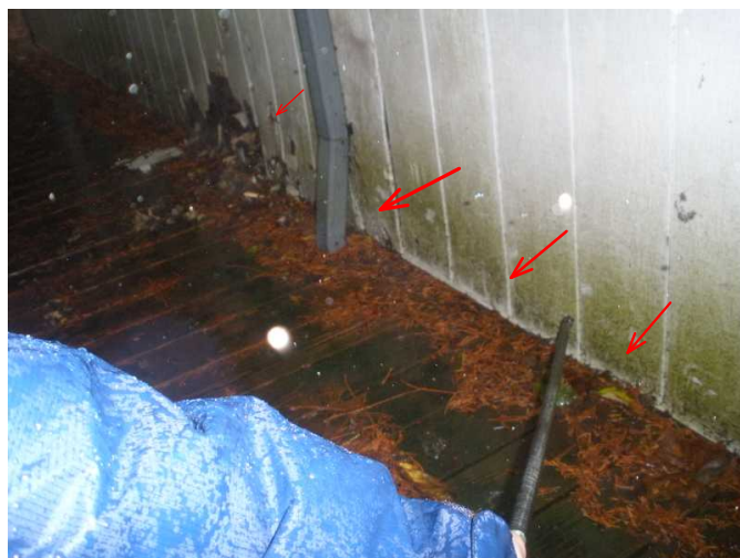
the lower areas where not even seen open are found rotted...
