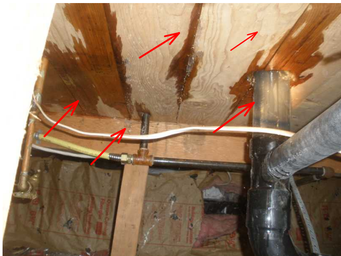
the planks under bath area at toilet and sink and tub are noted here....
