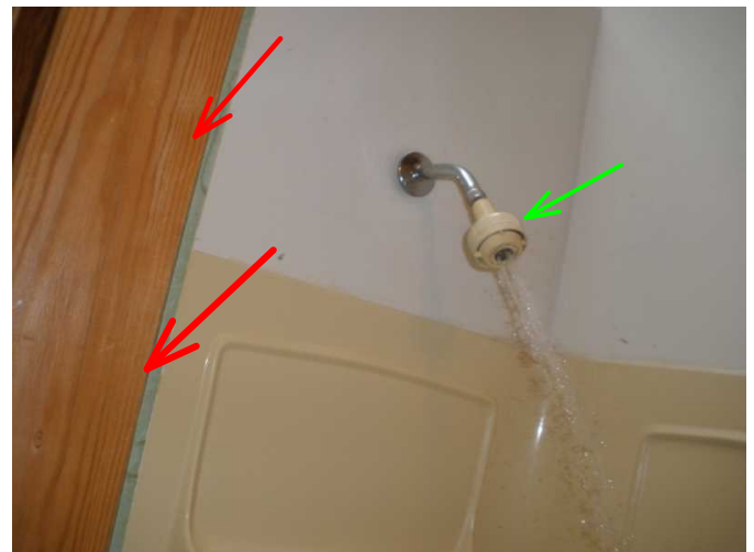
shower head is noted operable...recommend removal of added wall with no water proof finish...
