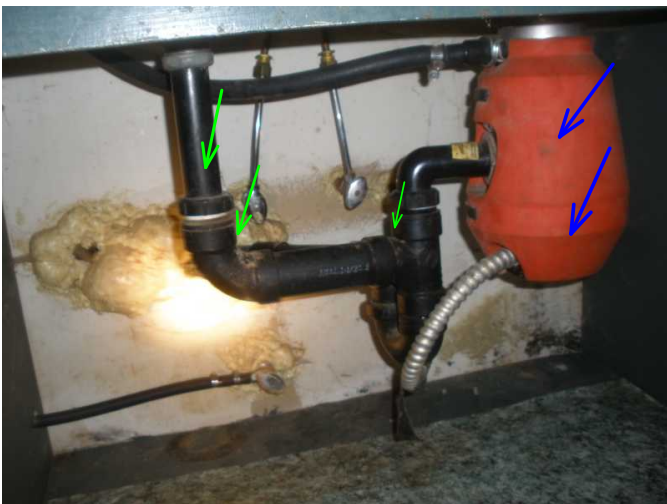
no leaks noted under sink...garbage disposal not recommended with septic system...
