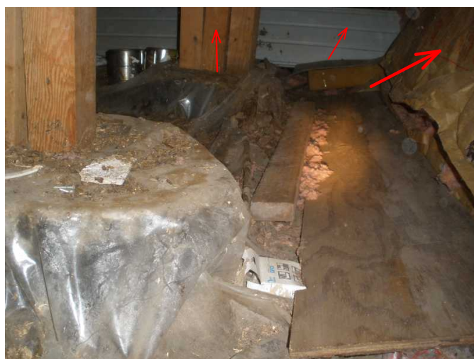
the perimeter flooring and walls at south area will need assessed and replaced to remove all damaged structure
