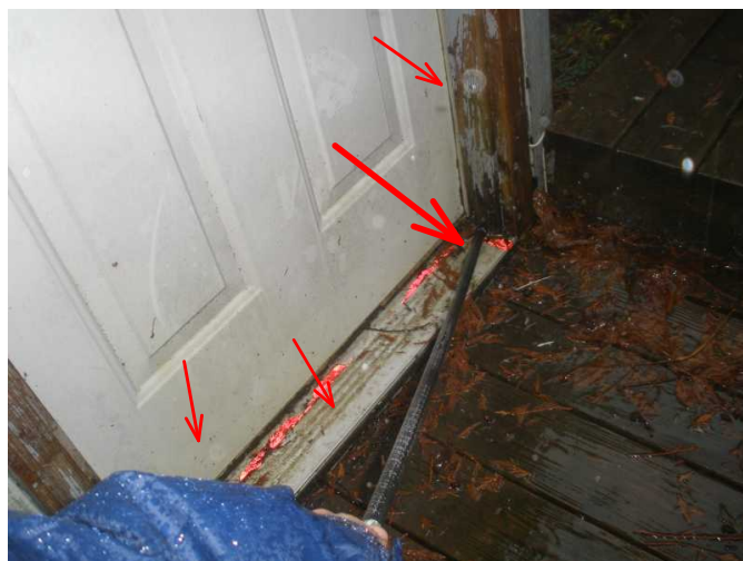
both sides of door frame are noted rotted..also noted water flowing into laundry room at door threshold...
