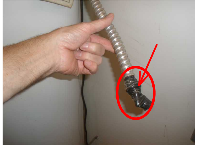
loose wiring from old electric water heater must be removed..is standard practice and is not allowed to have any loose
