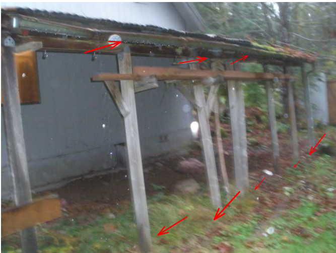
replace gutters and downspouts and pull back all earth to wood contact at base poles...
