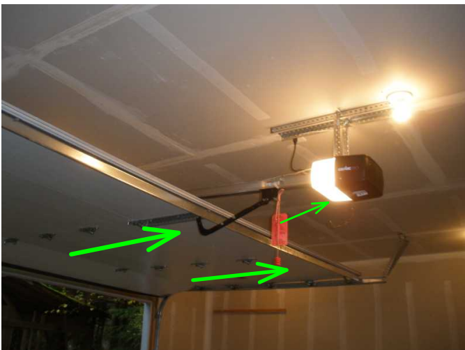
overhead door opener and overhead door are noted fine...operable...and auto reverse is fine...
