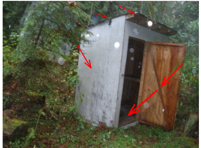
backout buidling is noted with random rot as well..repair as needed...roof needs replace on all outbuildings...
