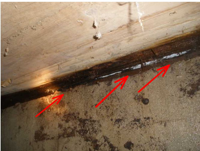
this took some work to pry off the foundation...but here is the wood plank flooring along foundation rotted and soaked...
