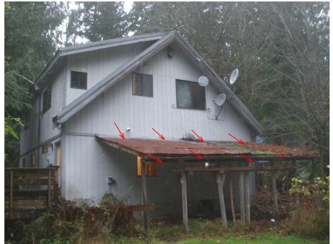
roof and gutters at back are noted damaged and recommend replacement...add flashing to roof to siding area...
