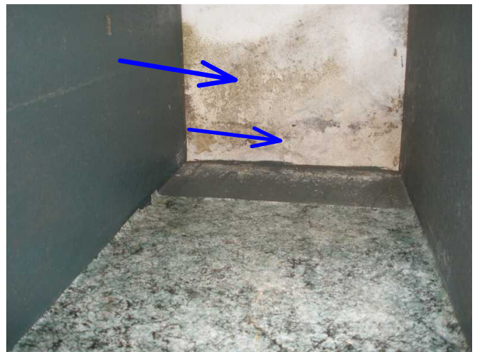
black mold noted at lower walls inside outer wall cabinets..
