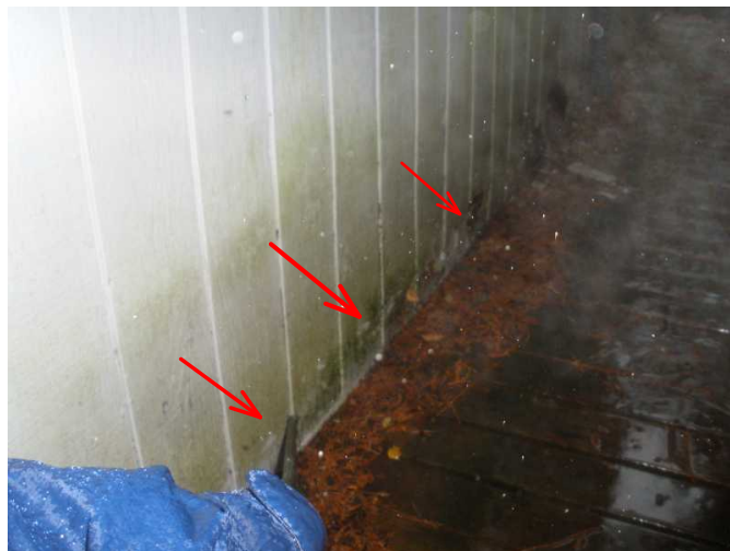
rot starts at area under dining room window and will need all of siding removed and assess damage to framing and floors
