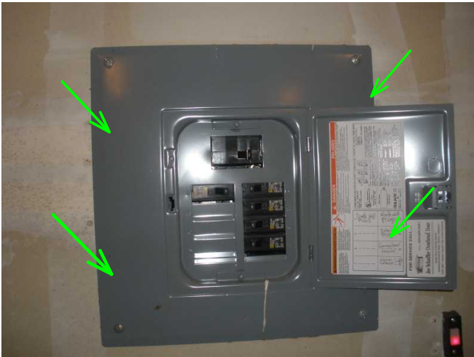
here is sub panel at garage exterior wall by exit door,,, noted with no permits..but appears professionally installed..
