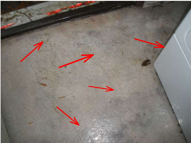
back door threshold is leaking water into area..floor is noted warped and discolored...remove all and assess...
