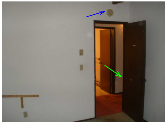
entry door noted operable..smoke detectors need updated and raised to ceiling areas...
