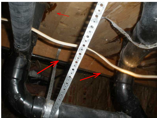
the area at foundation is noted wet at sub floor....
