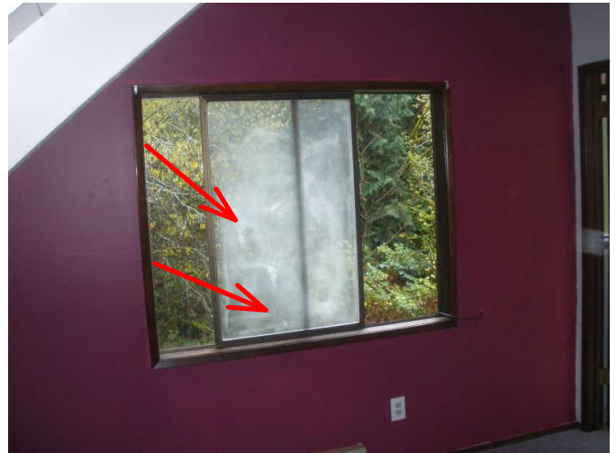
now at upstairs back bedroom showing window has broken seal..correct...
