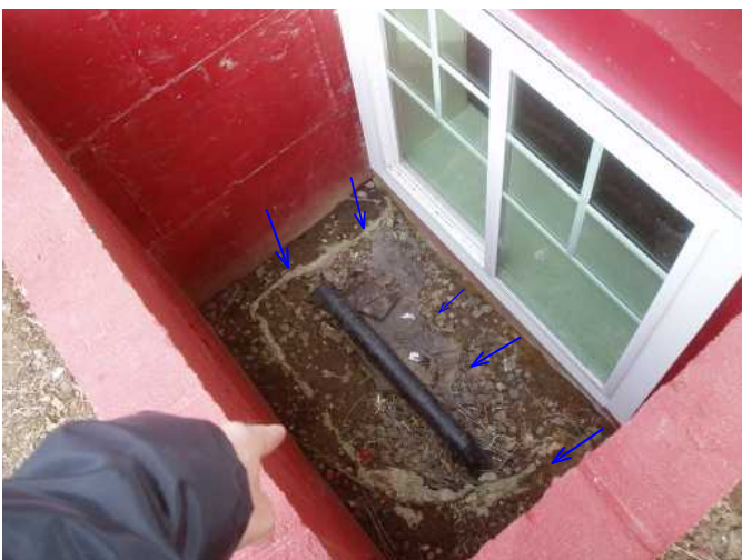
window well needs rock added for drainage...
