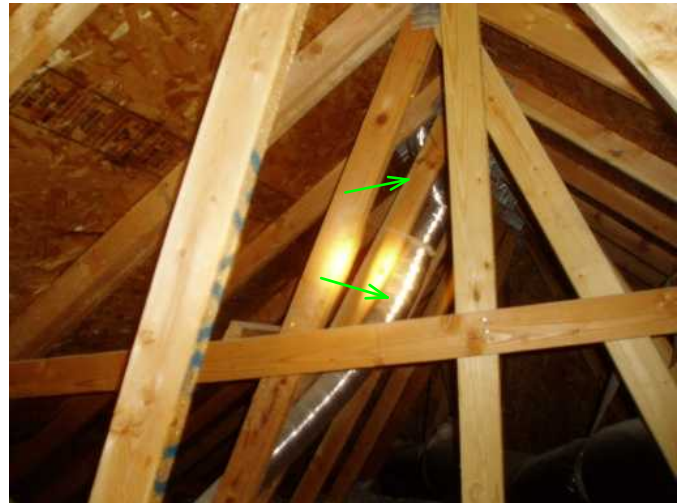
noting both 2 x 4 truss systems that are solid and sound...and bath vents to roof are operable..good..
