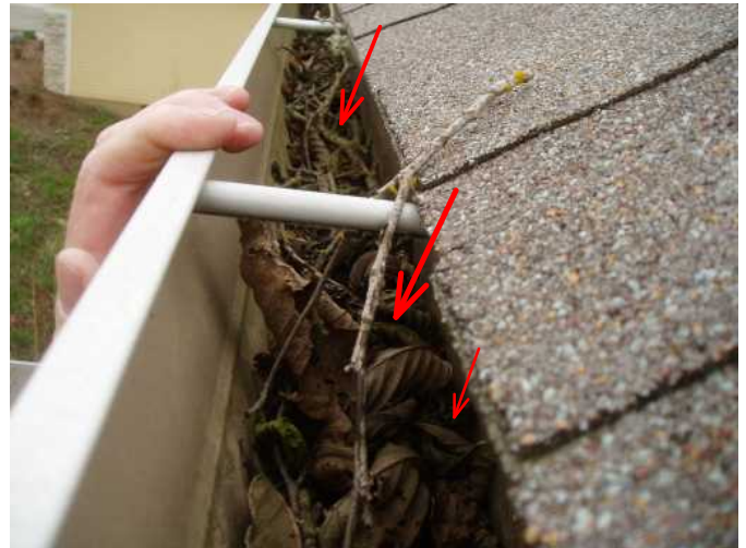
upper gutters around home are noted here with need to be cleaned...will overflow and cause erosion...clean...
