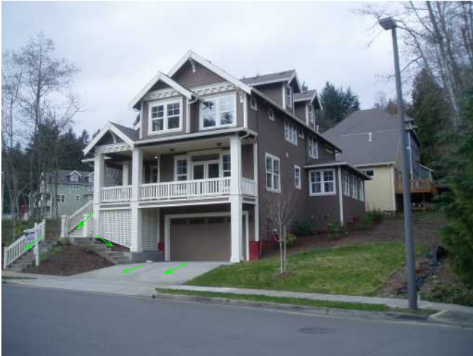
street view of home...driveway and stairs are sloped well for drainage...good..
