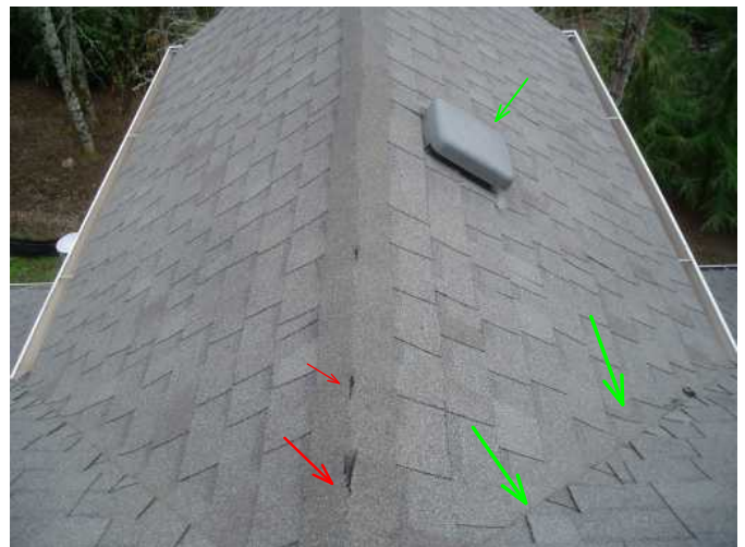
example noted here of gable dormer at back of east side is ventilated and has some damaged ridge shingles...valley fine..
