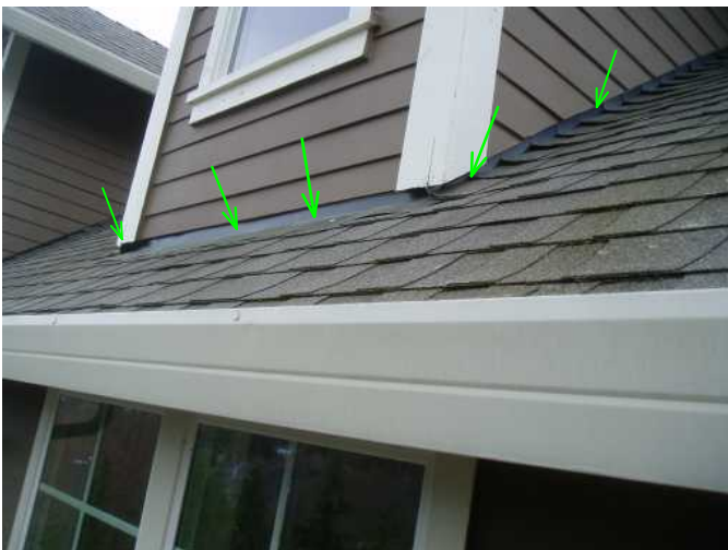
all dormers are decorative...but details are noted with excellent flashing jobs all around...very good...
