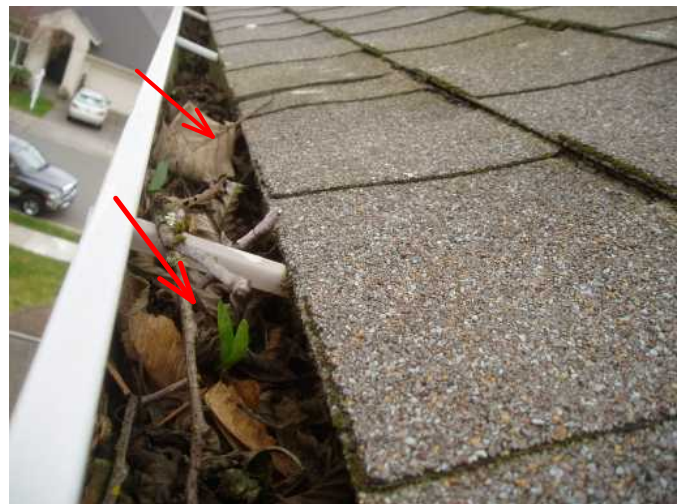
more full gutters...clean and try to clean often to avoid overflow and potential leaks into basement areas...
