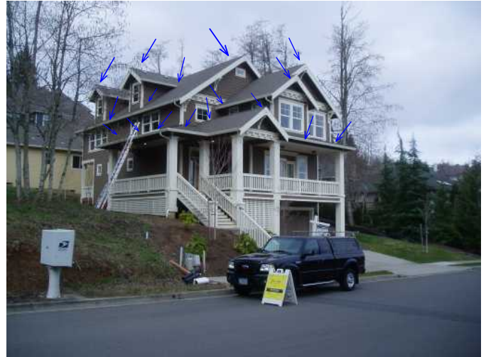
view of home noting multiple roof lines around home that means added cleaning and monitoring flashings...monitor often
