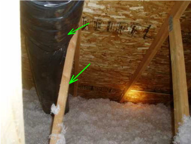
ducts are noted all insulated flex ducts...good...
