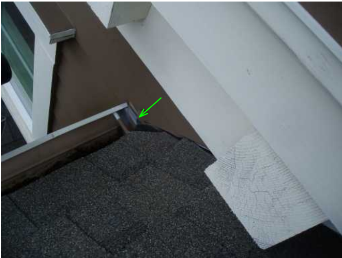
kickouts are noted at all needed areas as well...good...
