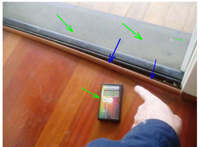
porch exit door threshold and weather stripping are fine..no high moisture noted..trim needs attached...
