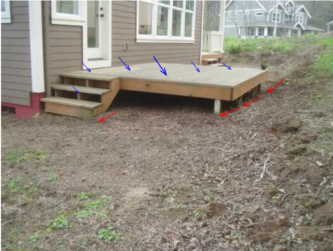
noting earth to wood contact at back deck lower grade to keep wood from rot..also clean and reseal decking...
