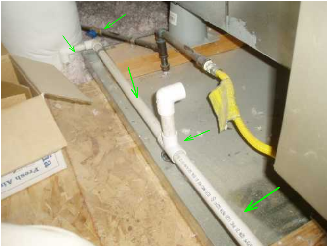
furnace is in drip pan and condensation drain and drip pan are plumbed to drain to lower and out area...good..
