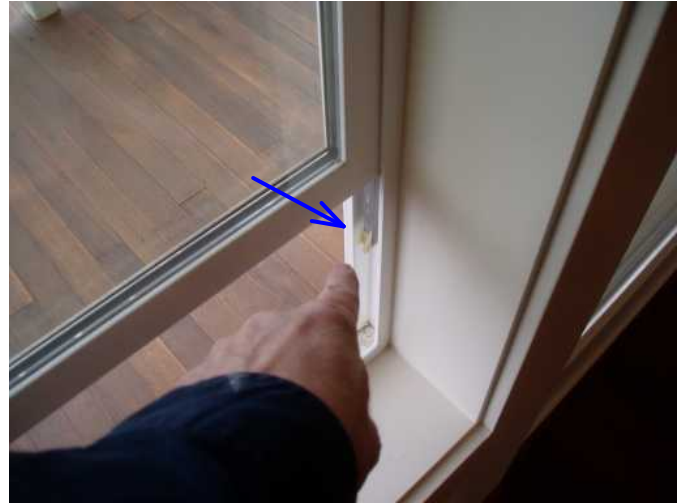
adjust tracks at living room window to flow easily....
