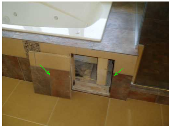
access to spa tub area is noted here...suggest all flooring around bath be caulked to avoid water wicking into MDF
