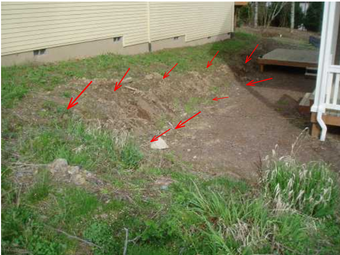
steep slope here needs retaining wall for erosion control...
