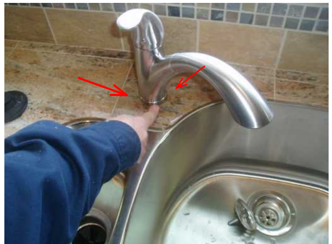
faucet at base here was leaking heavily and needs to be corrected..shut off at supply lines under sink....
