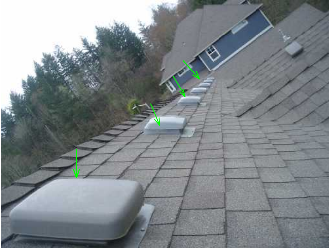
all vents at upper roof area are noted solid to roof..good..
