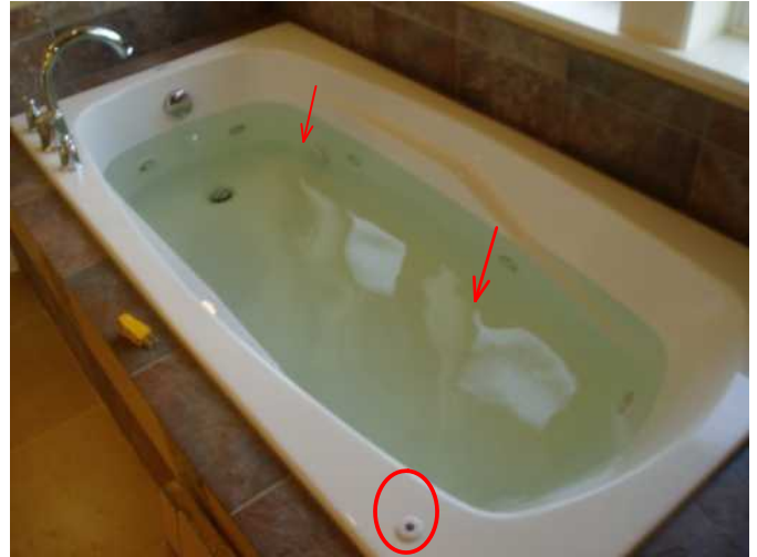
did not test pump..did not respond to switch...did not see how to plug in pump under spa tub enclosure..outlet energized
