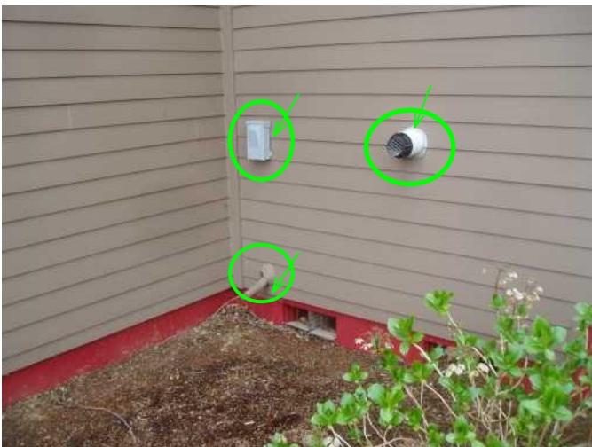
future home for air conditioner..add pad and a/c unit and rest is installed and ready...good..water heater flue is fine..
