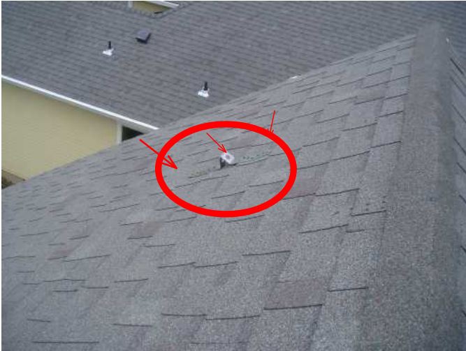
up on roof at back of home over west gable area....remove metal bracket noted here for roofer left behind....patch...
