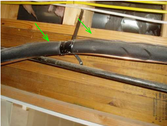
a/c lines noted installed and a/c ready...just add pad and unit at outdoors...and connect to furnace in attic area...
