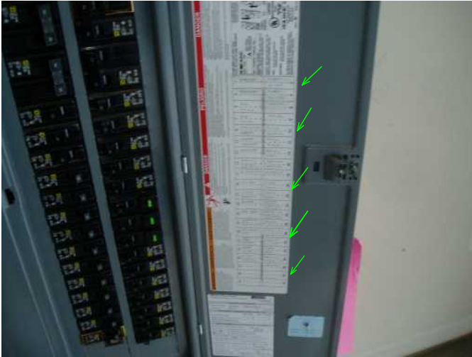
system is clearly marked and has additional breaker opening for future..
