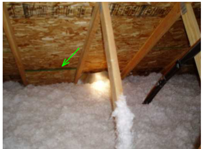
soffit baffles are noted spaced evenly and allow air to flow from lower to upper vents...good..
