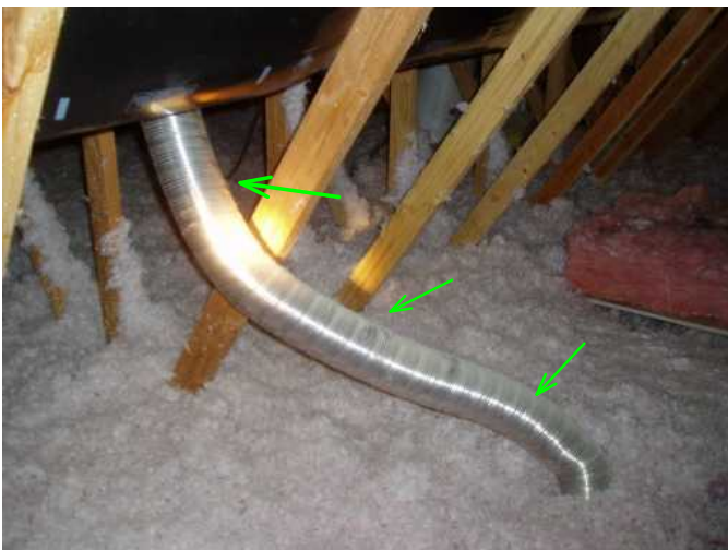
all bath and laundry vents to roof are installed solid and hung to stay...good..
