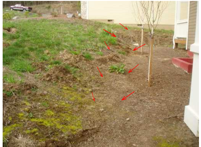
noted at side as well....add retaining wall to reduce or emove all potention erosion...
