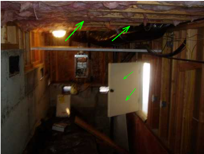
overall view of crawl space is noted here with under floor insulation found installed well...good..
