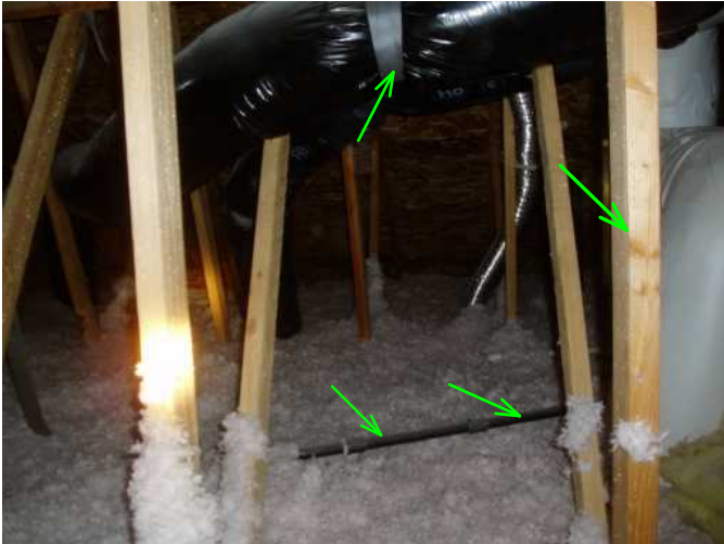
gas line to furnace is solid and dcuts are all insulated...good..
