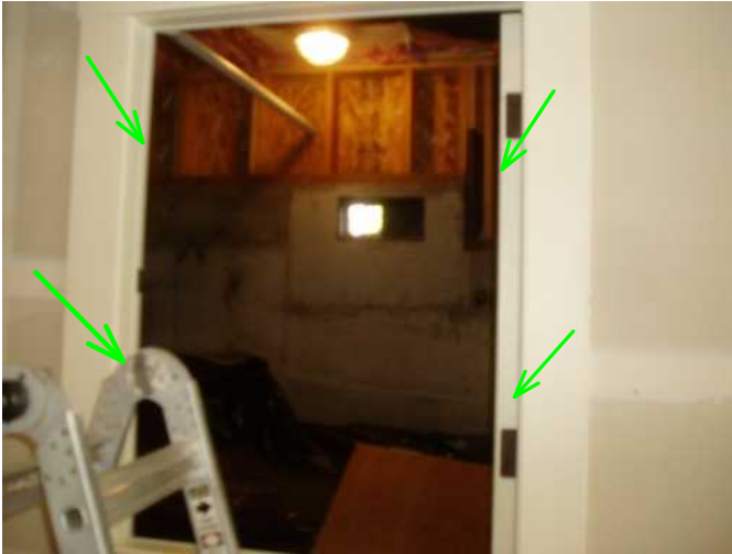
access door to crawl space is noted here in garage and is weathe stripped well...good..
