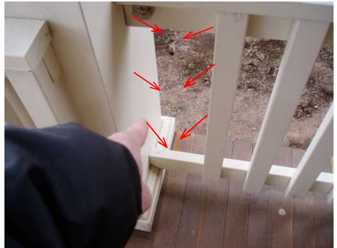
noted several areas that need spindles, max of 4 inches allowed between spindles...coorect where needed...both porches
