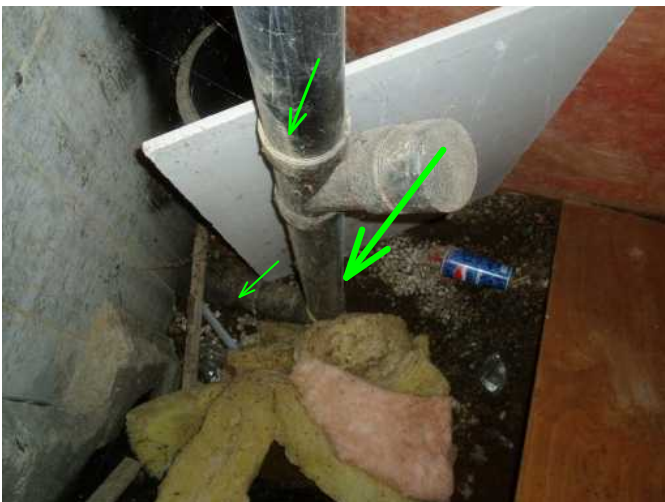
main sewer exit line is noted here and is accessible for clean out if needed...
