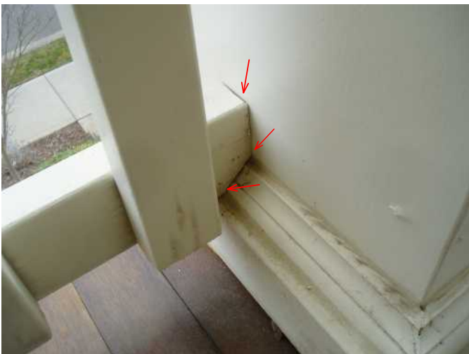
any gaps found at intersections will allow water to stand and rot wood...caulk all open gaps...cracks to extend life
