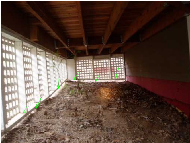
under front porch noting beams are in hangers and attached well to structure...good...no earth to wood contact here...
