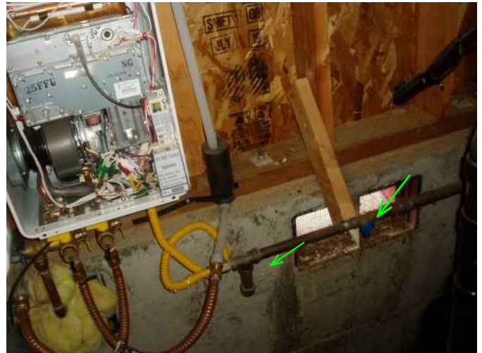
drip leg is found and main shut off was found off and was left off when found in state of condition here....
