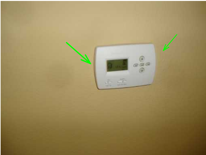
programable thermostat is noted in center of home...and appears to respond to requests...furnace not operable..
