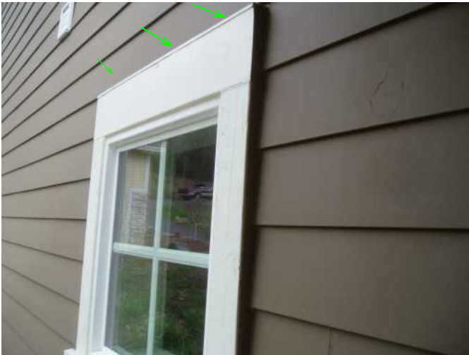
z flashed at all windows and trim around home at upper areas needed...good..
