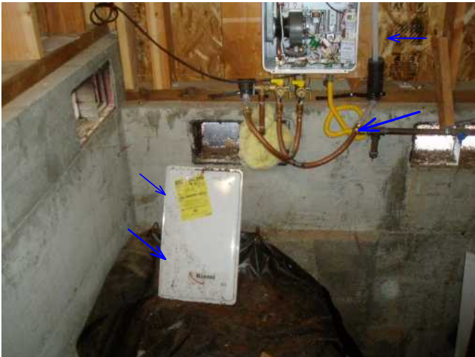
cover found on crawl floor and no screws found to attach...some PEX pipes need insulated...
