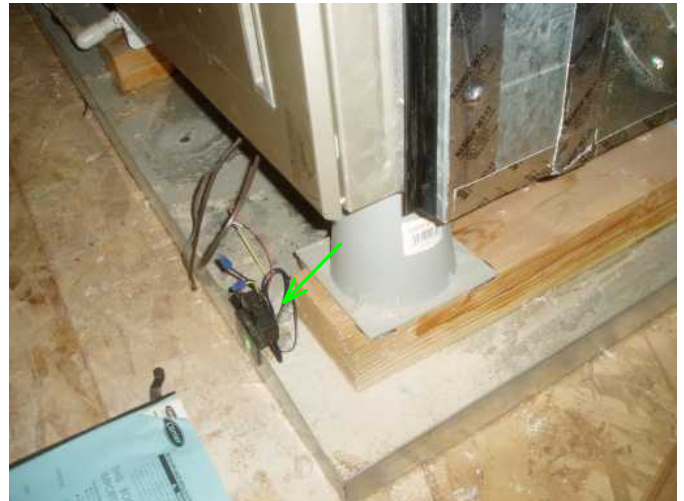
overflow shut off is noted in drip pan...if detected to be full of water, will shut off furnace/ a/c units...
