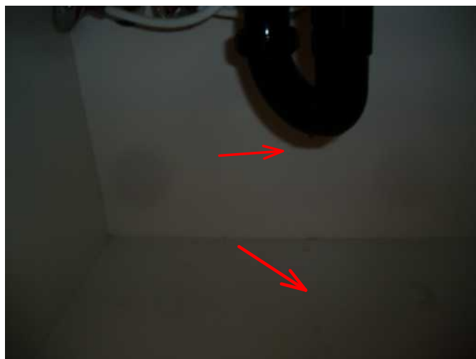
leak detected at left trap area...correct...
