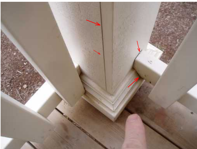
caulk at all open cracks at trim at porches and wood will last many years...will fail in a few years if not...
