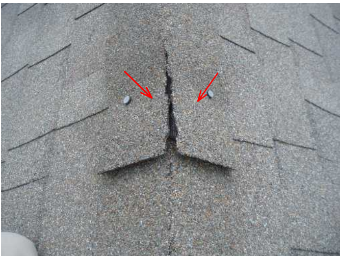
random ridge shingles noted split at many areas of several peaks...replace all damaged like this...example of many...
