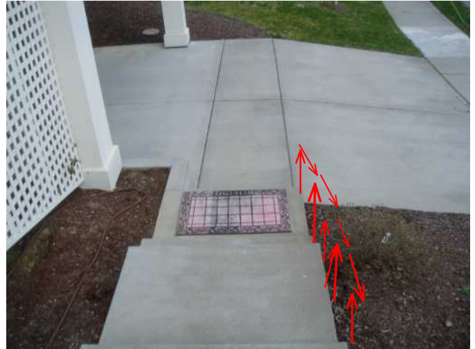
add handrails to second set of steps to avoid trip and fall concerns in winter freeze times...like front stairs..
