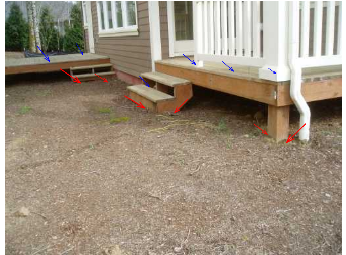
keep all earth to wood contact clear..and clean and seal both decks at back of home...
