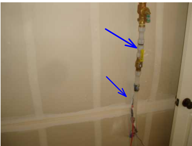
main water entry and shut off noted here, suggest insulation added to protect from freeze in winter....
