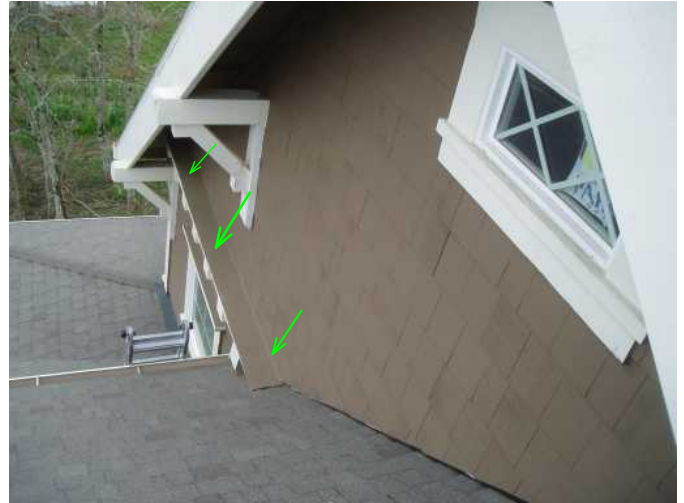
over windows are flashed very well..flashings over deep wood trims are custom made....and is sign of well detail home
