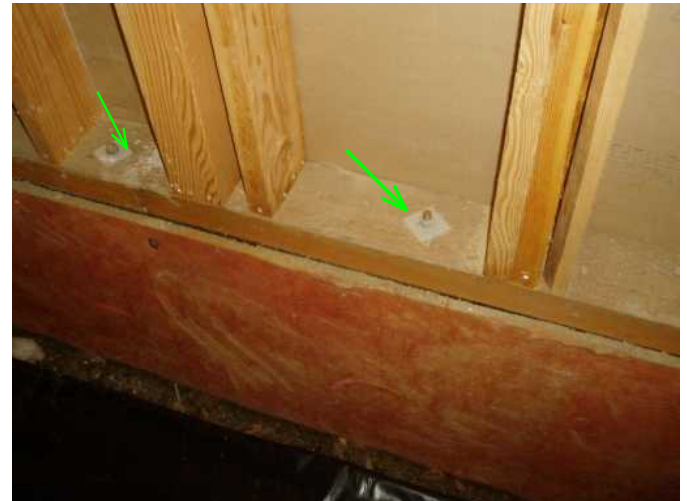
earth quake protection found at foundation and mud sills...good..
