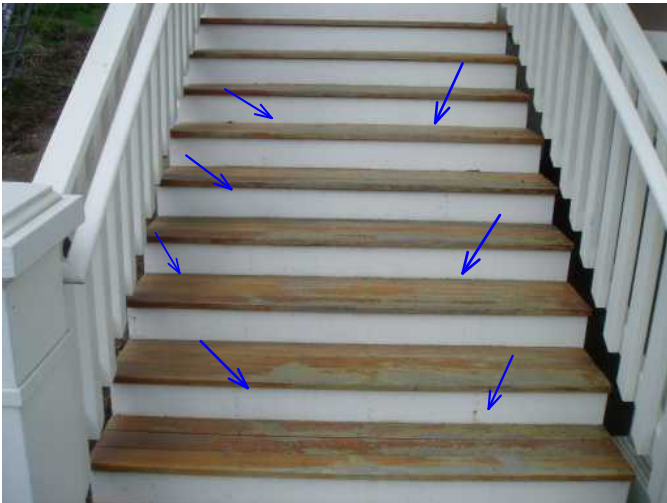
stairs have finish issues, needs to be sealed with weather resistant finish to extend useful life of wood...
