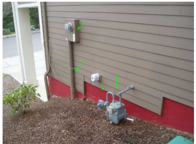
main electric entry is noted fine...gas meter is solid to home and main shut off at meter...fine...
