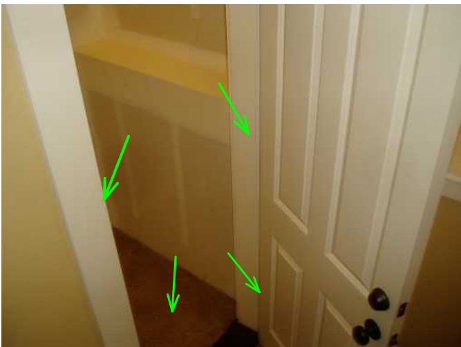
left door at landing to garage is weather stripped and threshold is noted solid and sound...good..
