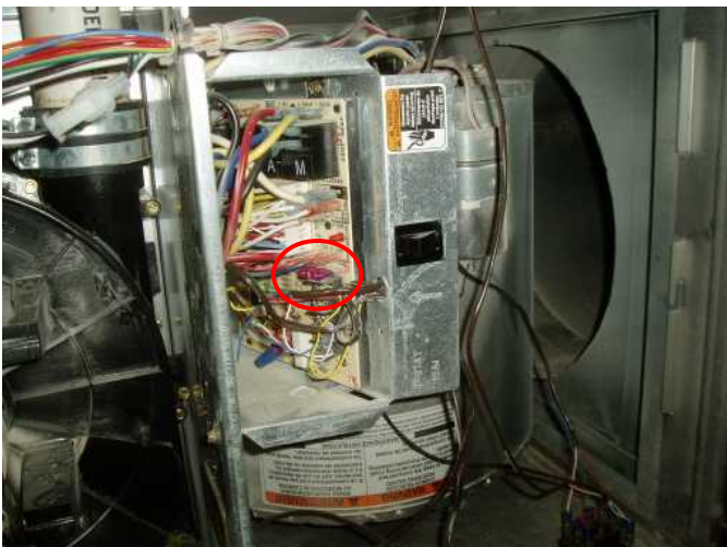
this little fuse is the culprit that appears to have failed and there is a second one on furnace as well..repair unit
