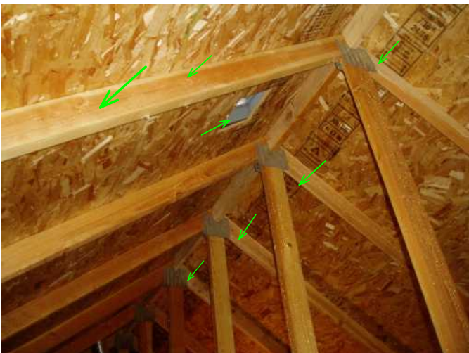
looking up at peak of main attic and noting the roof vents are without staining...good...trusses are evenly spaced...
