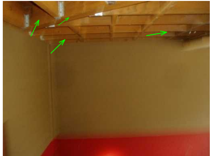
see hangers...very solid and installed well...good..under front porch...
