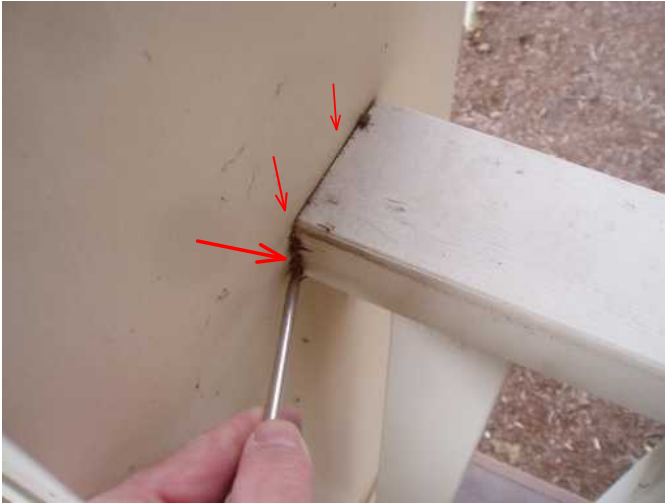
see how wood is dark and needs caulk and paint to extend life of wood by many years...
