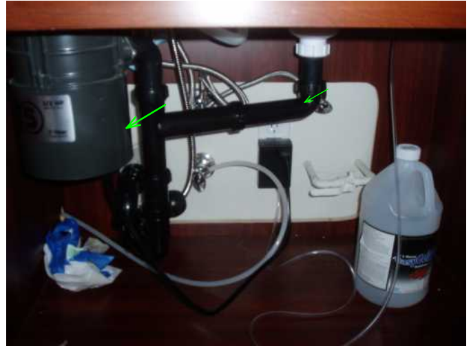
garbage disposal is noted operable..has pneumatic switch and is noted better quality install...good..no drips noted traps...
