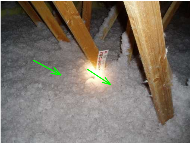
attic is installed with blown in insulation...good....deep and acceptable..will reduce energy bills...good..
