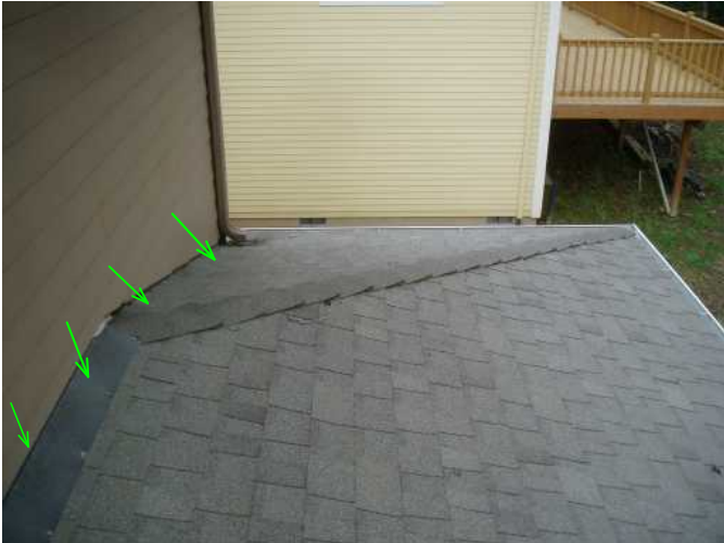
on roof over sun room ...flashed well...good..
