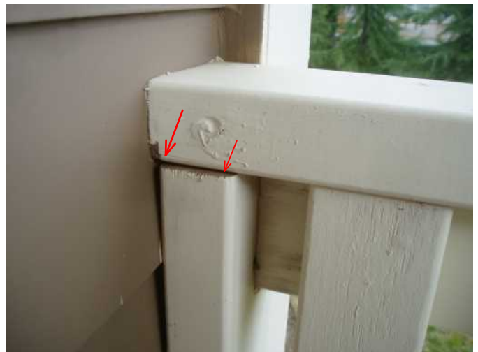
all wood is cut and installed and then painted...see raw wood here? Will wick water and rot...caulk and paint...
