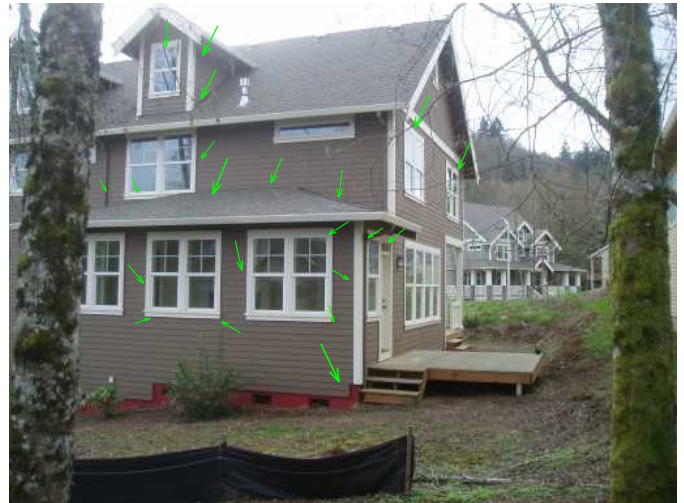
south side of home noting the roof lines and z flashings are installed well all around home...good..
