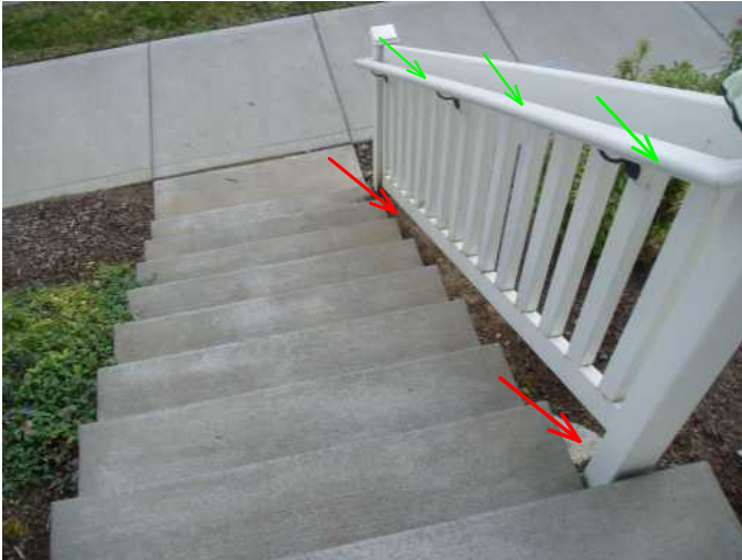
handrail at main stairs to home are solid and sound...but need earth pulled back at posts...
