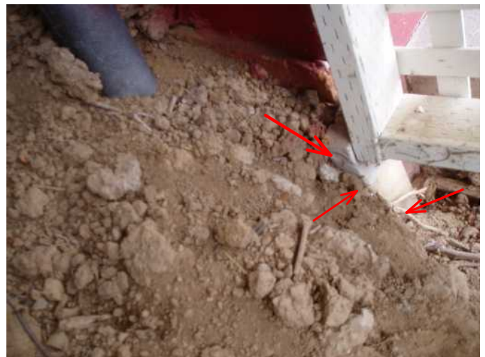
remove this 2 x 4 at garage area wall to skirting..is buried in earth...will draw termites and rot...remove asap...
