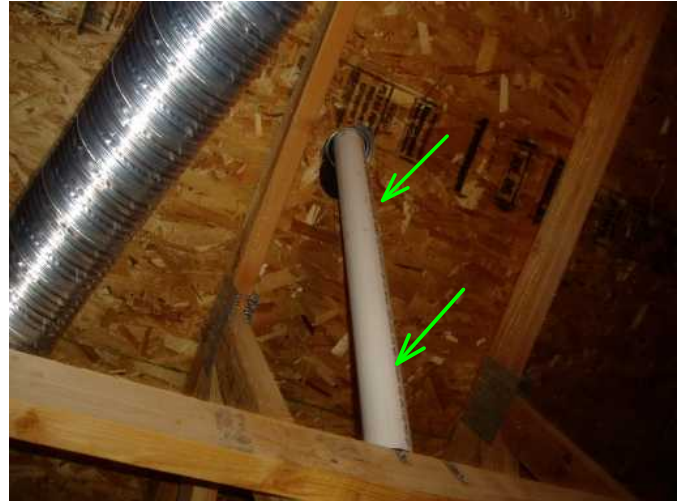
furnace flue to roof is noted here and is stain free.....good..
