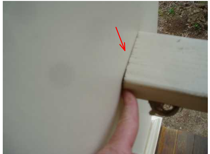
both front and back porch railings have open gaps at random that will need caulked to extend useful life of wood...
