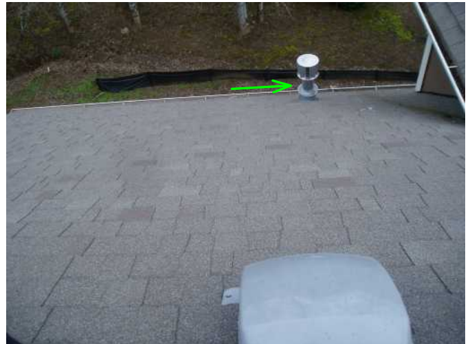
fireplace flue noted here is flashed well at south side of home upper roof...good..
