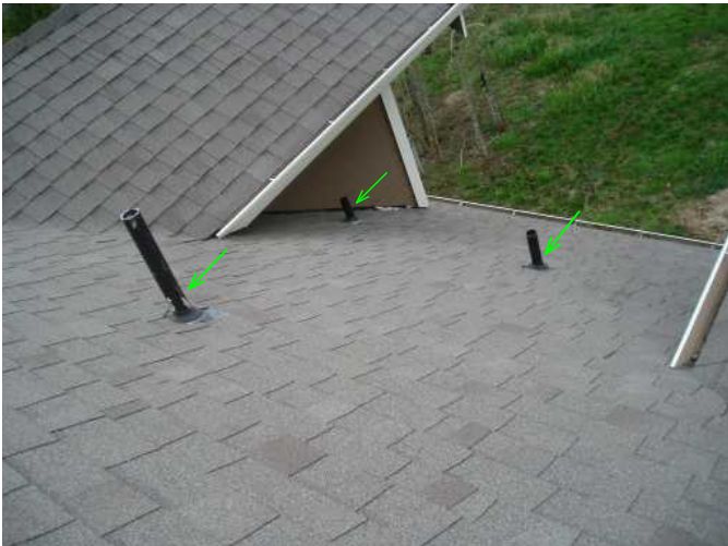
sewer vents are flashed well and step flashings are noted installed well at dormers...good..
