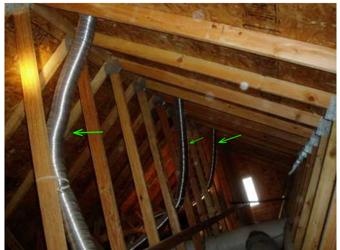
here is view of all three vent tubes to roof vents...srapped solid and attached well..good...
