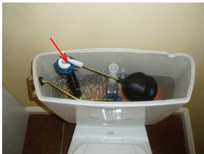
main toilet feed line is blocked and needs repair...did not fill tank as needed....correct....
