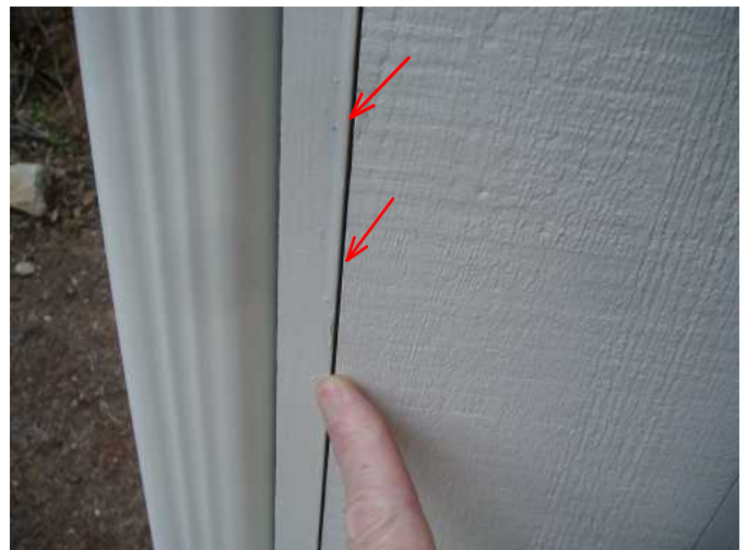
these seemingly innocent little cracks are suseptable to rot...correct with caulk...and then paint
