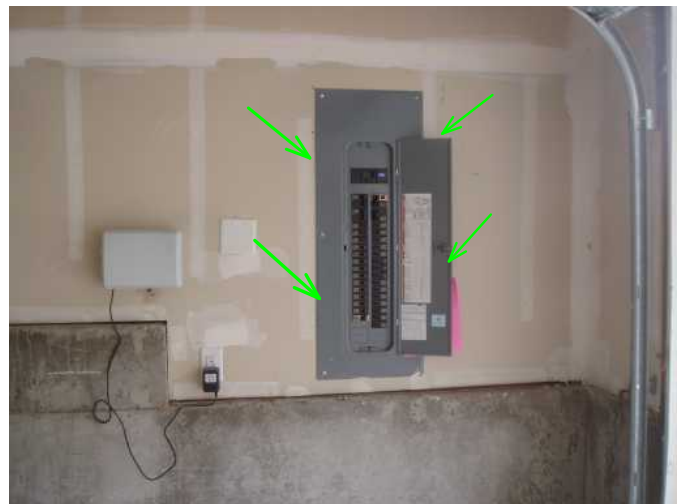
200 amp system is found in front of garage and is noted installed well, all clean and professional work found...good..
