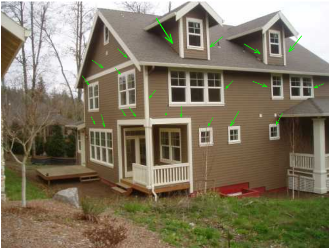
back view of home...noting all windows and trim are z flashed and envelope enclosure are installed well...
