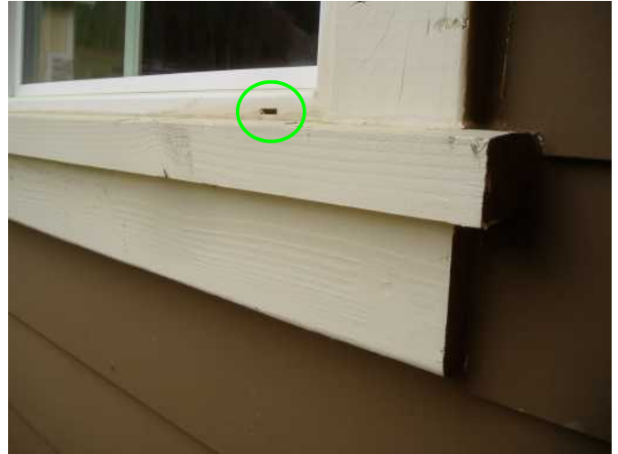
all windows are assessed to see that weep holes are in bottom of windows and not on top or sides...all good
