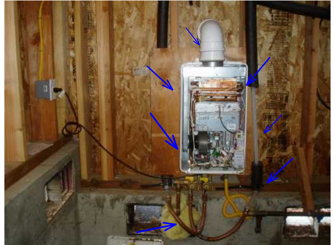
water heater is found not user ready...cover plate is off and gas is shut off and needs serviced to make user ready...
