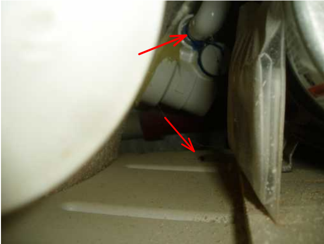
this is master bath spa tub and noted leaks at fittings under tub in enclosed area...correct....
