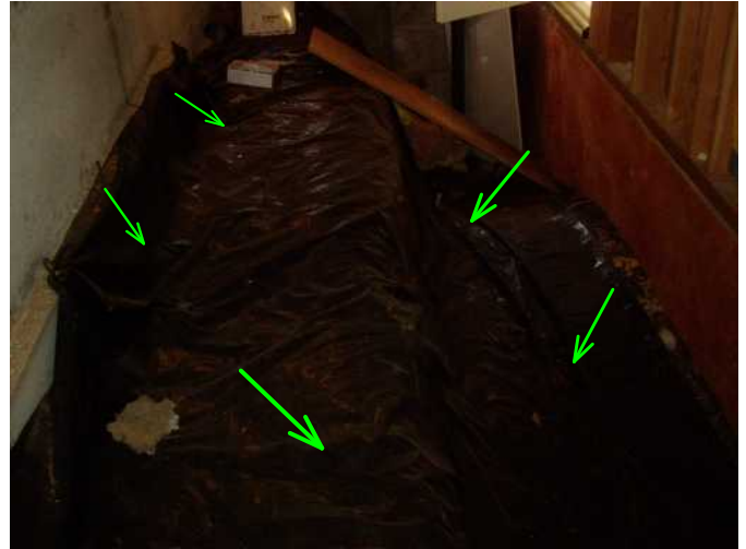
vapor barrier found all along floor of crawl space.....good..
