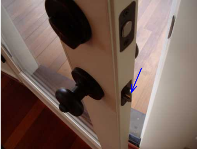
door handle latch is noted here to not latch...correct...
