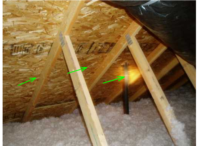
OSB sheathing is noted in attic for decking under roof and sheathing at sides...plywood is at exterior areas of soffits
