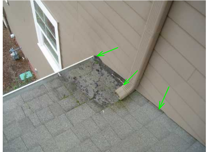
flashed well and kickout is designed to control flow from downspout and is working well...good...
