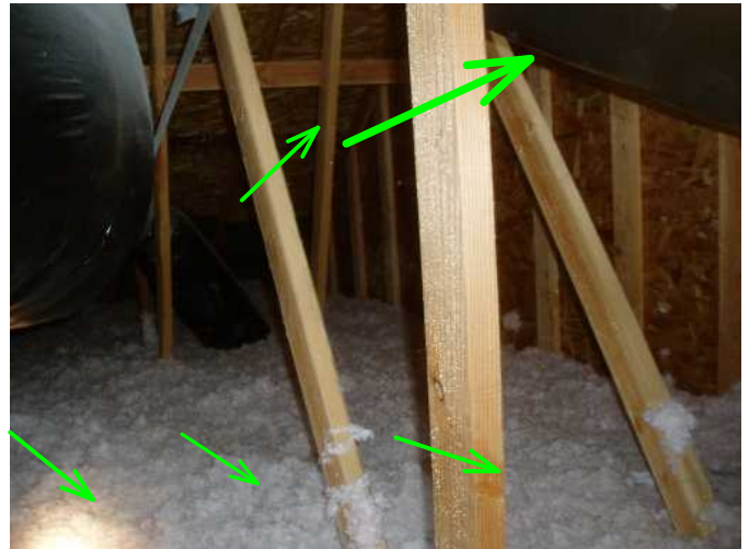
up in attic facing forward and noting solid truss system and insulation is installed even and well...good...
