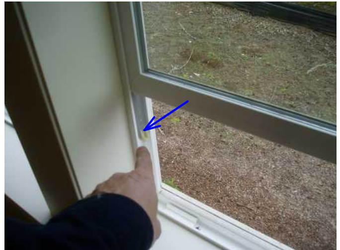
window track noted here at sun room window needs adjusted to flow easily...
