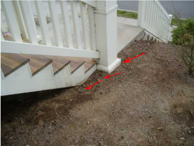
pull back earth and watch the wood last for years...
