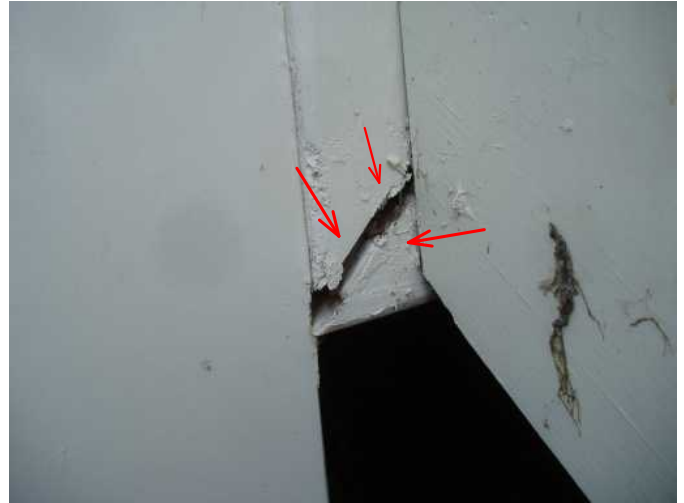
all open gaps like this one will promote rot quickly...a few years will be rotted...caulk all gaps...
