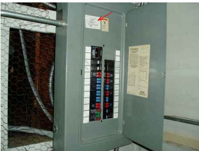
electric panel is 1985 installed and signed off...good...
