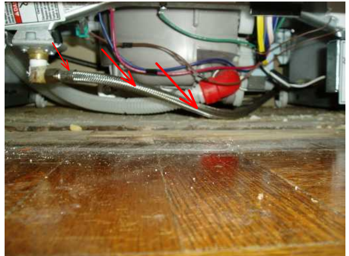
under dishwasher is dry..and metal mesh hoses are my favorite...
