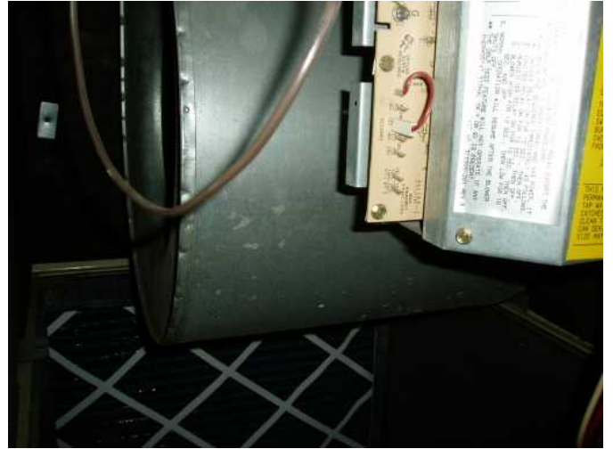
furnace fan and filter ....
