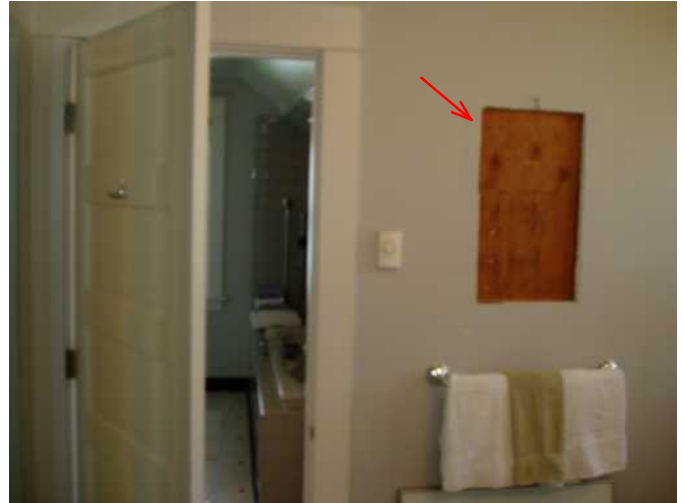
wall needs patch or cabinatt installed/had picture over it...
