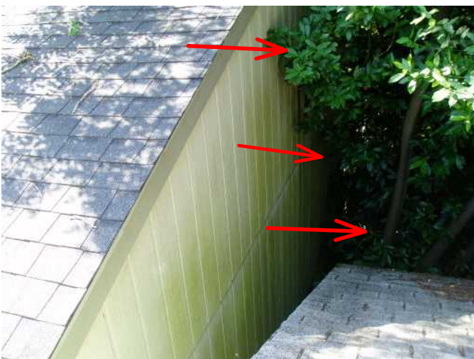
backside of garage will need trimmed back for vegetation...
