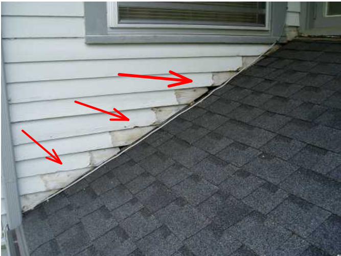
here is great new flash job/will need a bit of paint..see old step flashing marks?
