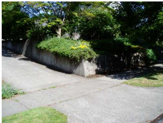
concrete retaining wall front lower area of home...good
