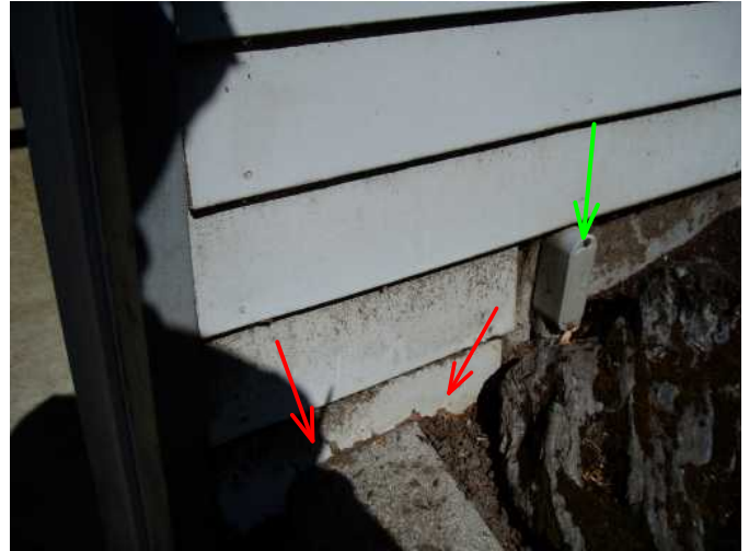
small arewa of siding show rot...at dirt level...replace this one piece...easy fix...electrical entry done well...
