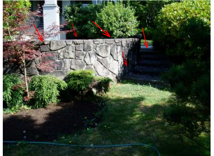
stairs and wall are solid...
