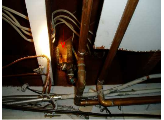
hose bib shutoff to outdoors above laundry..good...all copper pipes..very good...
