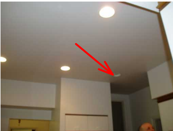
one kitchen light is not operable..please make operable..is probably bulb...but lets be sure...
