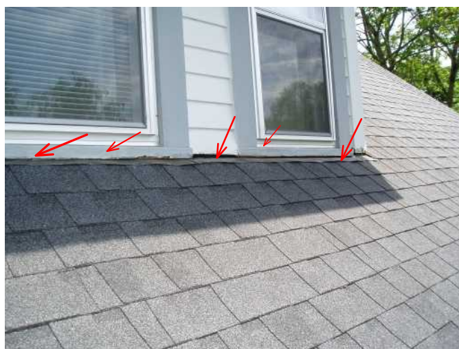
great flashing..will need trim paint...
