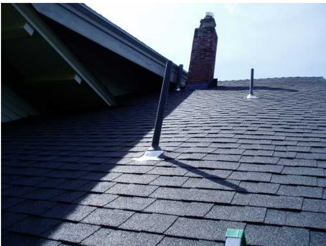
another better view of flashings...good...
