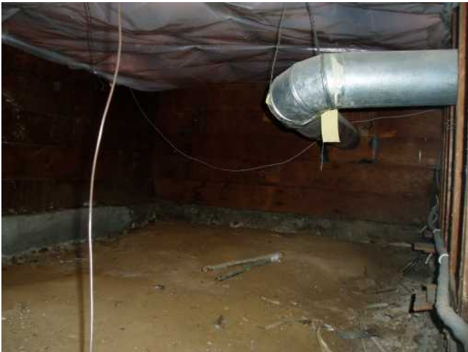
second view of same crawl space...
