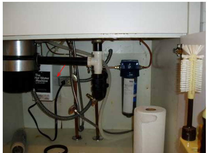
under sink no drips here...hot water dispenser should be monitored/known for leaks often(high maintenance)
