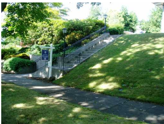
stairs and handrails are great...
