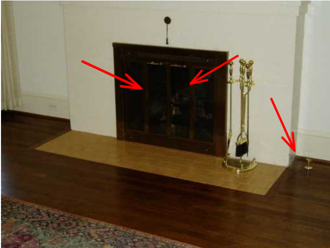
fireplace has gas log inside..good..control by key use lighter to ignite...confirm glass is tempered or ceramic...
