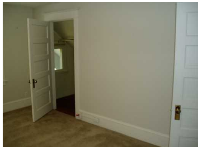
bed 2 doors work fine..only one grounded outlet here...
