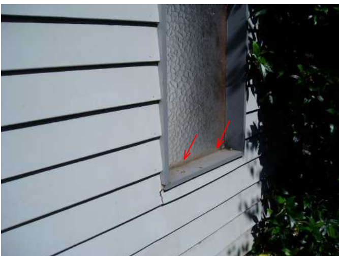
garage window appears to need new caulk around base of window...
