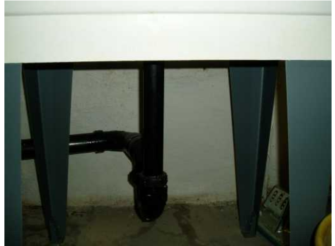
under laundry tub is drip free....
