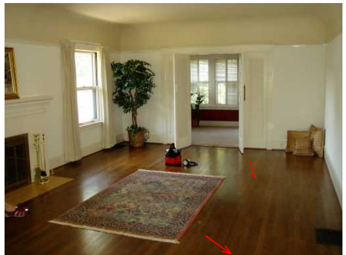
living room/wall outlets are mixed..grounded and ungrounded.floor outlets were not operable...
