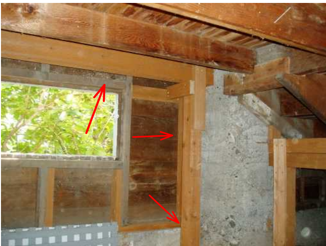
new support at front of porch/done by the book...great...
