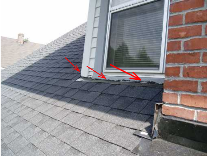
great new flashing..will need trim paint...
