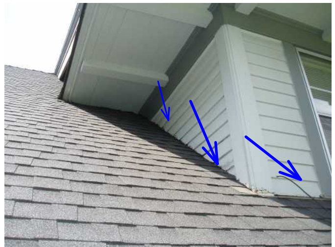
trim paint around dormer siding...
