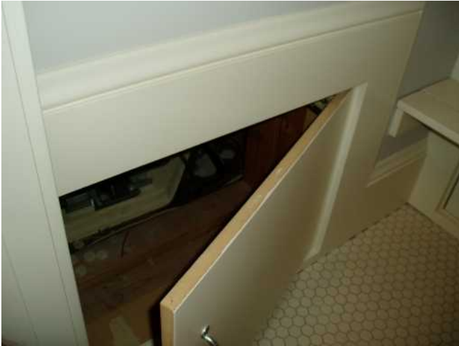
access to pump...bath...
