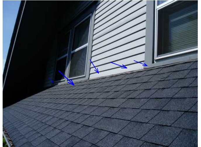
great flashing front of home...trim aint looks good here...
