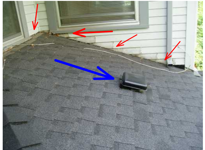
great flashing/needs paint...1st floor bath vent....good...
