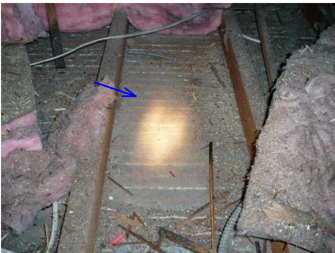
this shows that all walls and ceilings are lath and plaster
