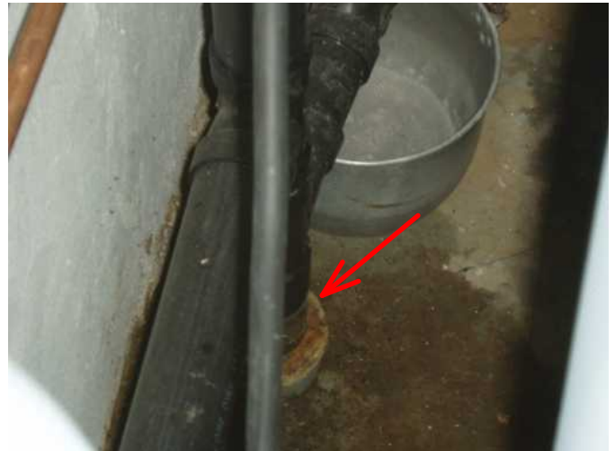
exit pipe to sewer exit is sound....
