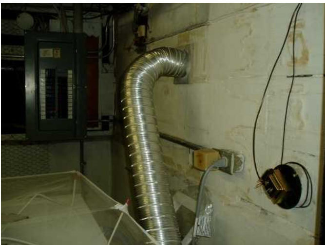
dryer exit vent to outdoors is good...
