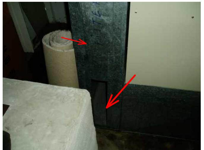
filter access on outside of furnace...
