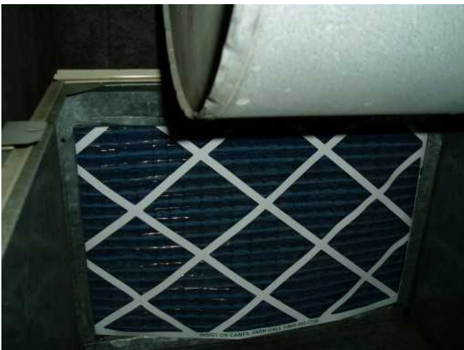
second view of filter/fan box...
