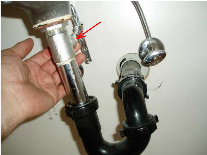
drip noted here at stop connector...small now/ will get worse...please fix...
