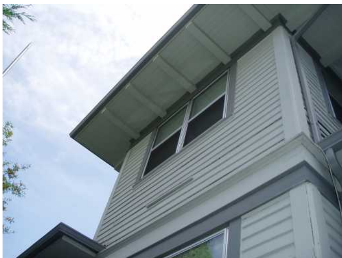
siding and trim are overall maintained well...
