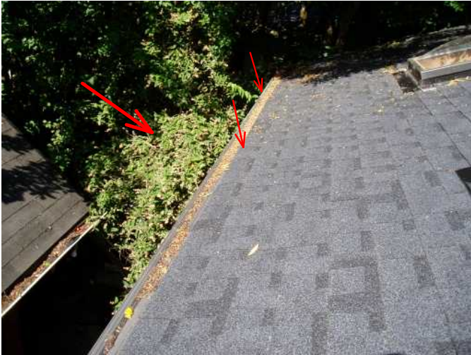
gutter cover is engulfed in debris/trim shrubs touching side wall of garage...
