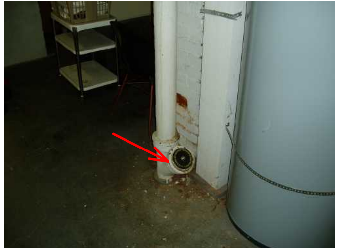
sewer cleanout access basement by water heater...good..
