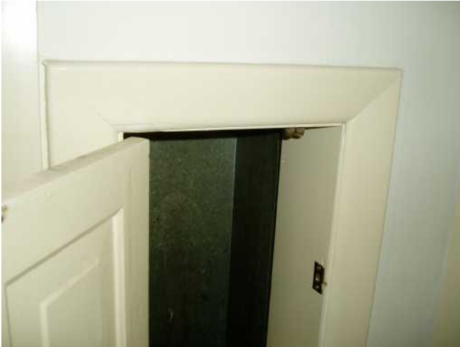
laundry chute in hallway behind kitchen door...
