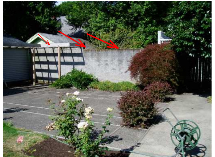
parapet wall is solid and secure...
