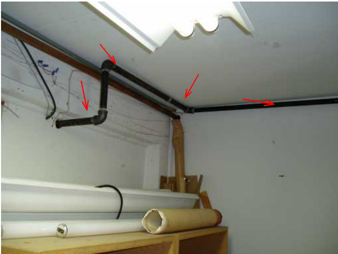
gas pipe to fireplace for gas logs....from furnace and water heater access...
