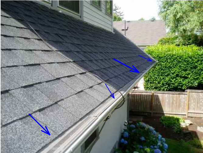
gutter covers are good this side of home...
