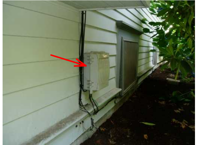
cable box and entry to home under dining room...fine...
