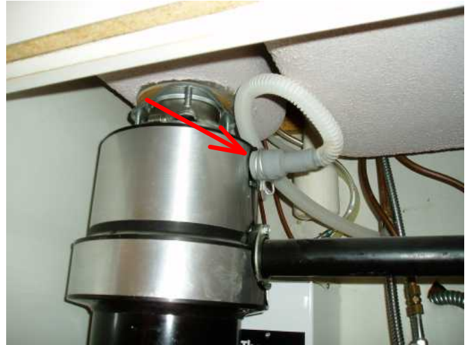
air gap for dishwasher is good...garbage disposer not responsive....
