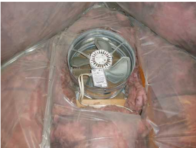
thermal switched attic fan woks great....
