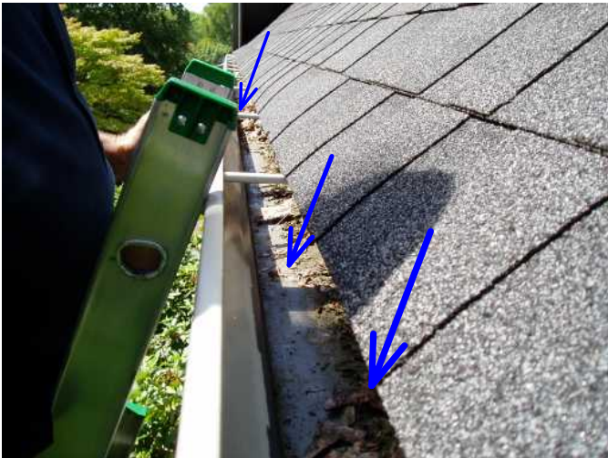
front section of gutters missing cover...odd...
