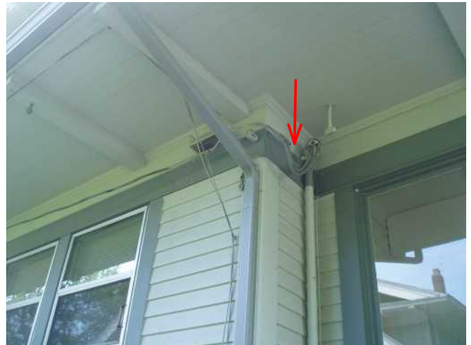
electric drip loop good....
