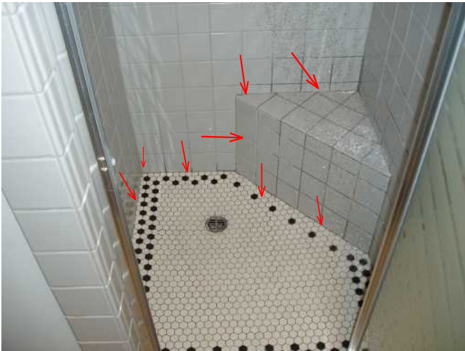
these areas are the most prime for cracks and leaks...
