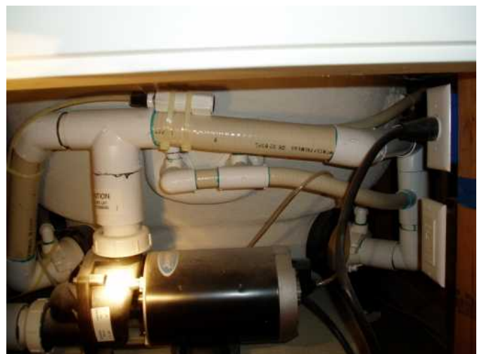
plumbing for bath appears leak free....
