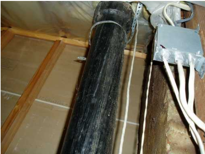
main sewer vent is installed fine...
