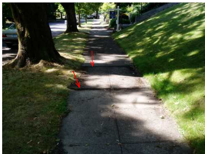
sidewalk..street level...has two noted uneven possible trip factors...suggest leveling...
