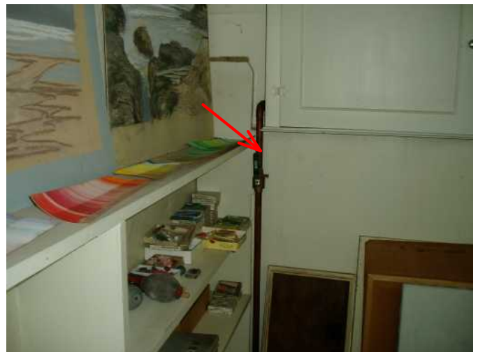
hose bib shutoff to outdoors ...
