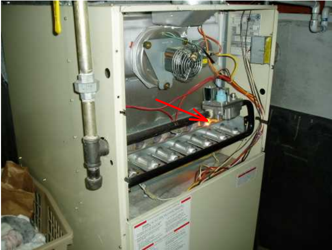
furnace in basement...showing electronic ignition..not standing pilpt...good...
