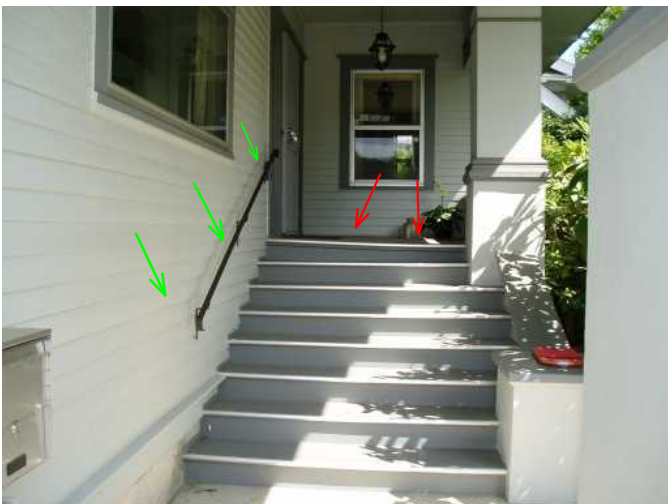
front porch has good slope/ stairs are solid and sound...handrail is solid as well
