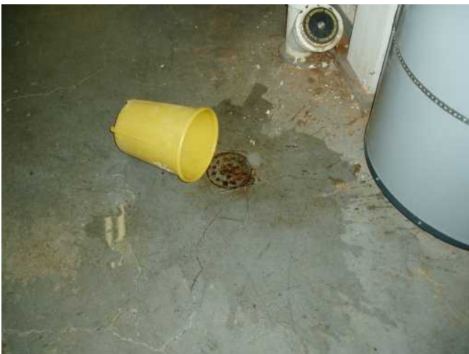
basement drain checked and operable...
