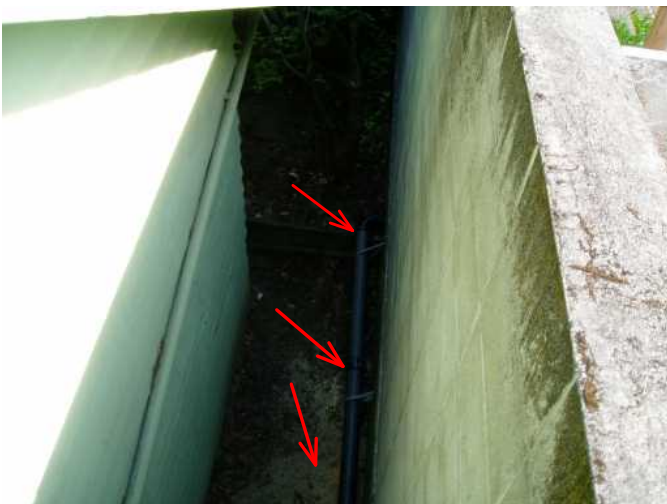
this is surface drain exit from patio..very nice...behind parapet wall....connects with downspout/garage...
