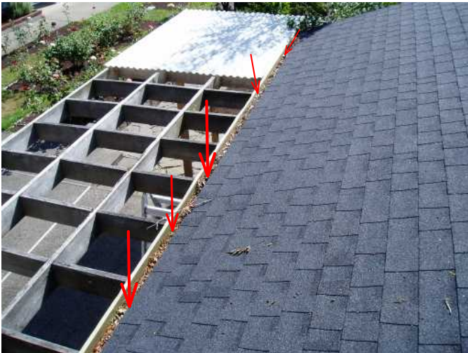
no gutter cover here and very full of debris..needs to be cleaned...
