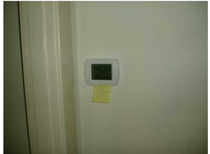
first floor thermostat control is programmable...ask for owners manual...
