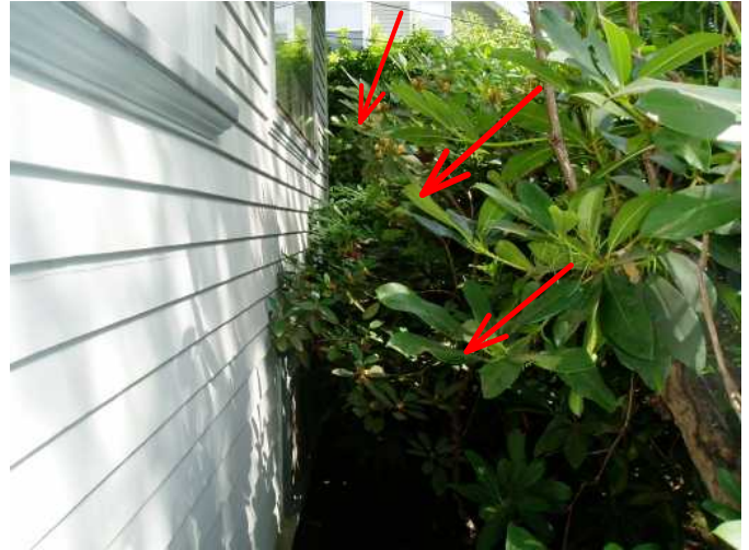
front of home has need for trimming back vegetation to keep 12-18 inches from home...
