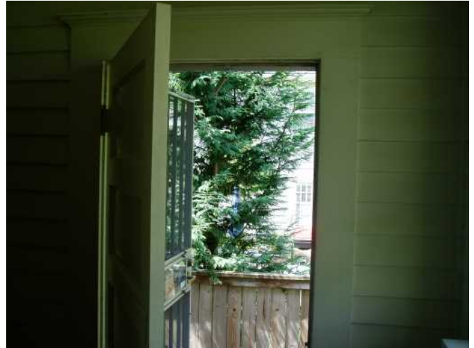
rear exit door is good and solid..weather stripping is good...
