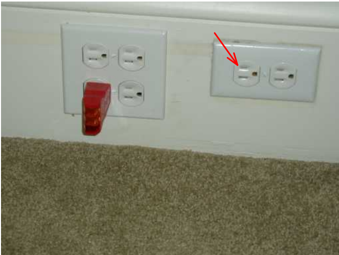
master bed outlets on left are grounded/on right tare not...go figure...
