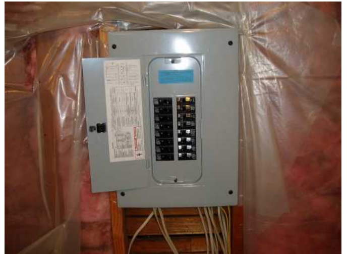
attic sub panel..installed in 97/signed off by inspector...
