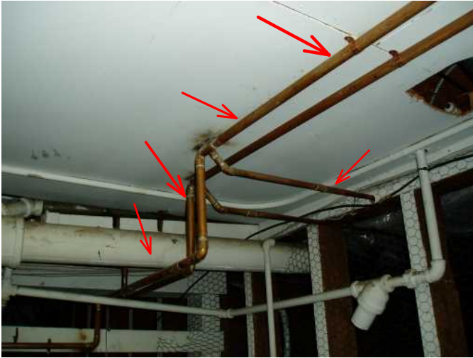
more copper pipes...
