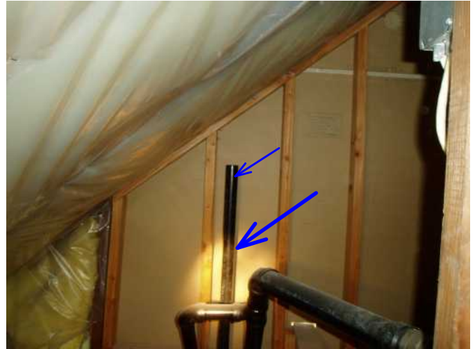
this is sewer vent pie in question..should be capped...
