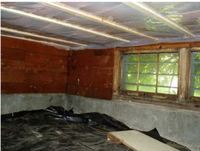
crawl space under dining room is awesome...insulated and moisture barrier is installed great....
