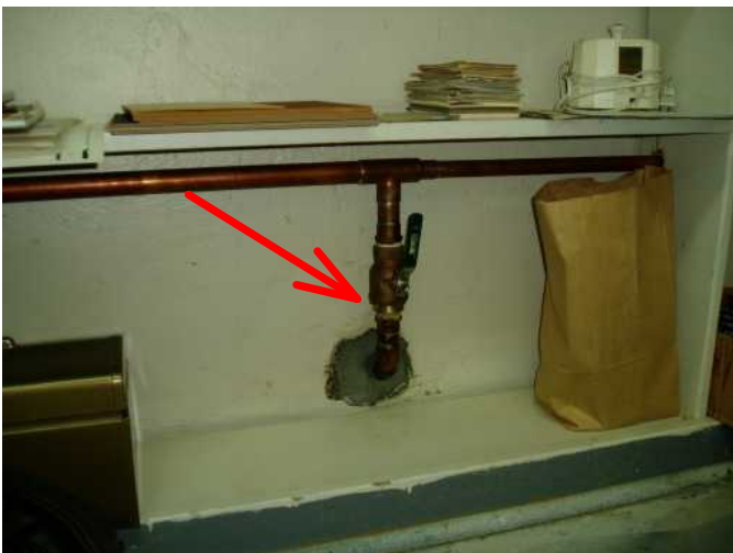
main water entry and shutoff in front of home basement under living room...
