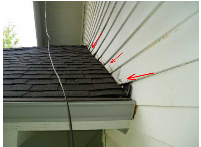
same here..great new flash..needs pant at old flashing areas...
