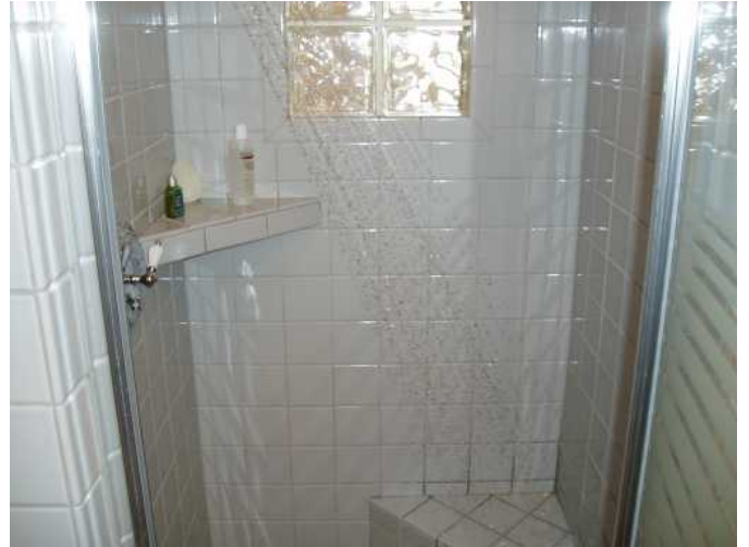
main shower works fine..no leaks apparent at this time...monitor grouting...around base mostly...
