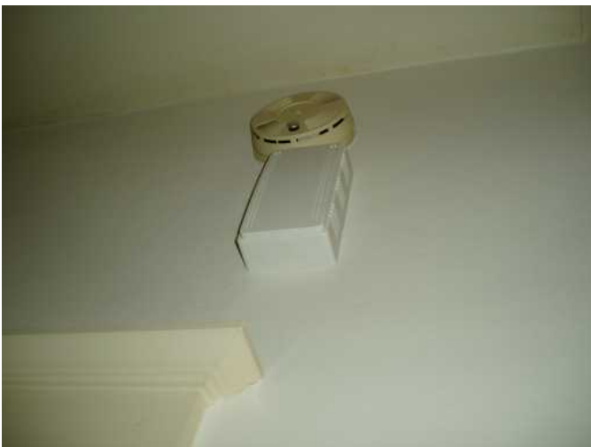
door bell and smoke detector...
