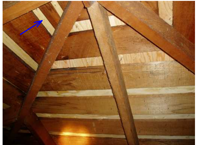
this is in rear attic area showing old plank and new plywood roof sheathing..very good...dry...
