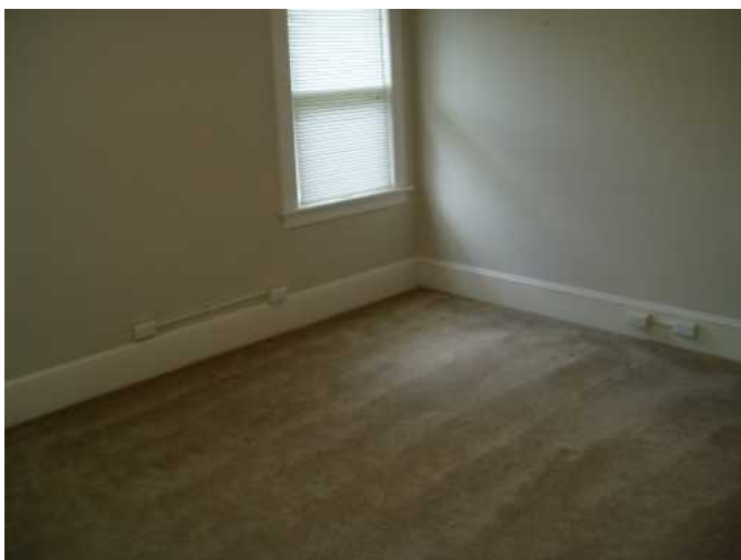
outlets in thsi room are all not grounded...windows work fine...
