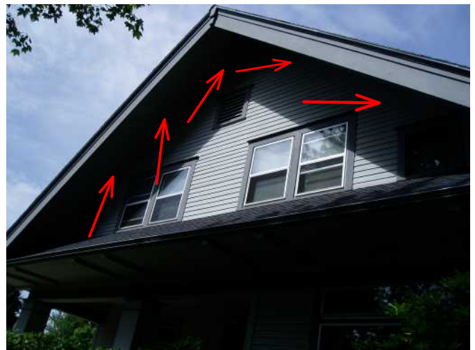
all trim under soffits around home is well maintained...
