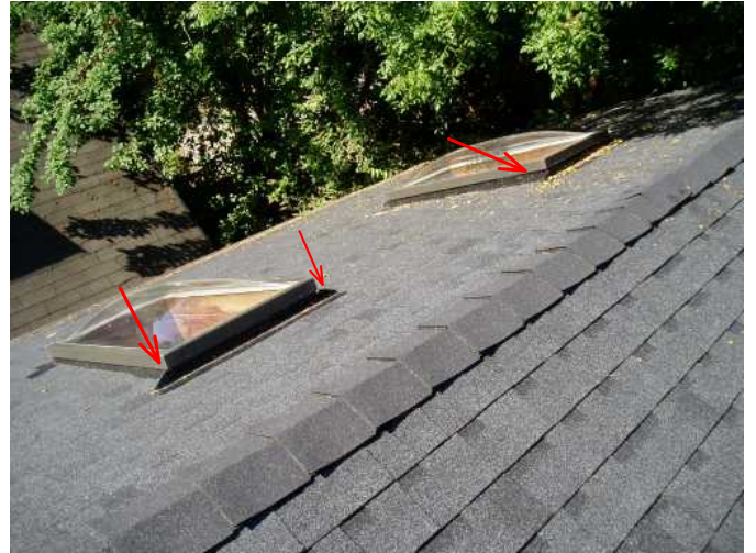
new roof and new skylight flashings appear to be installed very well...
