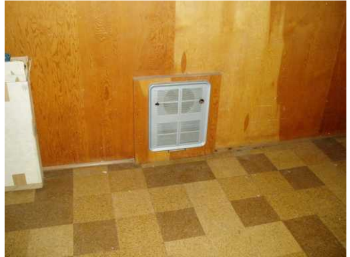
wall heater in basement room works fine...zonal...
