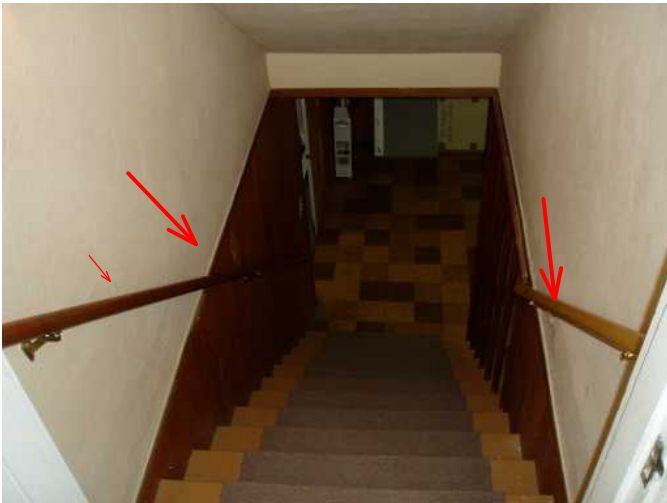
handrails to basement are solid and sound....
