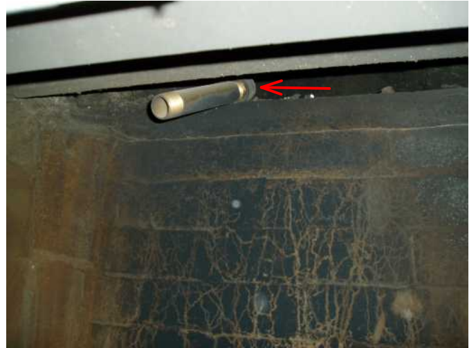
replace pipe with attached clip...easy fix...damper fireplace...
