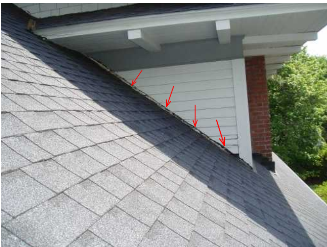
great flashing...trim paint needed...
