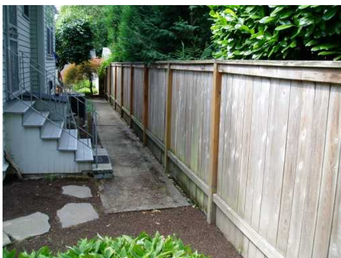
rear fence appears to be newer...
