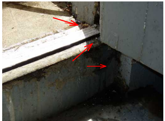
area noted with stains...
