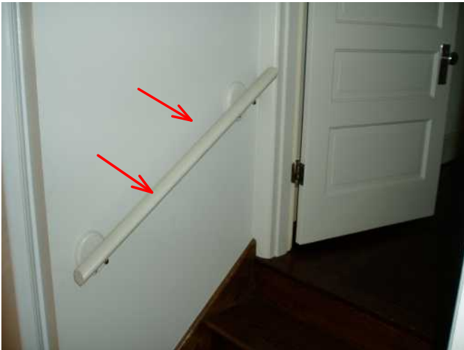
handrail to kitchen is solid and sound...
