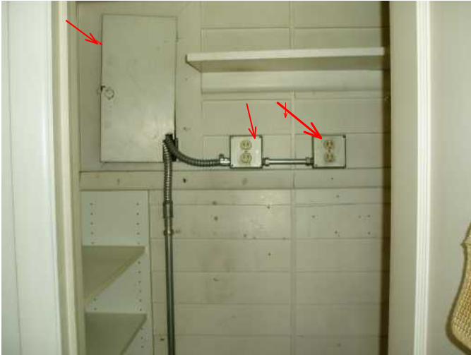
old panel...outlets are grounded....
