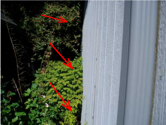
left side of garage needs trim back of vegetation to keep siding from moisture intrusion...
