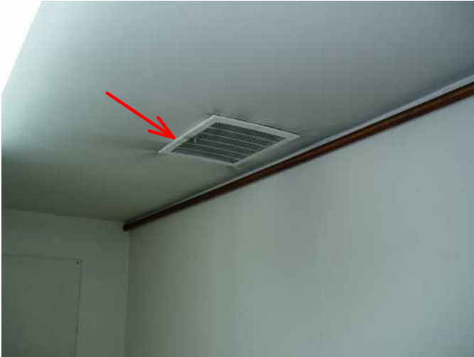
work room in basement has furnace/a.c access....good...
