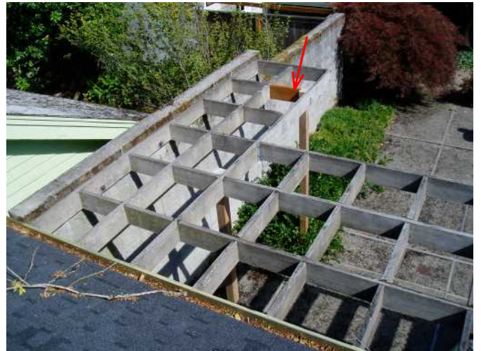
decorative wood needs to be power washed and sealed to extend life..see replaced section?
