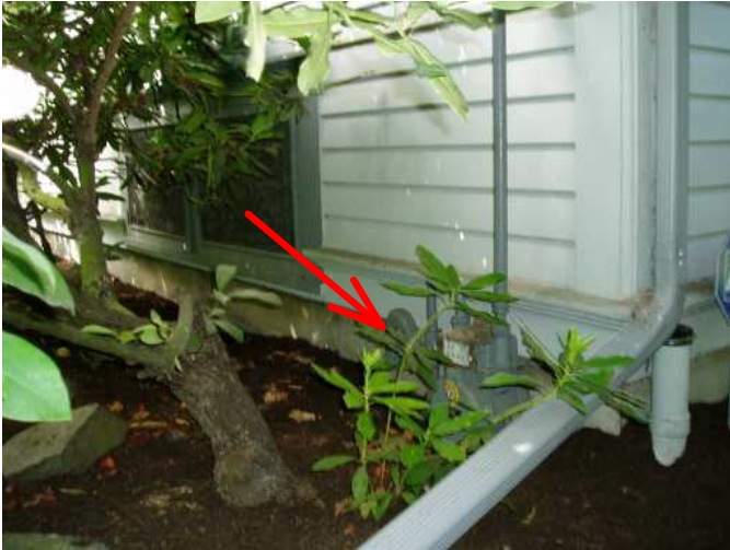
gas entry and main gas shutoff front off home...
