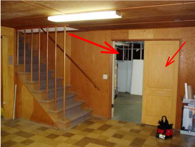
doors are solid to utility are....
