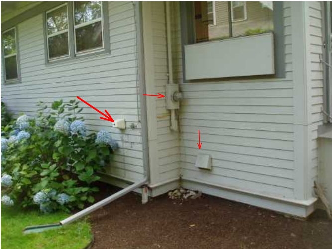
electric meter, good...exit vent for stove, kitchen...good...hose bib is covered...
