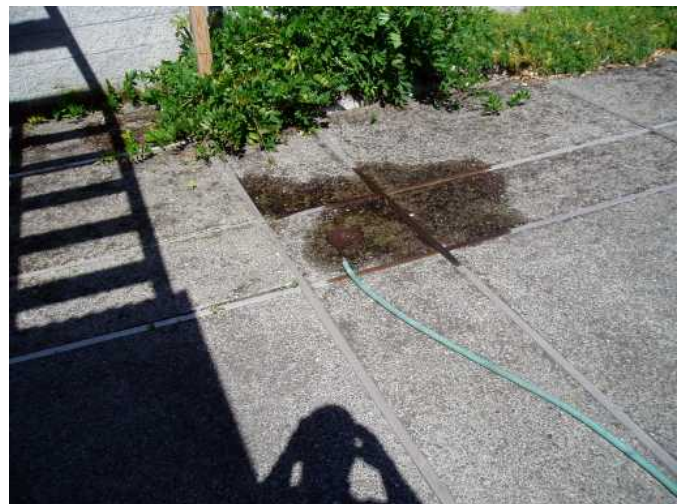
surface drain works well...patio...
