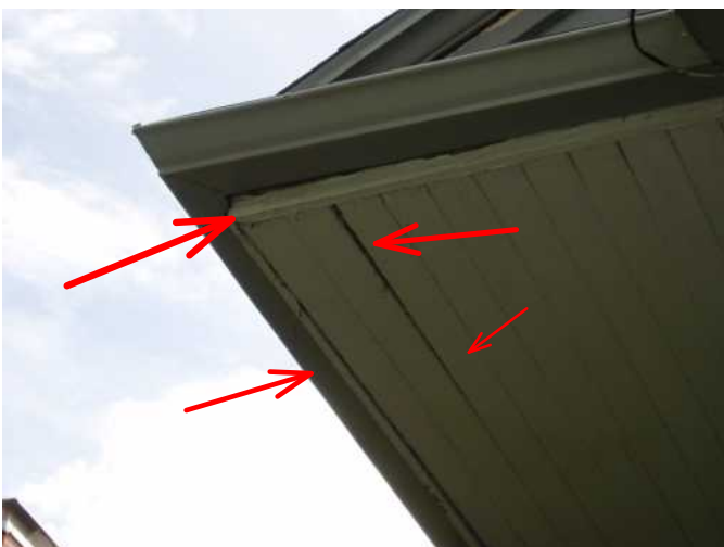
monitor this corner at rear of home...is a bit loose ...maintain paint to keep from getting any worse....
