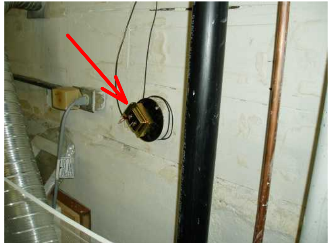
doorbell converter keeps low voltage to door bell button...
