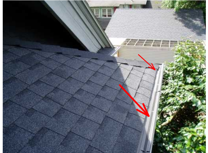
gutter covers are good at rear of home...
