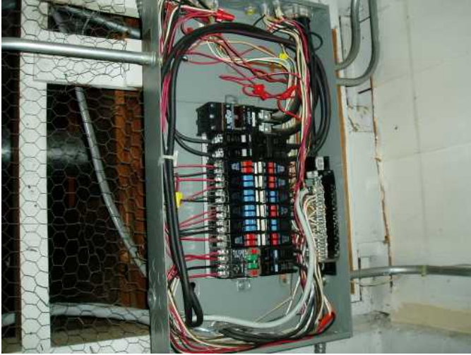
inside panel looks fine...200 amps and 100 amps to sub-panel in attic...
