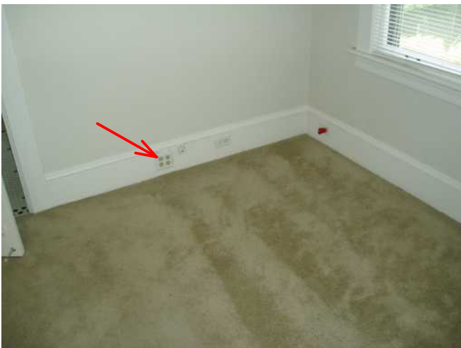
outlets here are grounded...
