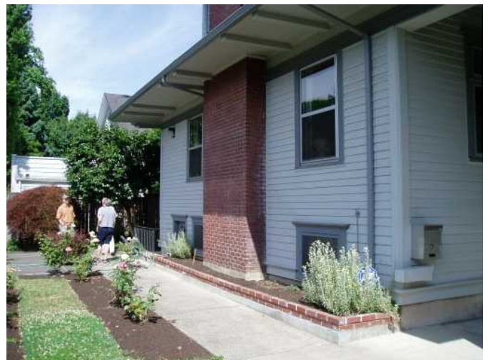
side of home siding is in great shape...trim is well maintained...
