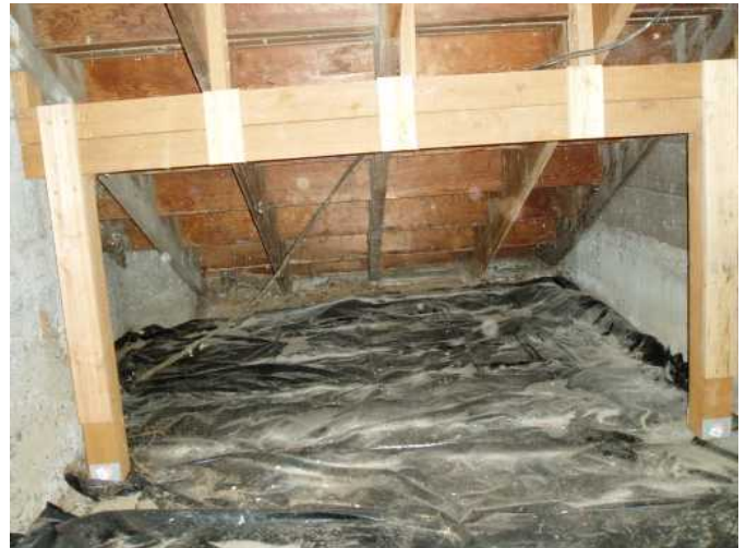
new stair support beam...moisture barrier..good...
