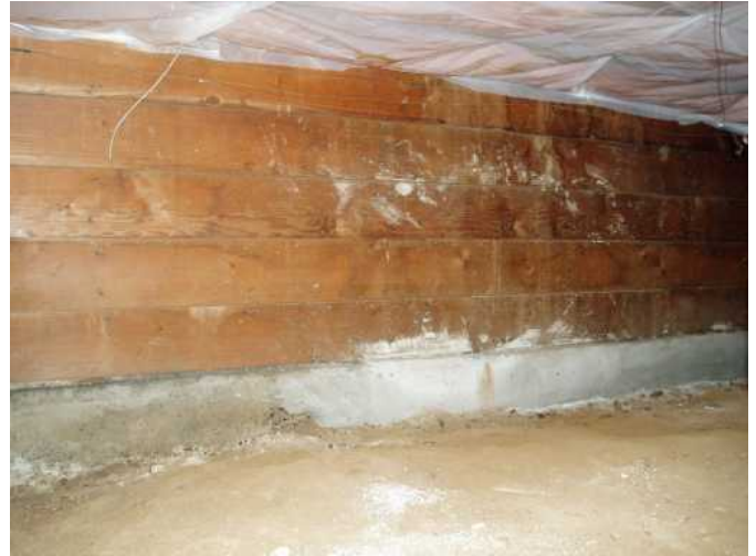
crawl space in back area of home..good...
