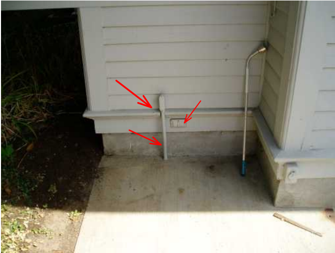
electrical exit to garage..and exterior outlets are grounded...fine...
