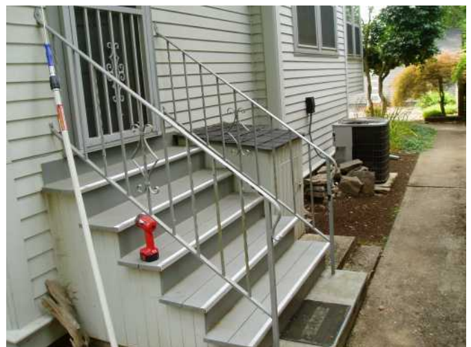
rear entry stairs are solid and sound...hand rails are solid as well...
