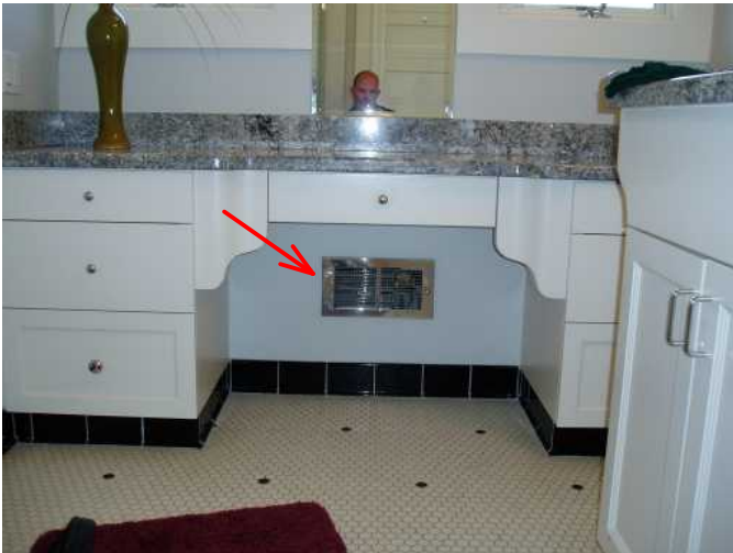
zonal controlled cadett heater works fine...
