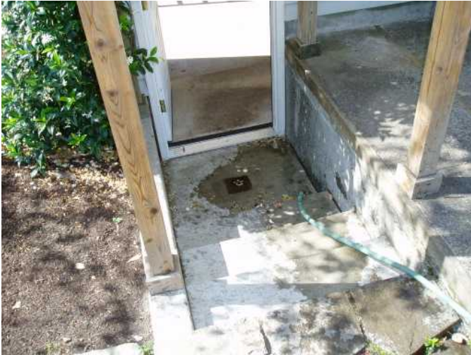
garage entry drain works fine...
