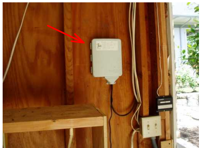
water sprinkler control box in garage...fine...
