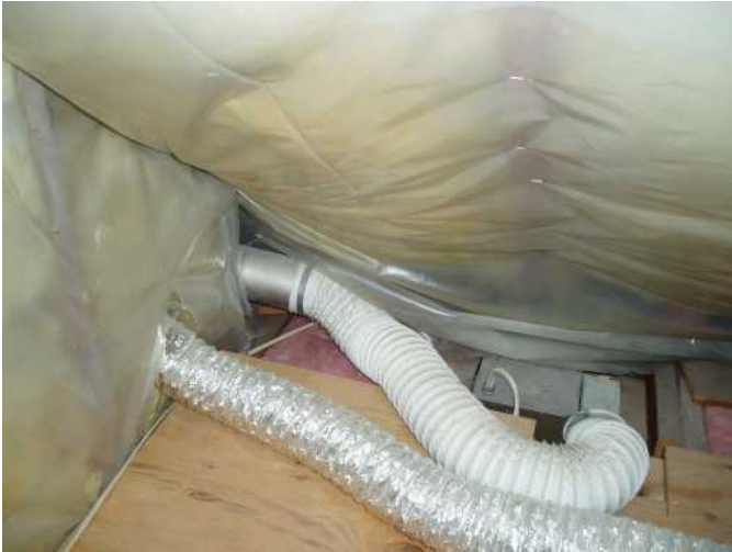
both bath vents are vented to outdoors..good...
