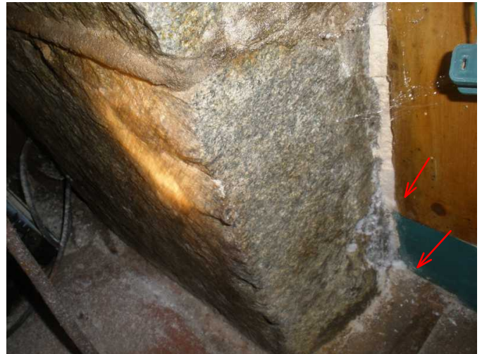
efflorescence noted at both sides of lower area of fireplace...
