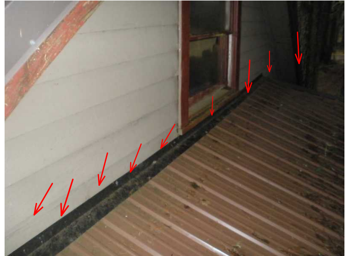
metal roof flashing to siding is noted over siding and should be under it...did note high moisture at wall area in bath
