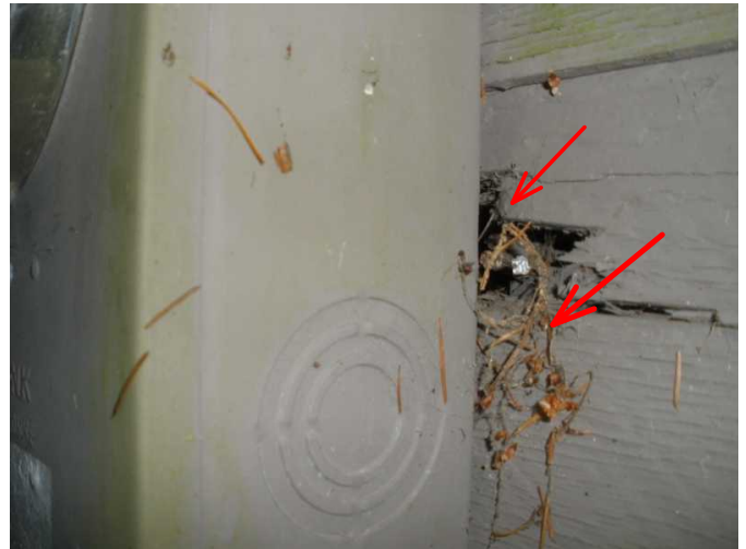
open gap is noted at electric meter area...close up...and seal...
