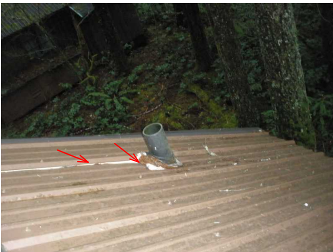
noted main sewer vent is noted with caulk at flashing and will need new caulk in spring...to ensure sealed...
