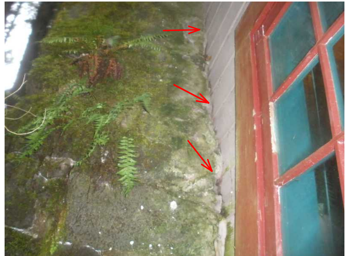
both sides of fireplace are noted with open gaps to siding at west side of home...and trim needs paint...correct..
