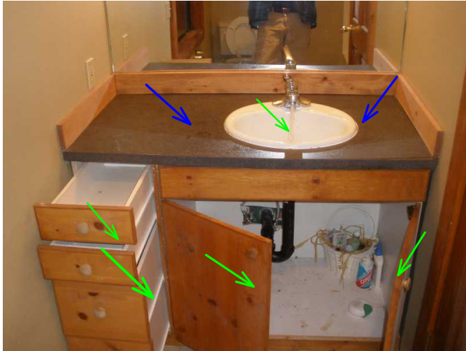
cabinets noted operable...sink is fine...counter is damaged and will need replaced...
