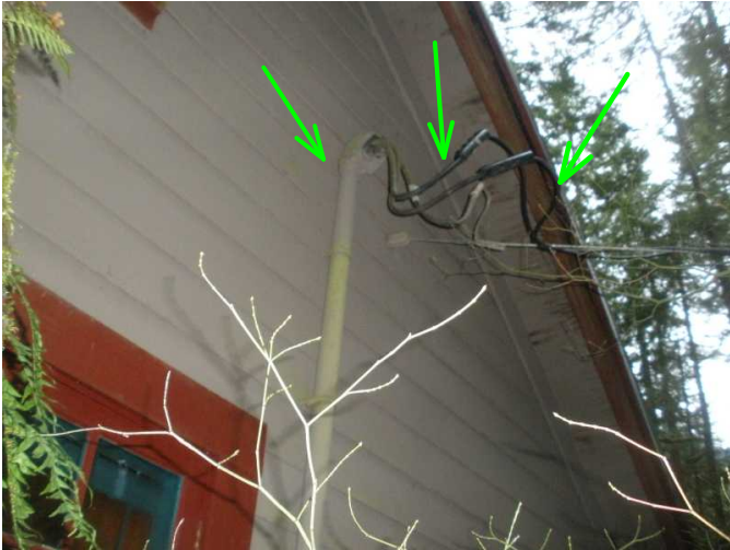
main electric entry is noted here at west side of home...drip loops are noted fine...
