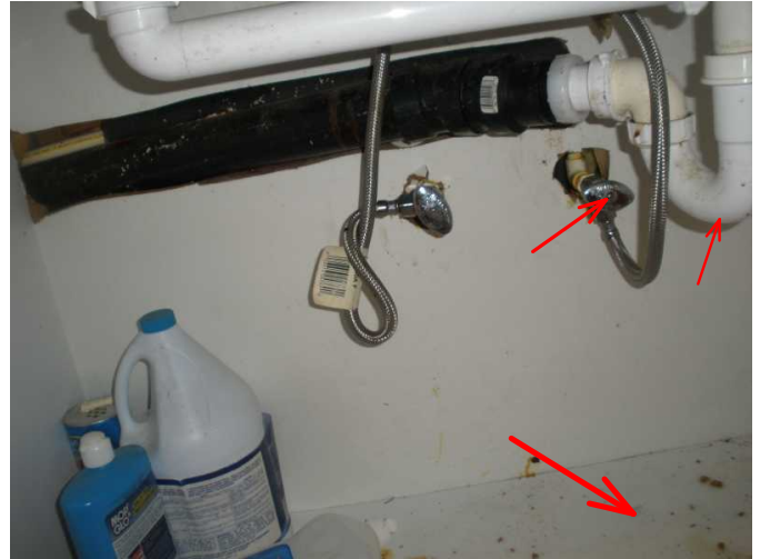
leaks noted and will need repaired...may need to assess water lines in wall..did note leaks at exterior siding as well....
