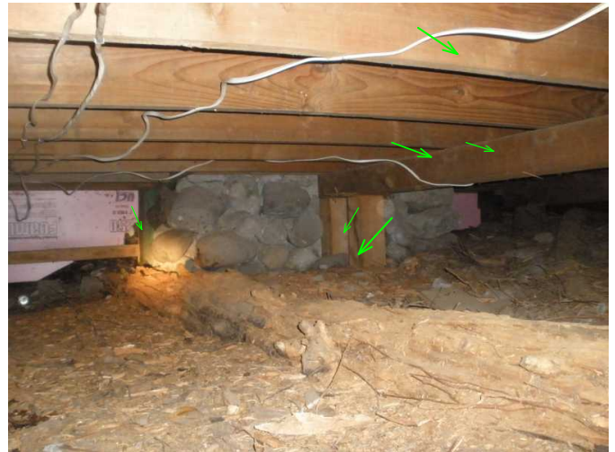
joists and posts are noted solid...but rotted wood needs removed...recommend adding under floor insulation...
