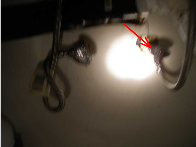
under sink is noted with leaking at connection to right...and trap to right sink as well...
