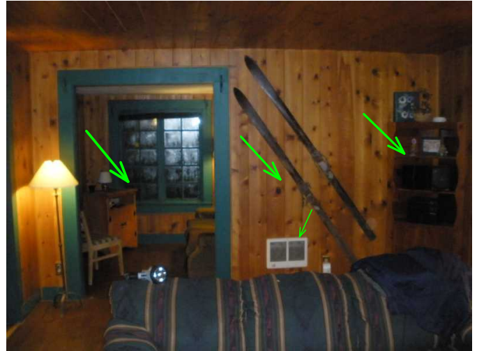
cadet heater is noted fine as well...walls are solid wood and are fine...some higher moisture detected...leave heat on...
