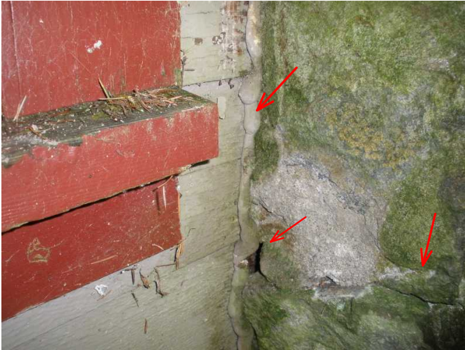
fireplace is old and has issues with seal to siding..is letting in water to home...have assessed and repaired/replaced
