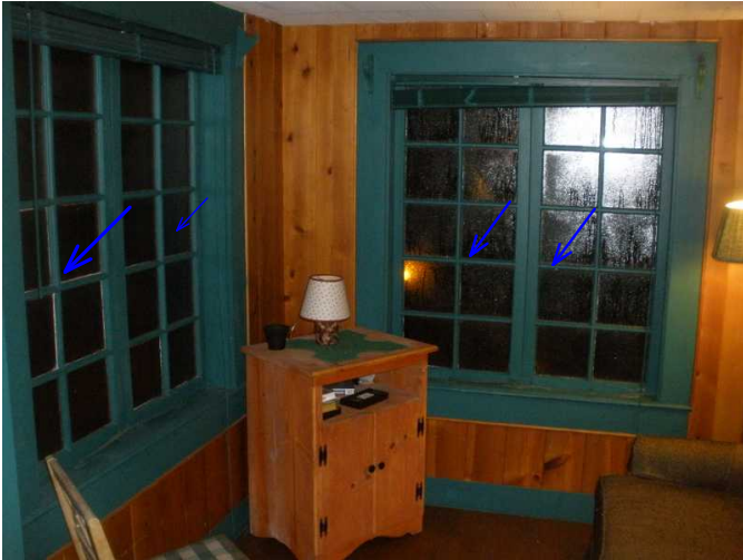
study area noted here with windows not operable...condensation noted...
