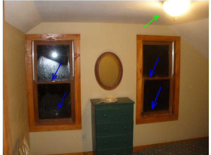
bed 3 ceiling fixture is noted operable..all outlets noted operable..windows not operable..and single pane....
