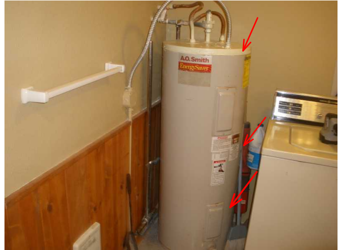
water heater is noted here with no earth quake strapping and was not very hot water noted...is older unit...
