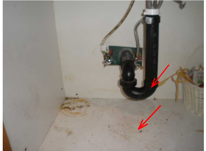
drain trap under sink is noted leaking...correct...
