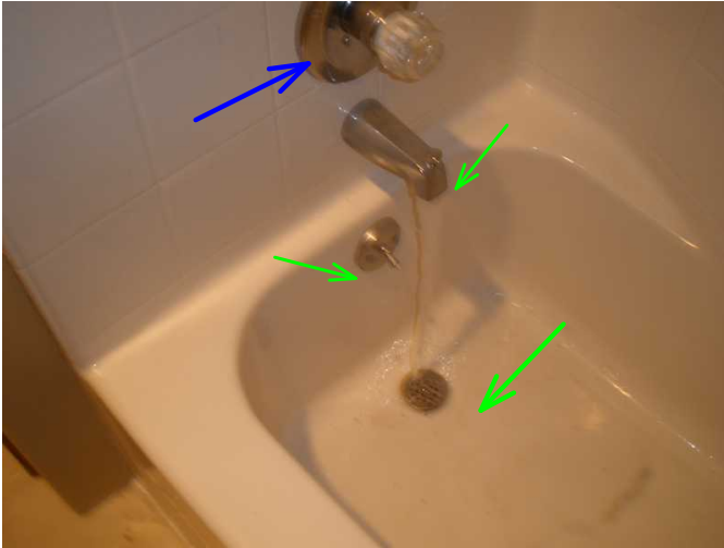
tub faucet is noted loose...operates....drain and drain stop noted operable...
