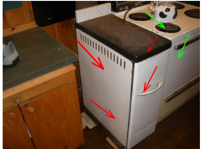
the wood burning cook stove is not acceptable and will need to be removed...is not DEQ approved...main stove is operable
