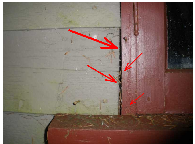
any and all open gaps need sealed to close off the exterior of home and avoid water entry...is issue with this area..
