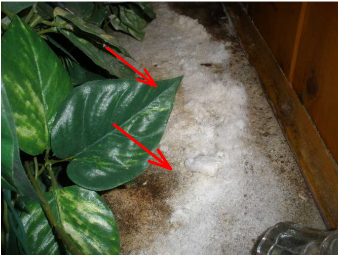
this is the mantle of the fireplace with salts...(efflorescence) appears the fireplace may need replaced...very wet...
