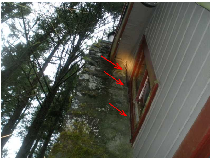
large open gaps are not good...have assessed and corrected by licensed mason...
