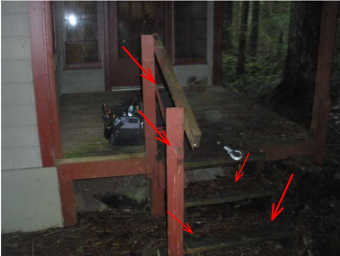
handrail and steps need repairs...wood touching earth and handrails are loose...
