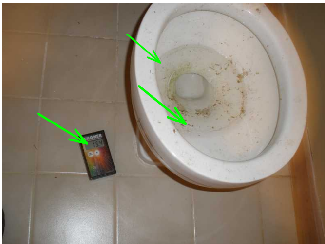
toilet is noted solid to floor and operable...does run after flushed...correct...floor moisture is fine...
