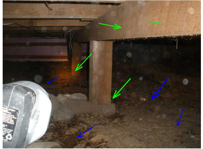
all wood under home is noted solid and raised..remove all rotted wood on earth and add vapor barrier...
