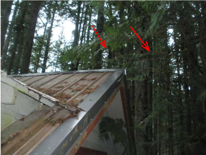
cut back tree overhangs at roof area...east side upper gable...
