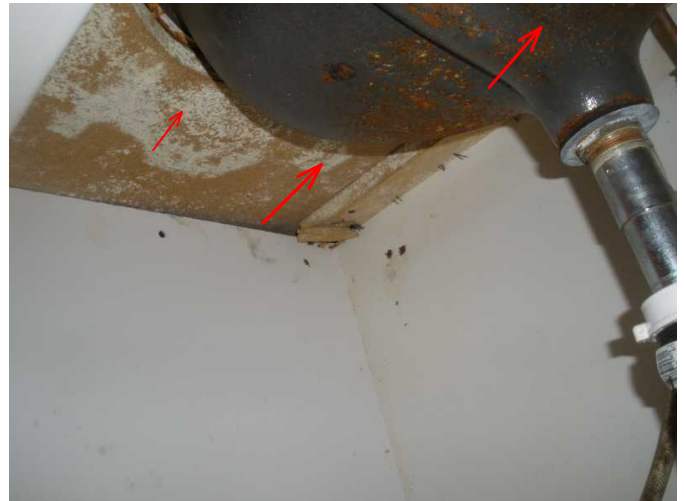
underside of sink counter area is noted damaged from water...is sinking in center...replace...
