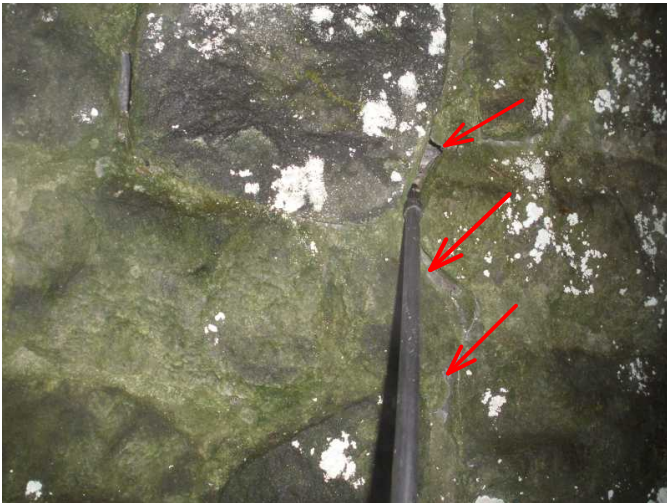
many gaps noted in fireplace to allow in water and leaks...correct...may need re-build...
