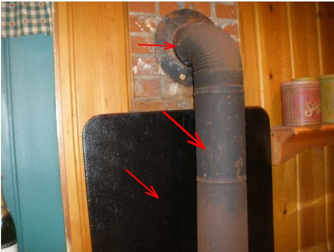
the single wall flue is noted here and is noted to close to wall...has simple wall protection,. but needs secure brick..
