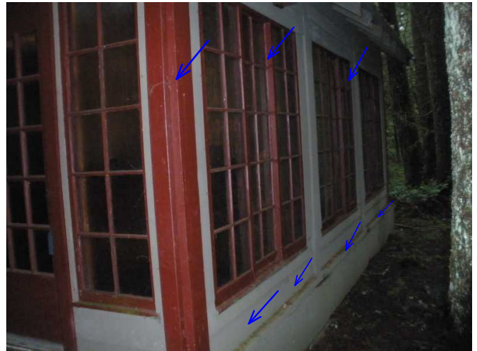
north view of home...trim and siding need paint...
