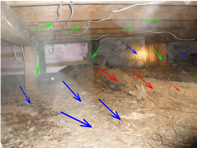
remove rotted wood...add vapor barrier and noted the base of fireplace is here...assess mortar joints...posts are solid...
