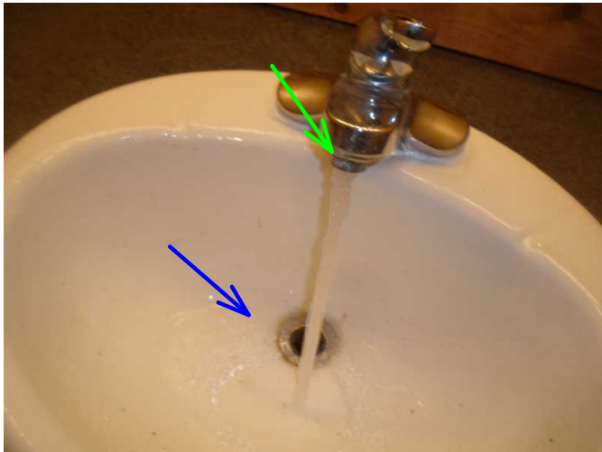
faucet is noted operable..drain is noted operable...no drain trap noted...correct...
