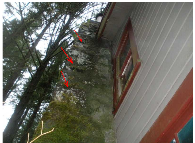
efflorescence noted at exterior of fireplace...is letting in dampness and getting wood wet...correct...
