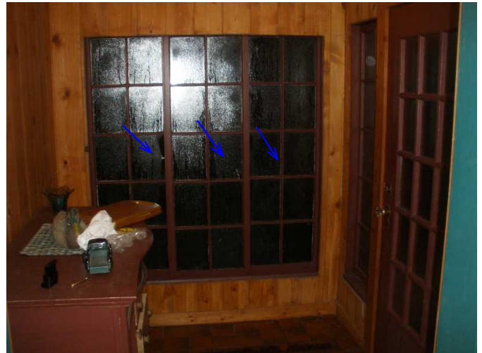
entry noted here with windows not operable..and condensation noted ...
