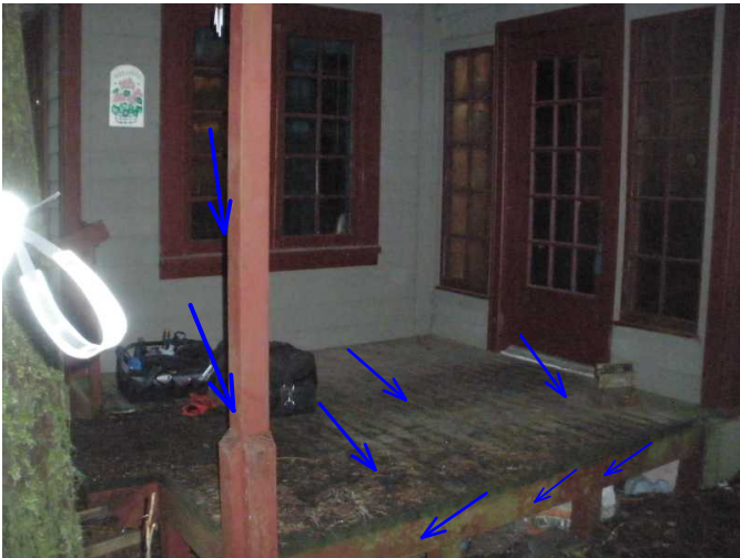
general view of porch is noted solid...just needs some cleaning and sealant on wood...paint to trim needed...
