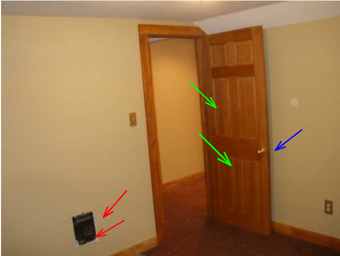
bed 3 entry door and wall heater...wall heater needs cover plate and entry door needs door stop...operable...but swollen
