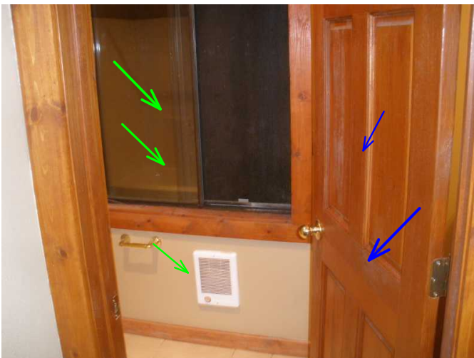
second floor entry to bath door is noted operable..but swollen as noted all doors...heater and window noted operable...
