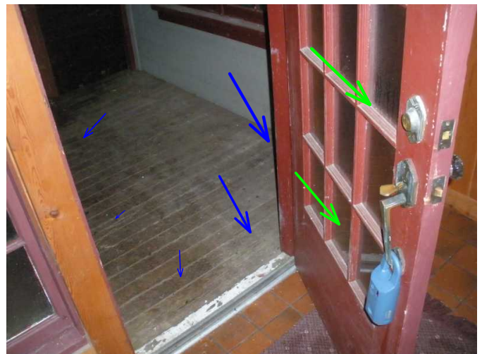
main entry door is noted operable...recommend adding weather stripping around entry door...
