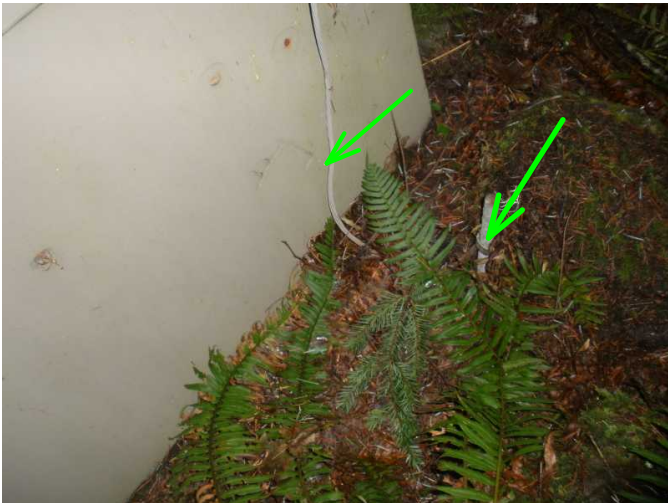
grounding wire is noted here at earth below meter at corner of home...
