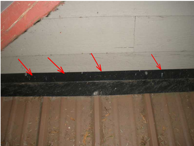
this flashing at roof to siding will need repaired to have counter flashing or plenty of caulk to seal...appears leaking
