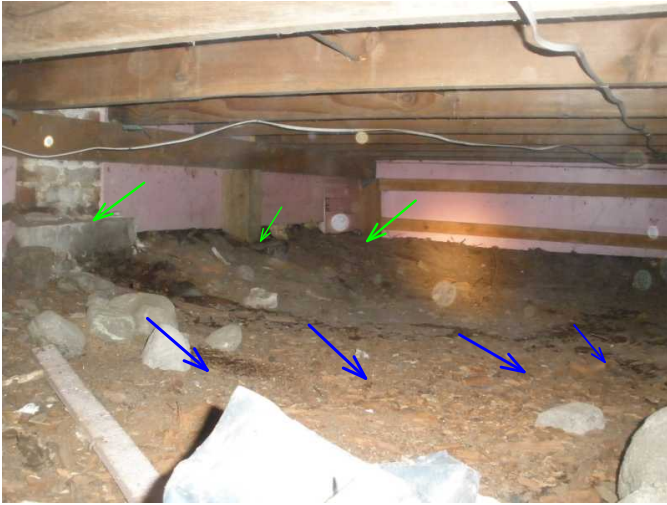
all post under dining area are noted raised on rocks/recommend pads...no vapor barrier noted for most of crawl..correct...
