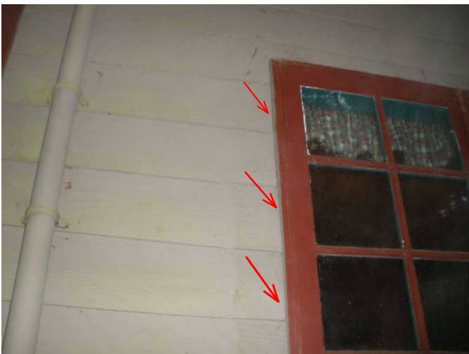
open gaps noted at dining area window at west side...seal with caulk...
