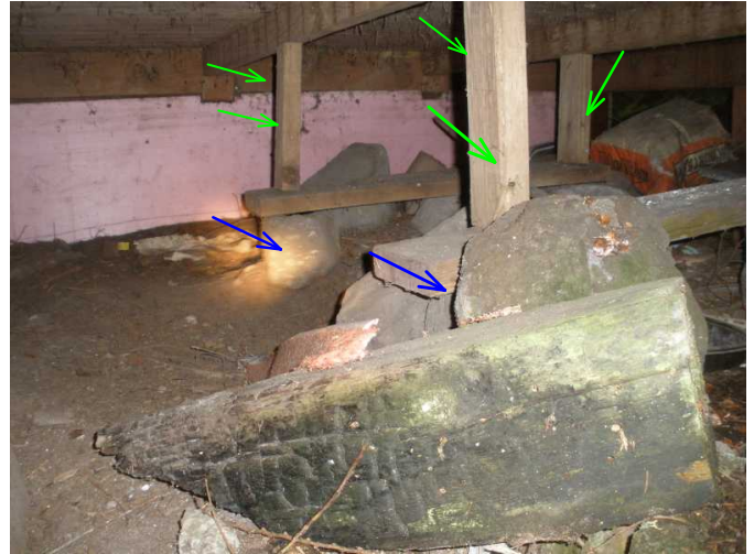
all supports under porch are noted dry and solid...on rocks and pads...raised...recommend adding pads..not rocks...
