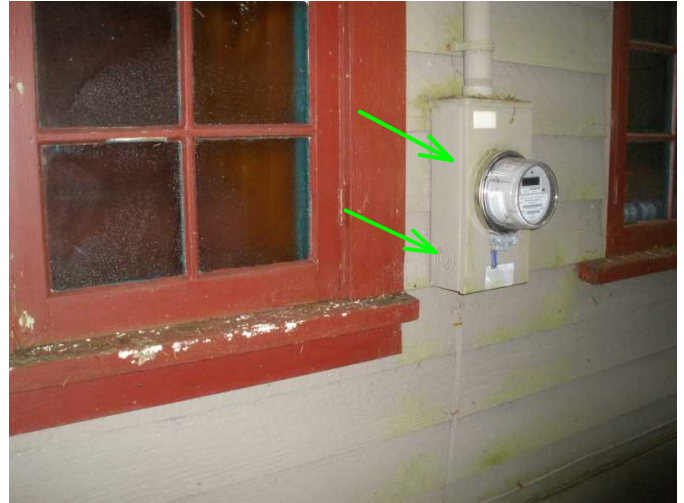
meter is noted fine and is solid to siding...
