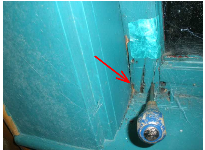
rot noted at window to right of fireplace in living room...correct...
