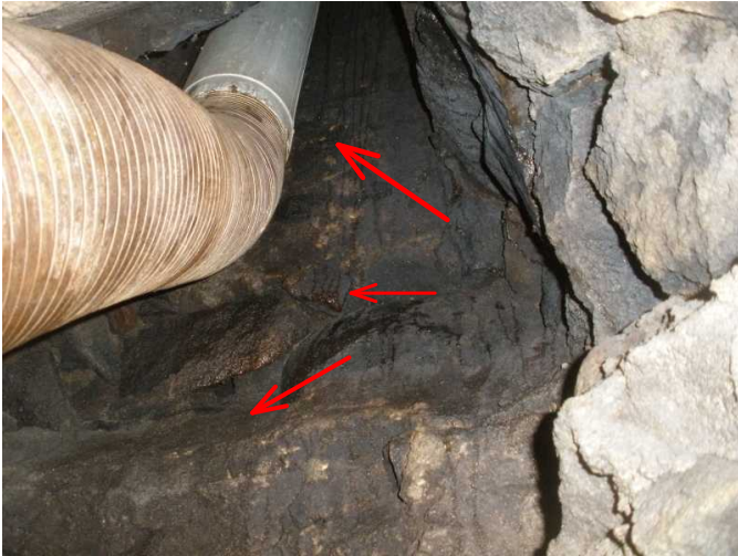
the wood stove insert is noted with single wall flue installed up the original chimney... no damper noted...
