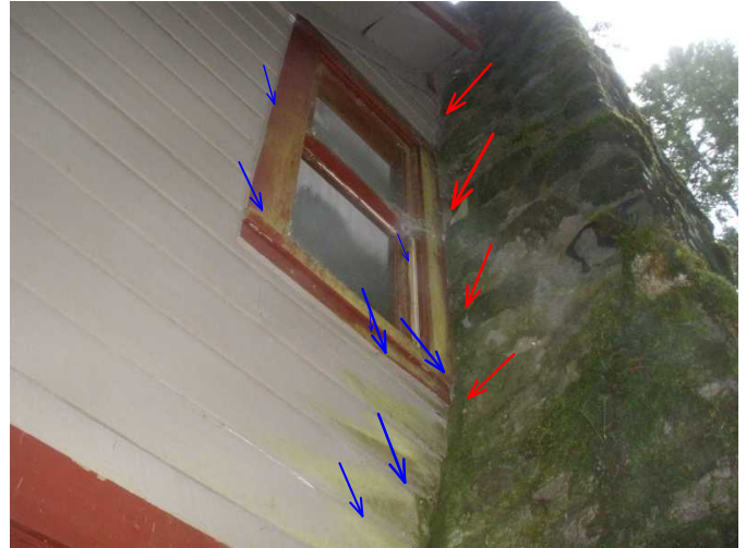
siding and trim are noted here with algae and fireplace is noted gapped away from siding..allowing in rain water...
