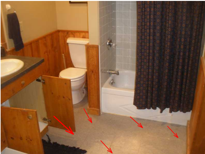
overall view of bath is noted here...the floor is high in moisture...from past water line break...
