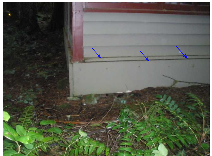
paint all trim and siding and seal any open gaps noted at trim to siding...
