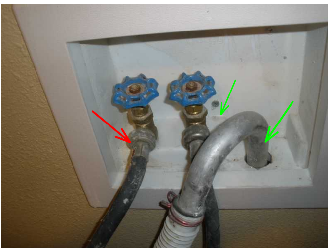
main hook ups for washer are noted here and are operable...left valve is noted leaking...correct...
