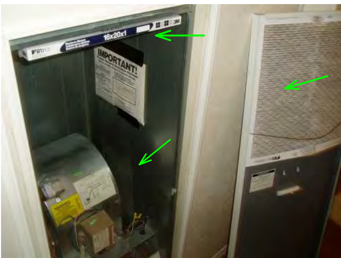
open view of electric furnace is noted here and has two filters....fine....
