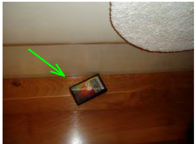
no high moisture noted at floor area as well....good...
