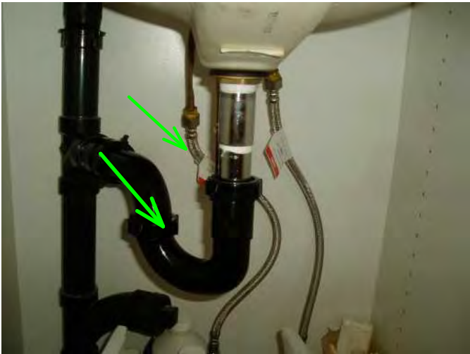
again, better quality found here under sink and no drips or leaks noted....very good...
