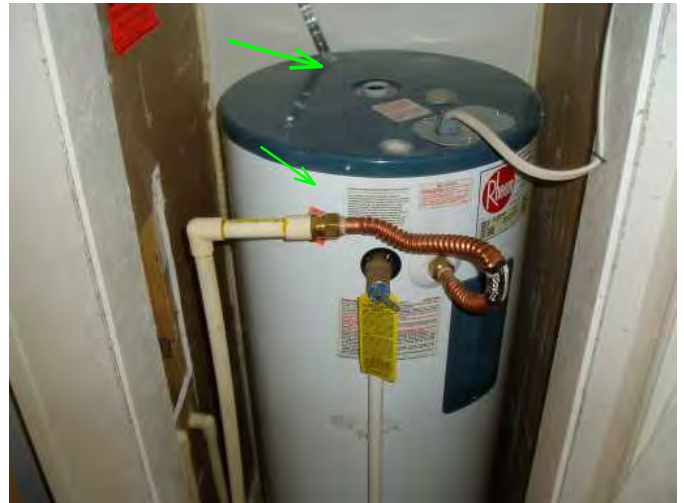
water heater is fine and is strapped in its own odd way...fine...
