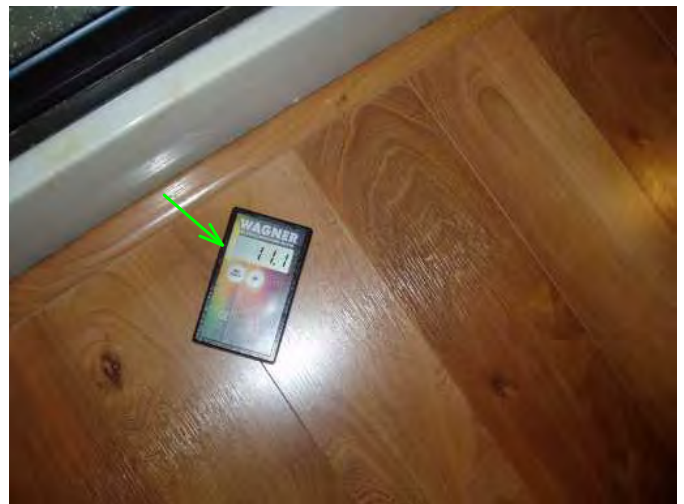
no high moisture noted at floor area....good...
