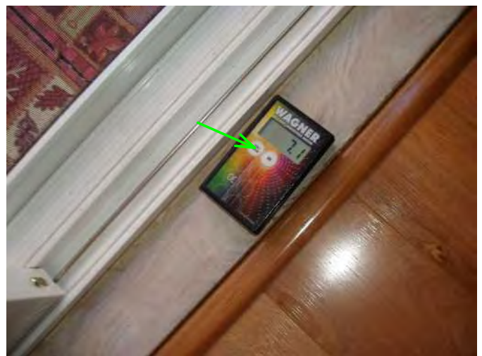
no high moisture noted at slider door area....good...
