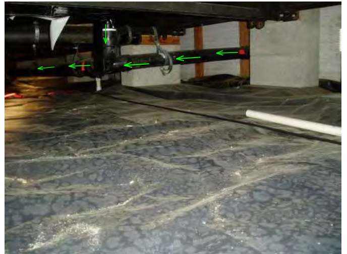
main sewer and clean out noted here and all drip free...good...
