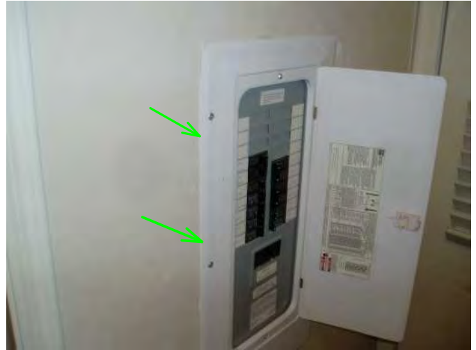
main breaker panel is noted behind back door area....
