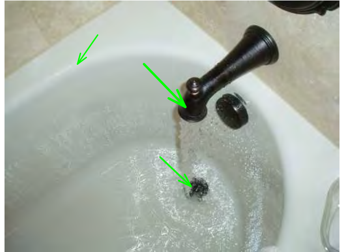
tub fixture and drain are operable...is better quality fixtures as well...good.....
