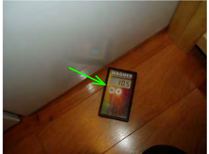
no high moisture noted at washer area....good...
