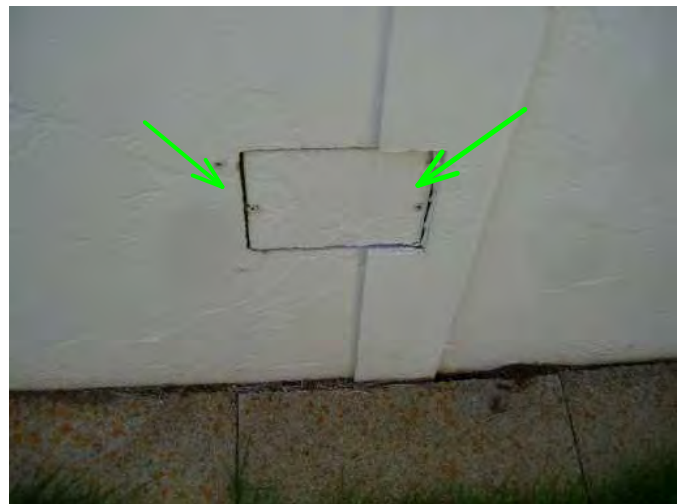
sewer clean out access hatch...good...
