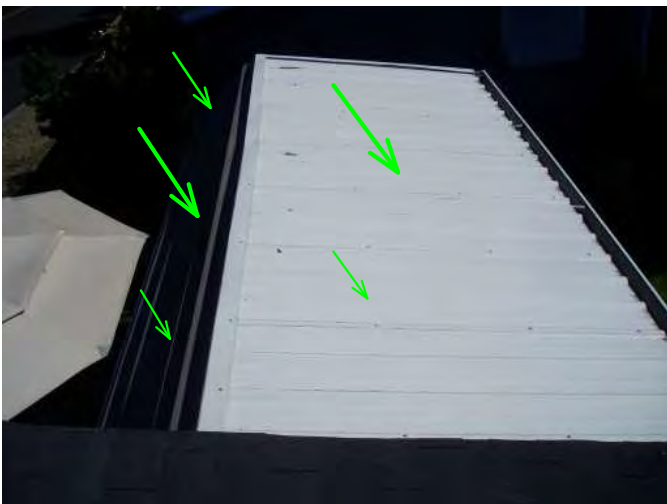
deck metal roof over covered deck area and wood siding at front area noted as decorative finish...keep painted...good
