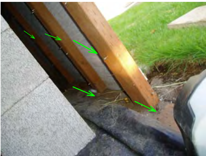
all skirting framing is treated wood...all of this home is proving to be better quality than I normally find
