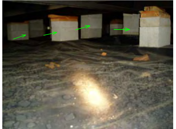
all of home is on blocks and wood levels...solid and sound...all of under home is clean and dry and insulated...good...
