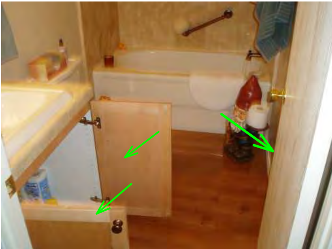
entry door to front bath and cabinet doors are operable...good...
