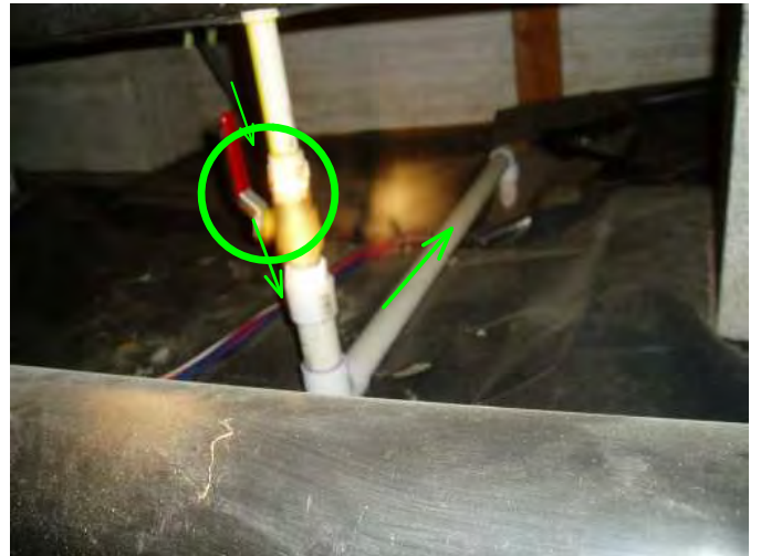
this is pipe to supply to irrigation system for lawn...has shut off for winter...use to keep from freezing pipes...
