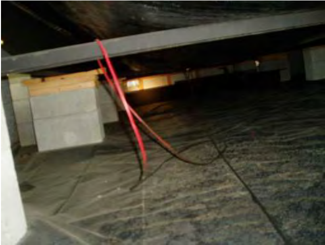
under home is clean and dry and appears to be checked regular....good...
