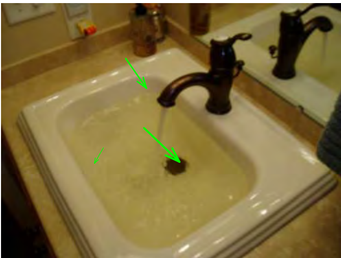
faucet and drain and overflow are operable...good...
