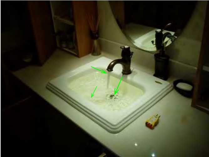
master bath sink faucet and drain and overflow are operable..good...
