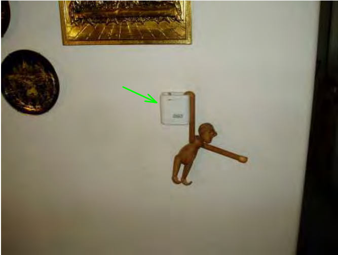
thermostat is noted in center of home in dining area....change filters every 30-60 days when in use....
