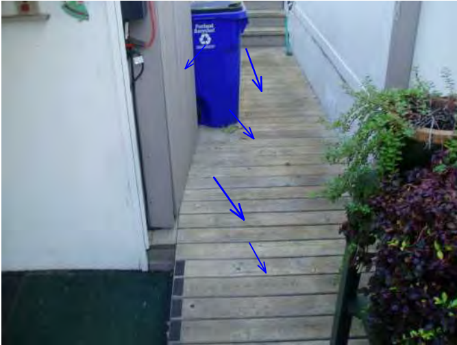
wood is solid and sound...will need to be cleaned and sealed to extend useful life...gate is solid...good...
