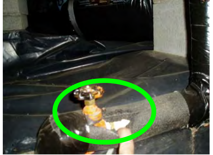
main water entry shut off and pipes are C-PVC and are fine..insulated as well...good..
