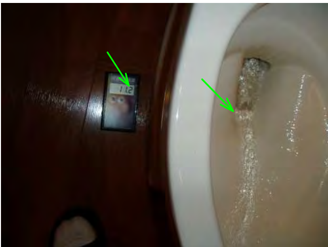
toilet is operable and no high moisture at floor is noted...good...
