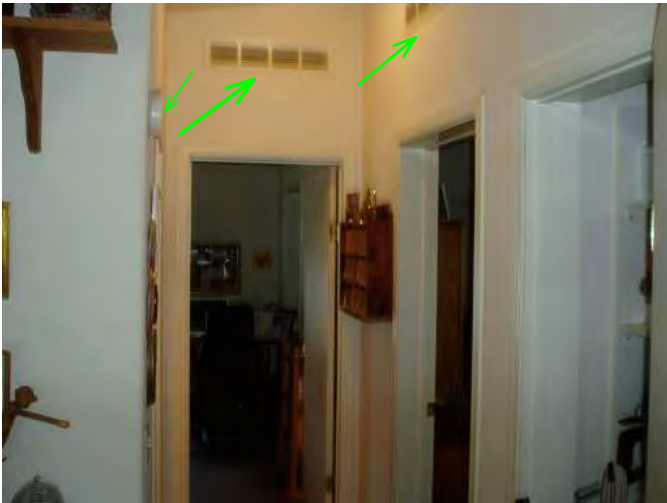
small hallway area has vents above doors to allow air flow around home...and noted smoke detector in hall...
