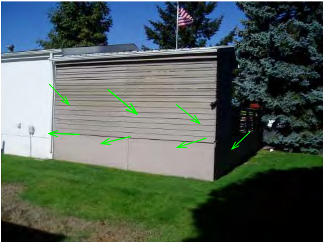
back area of small covered deck area...good...has plastic baffled sections to cover in winter to keep out rain...good..
