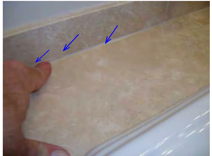
minor issue here needs to be caulked.....
