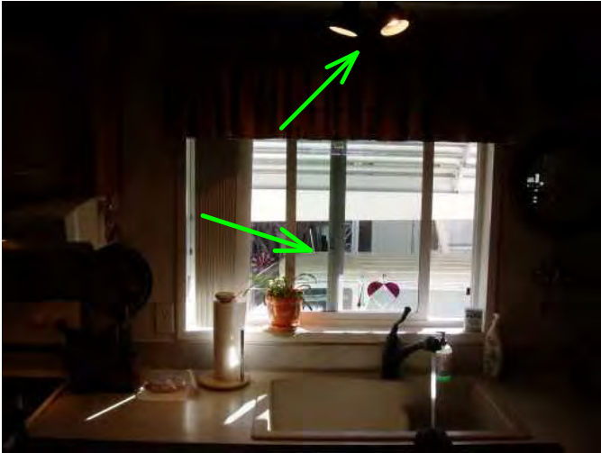
kitchen window and fixture and faucet are operable...good...
