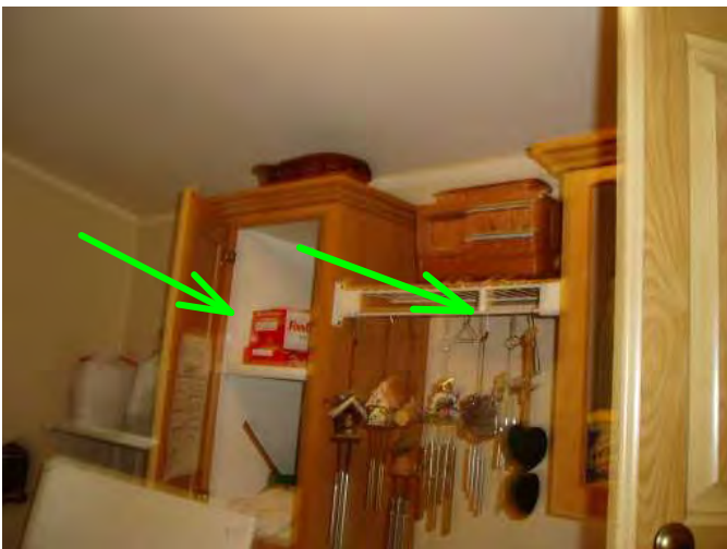
upper laundry cabinets are solid to walls and operable..good...
