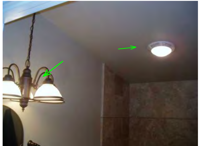
fixtures and exit fan are operable in bath as well....good...
