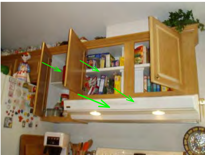
over stove cabinets and exit fan are operable...good...
