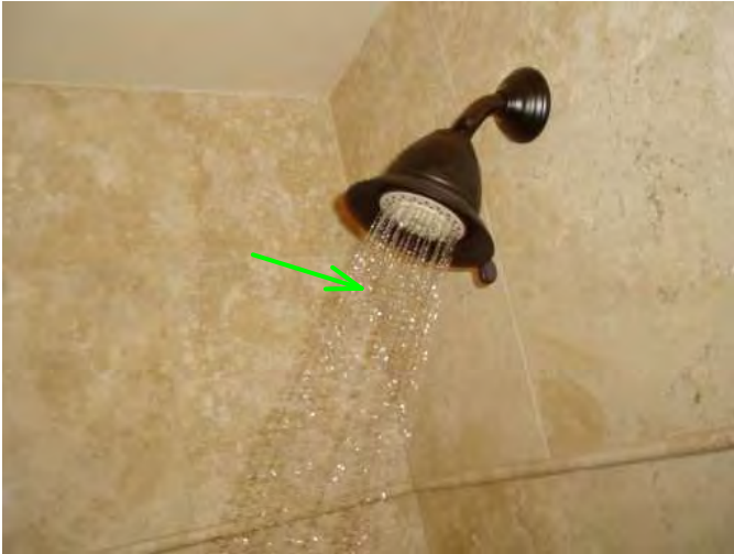
shower head and shower walls are operable...walls are awesome! not noted in any other home in area!!
