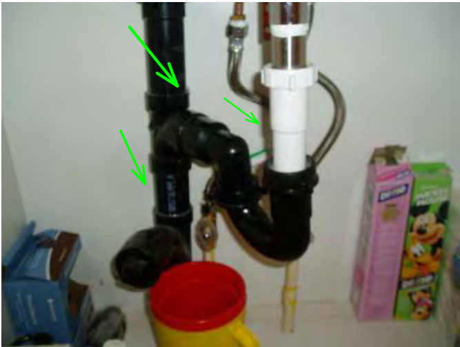
no drips or leaks noted under sink area....good...
