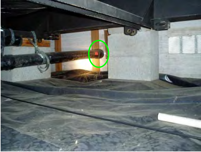
main sewer access has outdoor access clean out hatch for easy access when/if needed....
