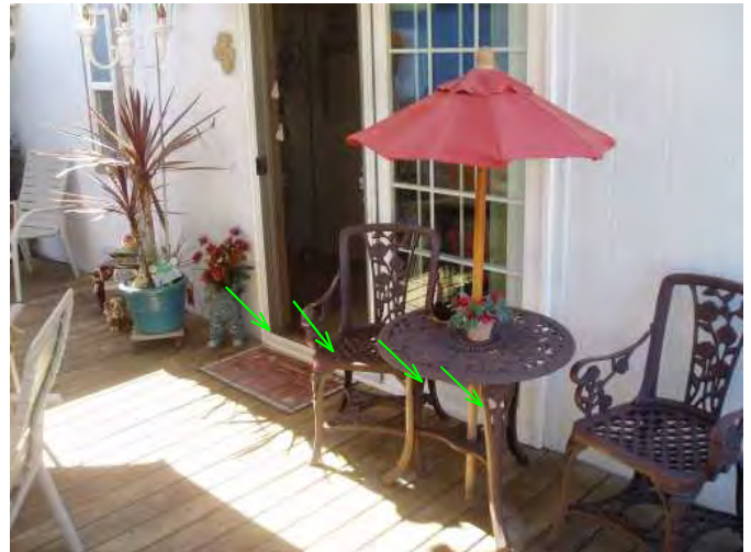
patio slider door is higher than deck...good...raised to keep out rain water...good..
