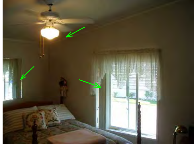
bed 3 windows and fixture and fan are operable..good...
