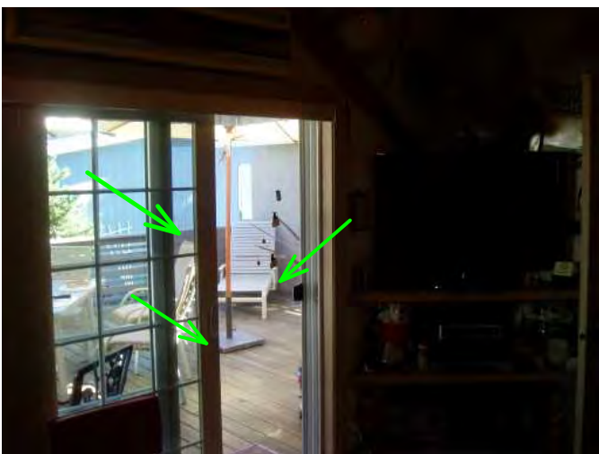
patio slider in master is operable..good...
