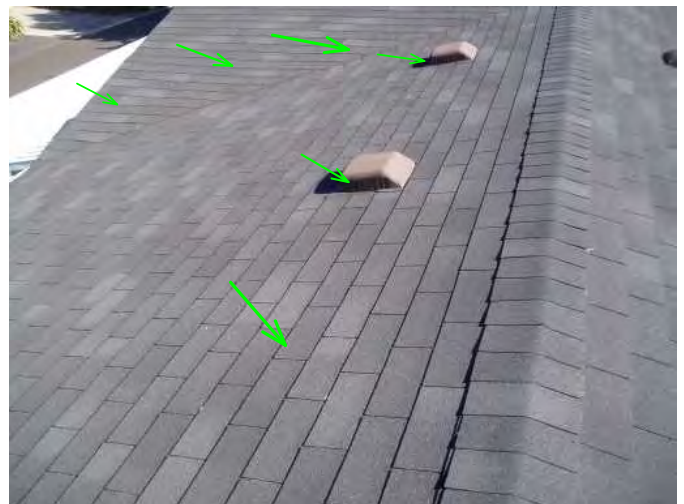
facing back of home on roof and noting clean and solid. ...shingles are fine...vents are fine as well...
