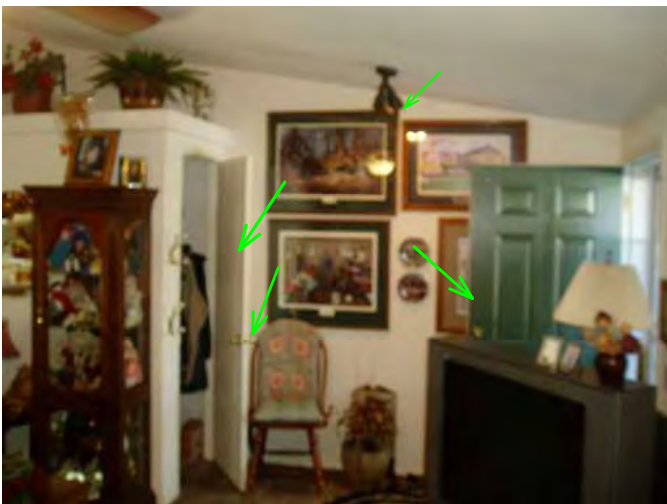
fixture and entry and closet doors are operable...good...add door stop discs wherever needed....
