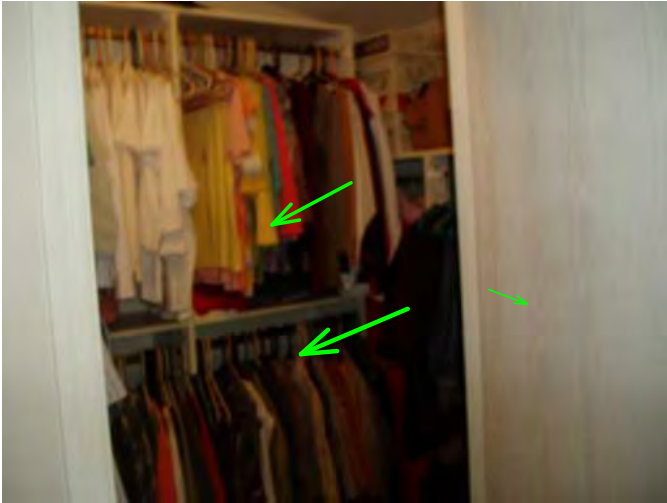
bed 2 walk in closet entry door and shelves and fixture are operable....good...
