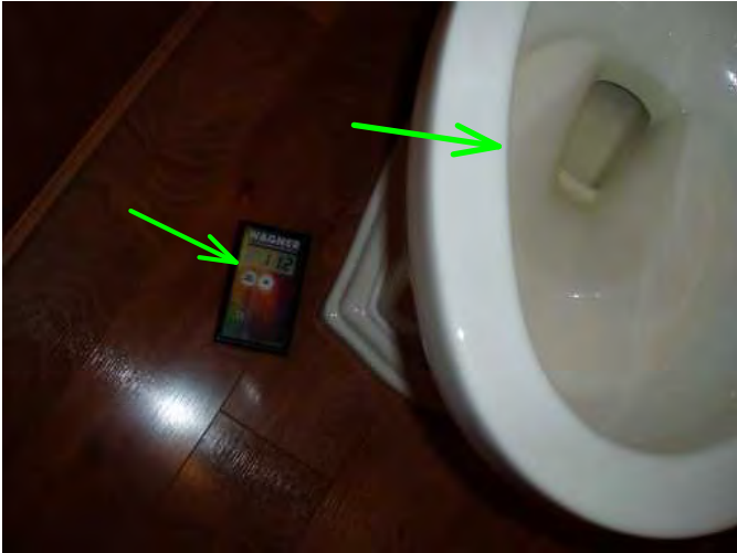
toilet is operable...and no high moisture noted at floor area....good...
