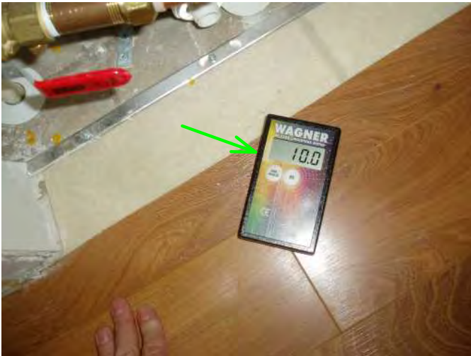
no high moisture noted at floor area at water heater area...and noting old flooring was not as nice as wood new....
