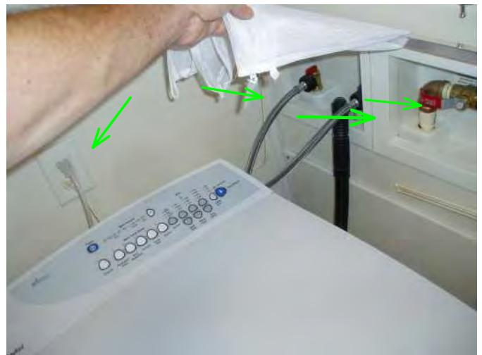
washer hook ups are fine..noted hot water heater has shut off in wall area....good....
