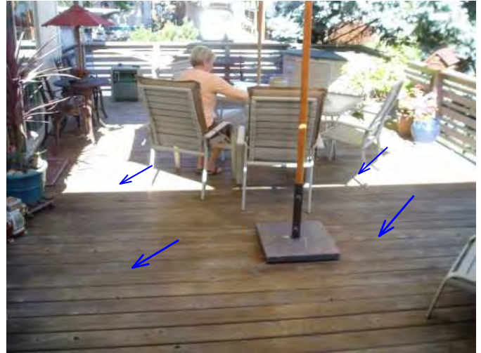
main deck and handrails are solid and sound...deck surface should be cleaned and treated/sealed
