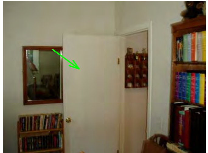
bed 3 entry door is operable...good...check all doors for door stops and add disc to wall if missing ...
