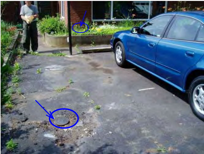
oil tank and vent noted here at driveway...
