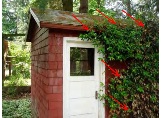
remove all vegetation that creeps onto structures..can not maintain and see what is going on with structure...
