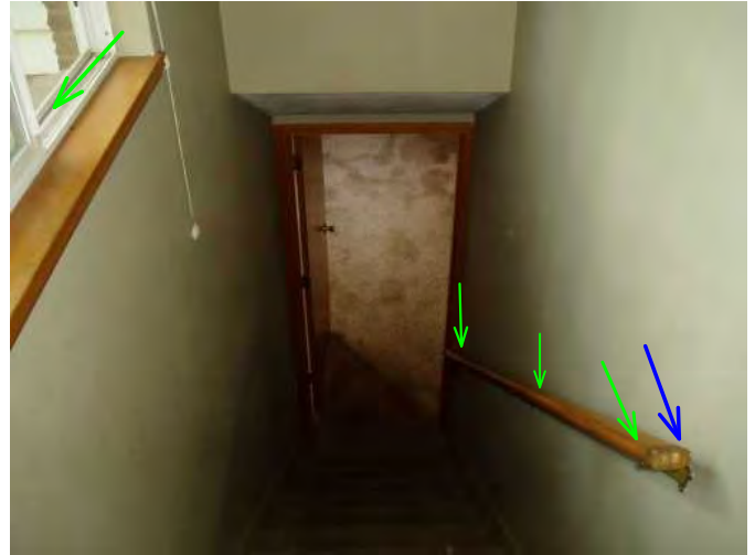
window in staiway is operable...handrail is solid...but needs repair...missing end piece...
