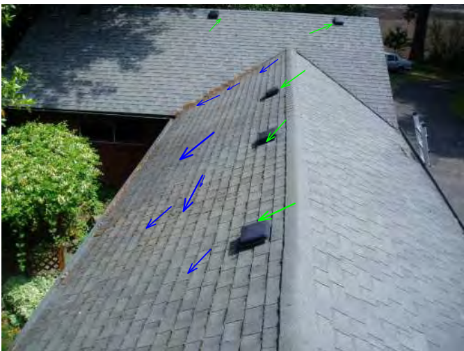
over back area and breezeway to garage roof at back, just needs cleaned valley and some moss removal...
