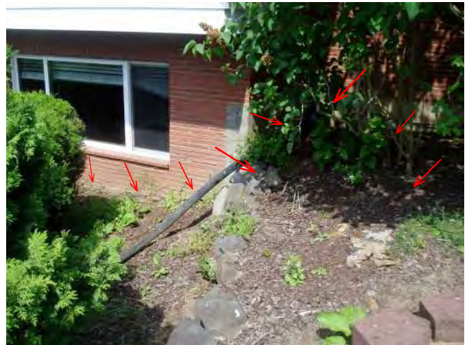
red arrows signify issues to address...this is area of great concern for family room walls and drainage at outside....
