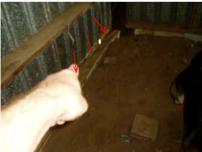
mud sills need to be kept from earth..or will need repalcement as this area is noted at back of pole shed....
