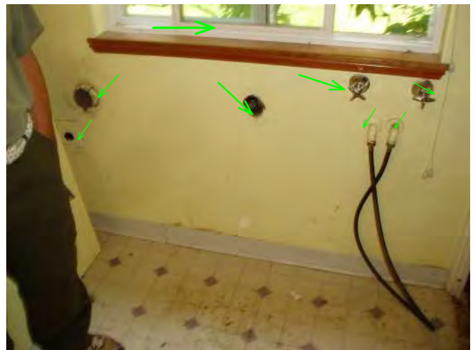
laundry room window and hook ups are all good here...
