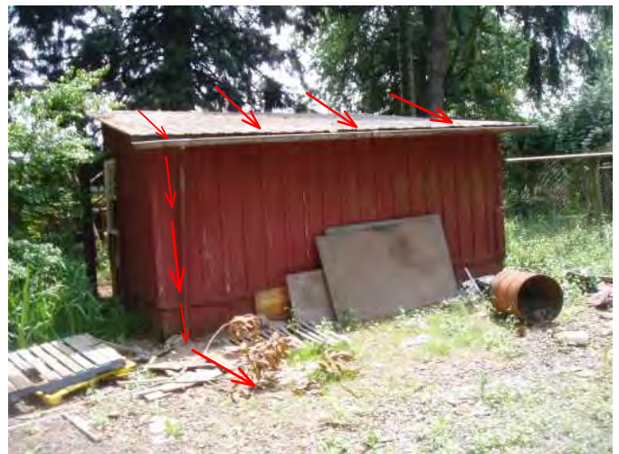
back of chicken coop needs gutter re-attached and downpout added adn extension as well...
