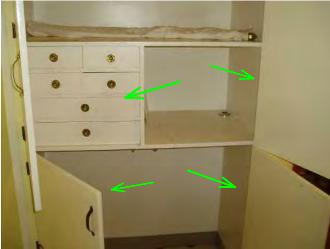
cabinets in laudnry room are operable...
