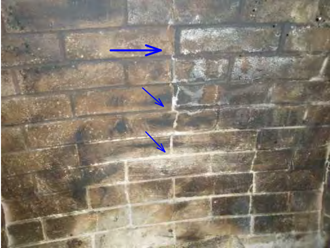
cracks in fire brick are needing sealed, but are not fire threat...repair...
