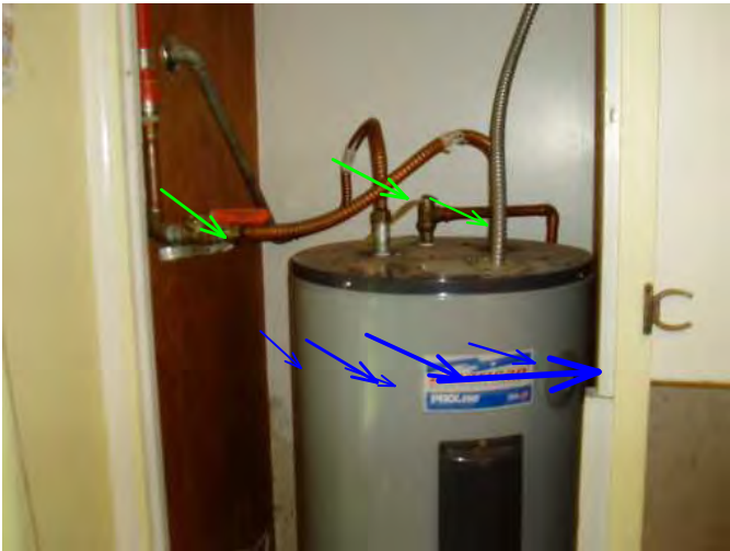
upper area of water heater in laundry room is noted as fine ..but needs strapped to wall...
