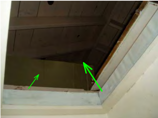
going up into attic in upper home area above bedrooms....in hall closet access...
