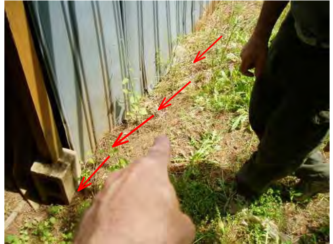
pull back earth from back of structure..this is at pole shed...
