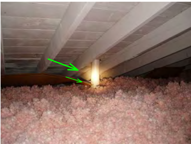
sewer vent and sheathing are good here...
