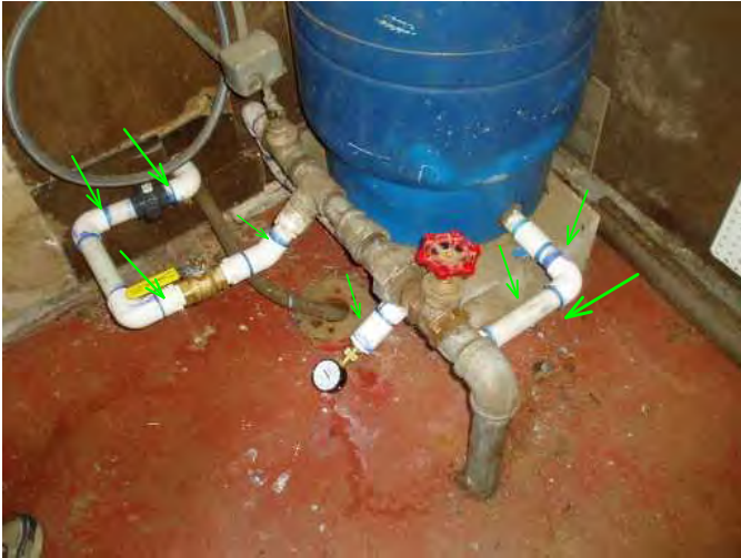
noted many new parts here in plumbing..very nice....
