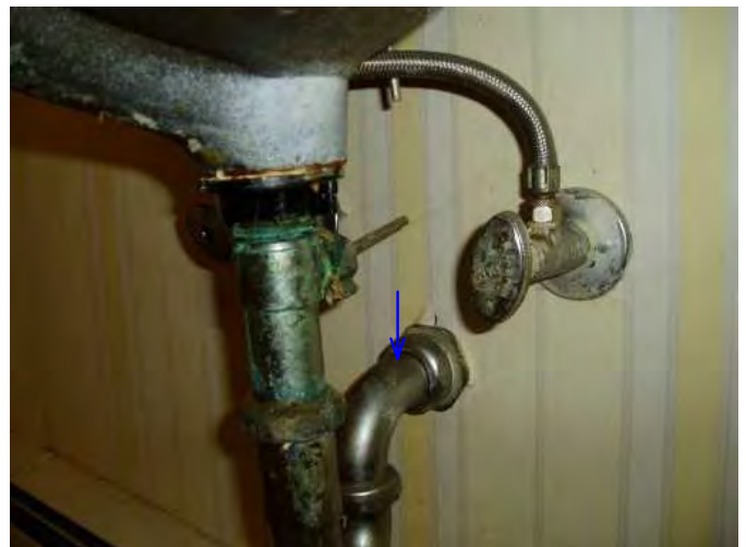
dripping at trap area under sink...
