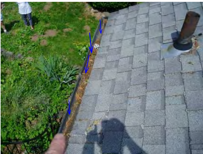
back area over patio shows full gutters and they are reversed flow as well...not good..re-hang...
