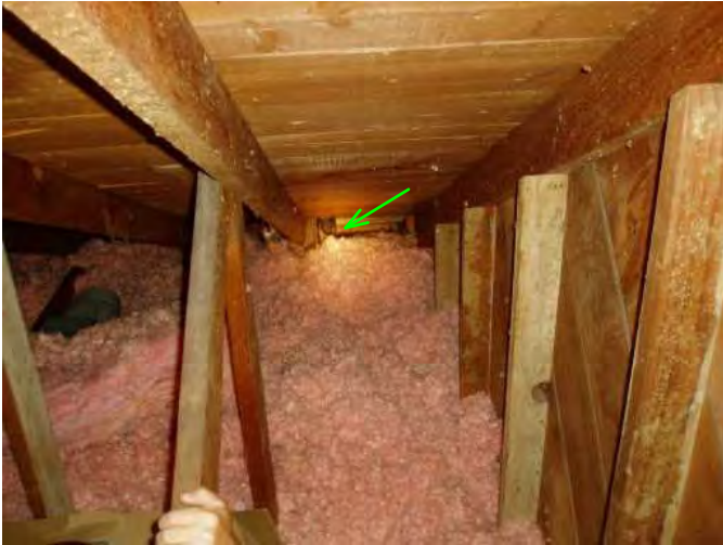
sewer vent is noted here over bath at back of home....
