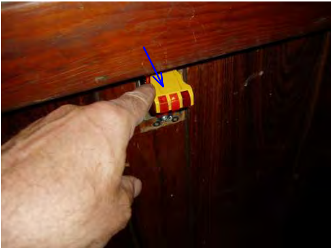
just noting that outlets in garage have 3 prong outlets, but are not grounded....
