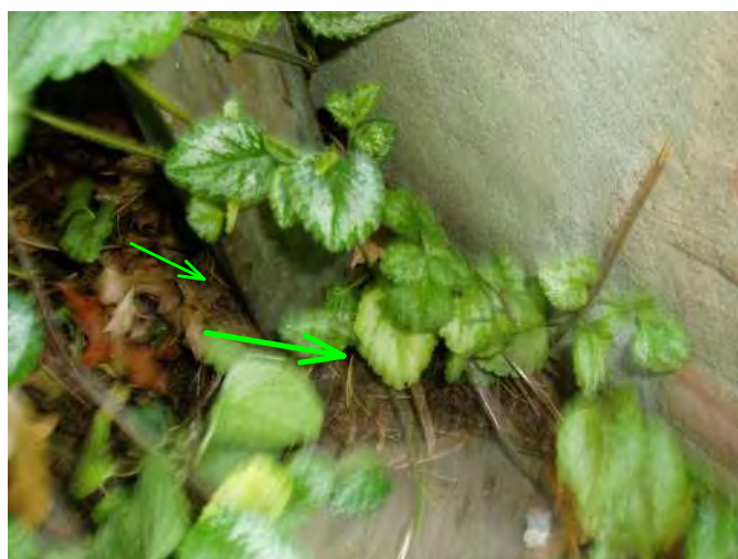
downspout at left of door to bed 3 is connected and draining....good..
