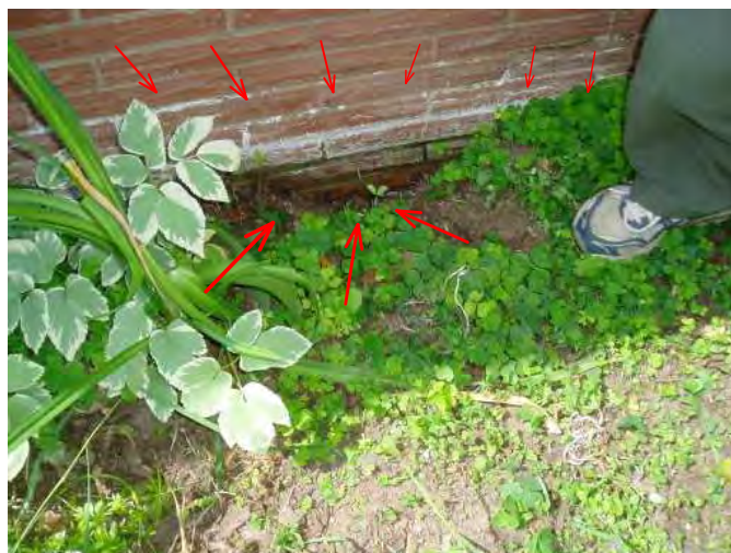
pulled back earth to show wet brick and white substance is spalling(salt from wet brick mortar) pull back earth...
