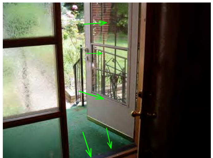
storm is operable, and threshold is solid...good..entry door area....good..
