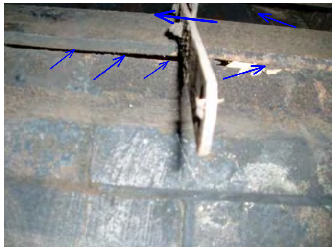
damper is needing cleaned, and will need sealed at base....
