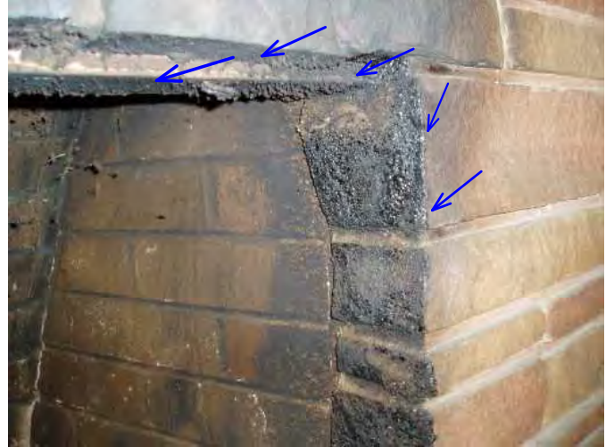
lots of soot noted here and in chimey flu and smoke chamber..have cleaned...
