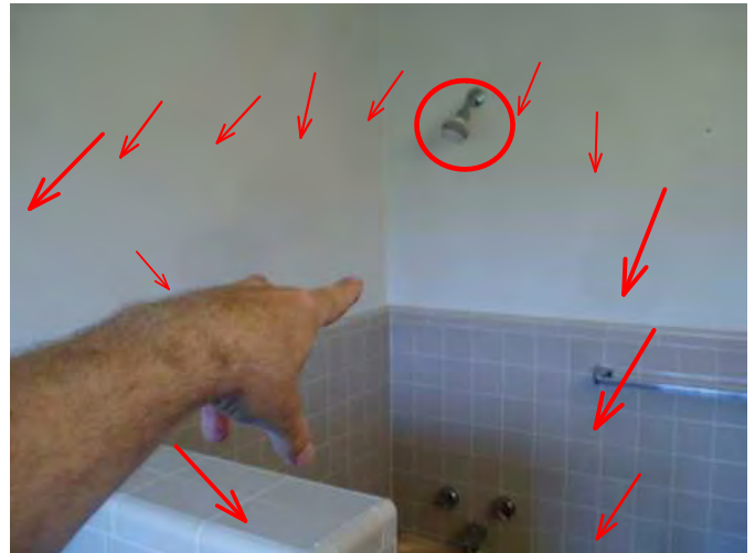
this is all wrong for wall wetness protection...needs tile to area at shower nozzle and enclosed to contain spray....
