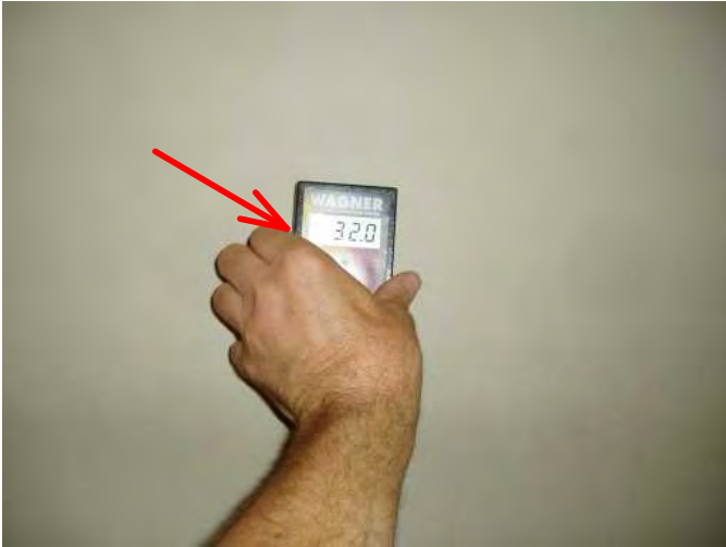
this is area at center of wall on opposite side of room where patio slopes into center..and drains into wall...
