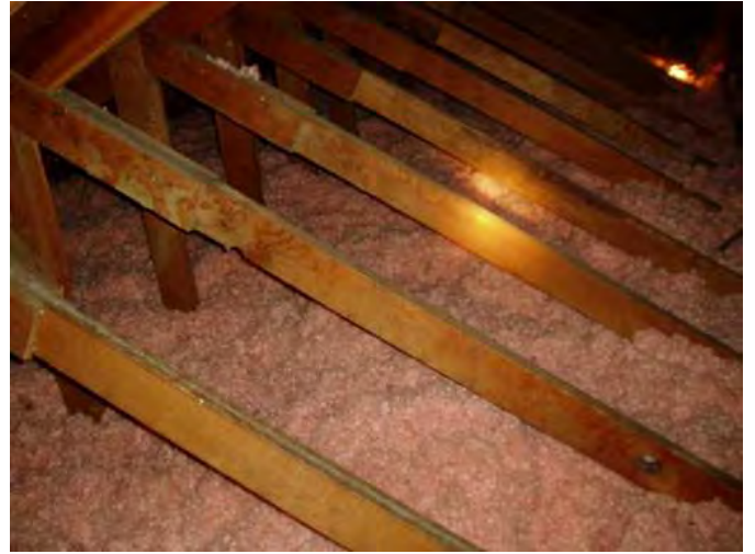
rafters are built in truss style with extra strong junctions...very good...
