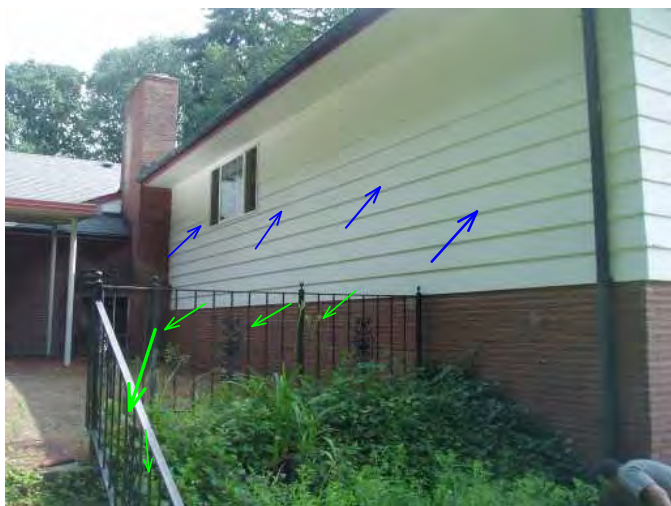
upper area is appearing solid...just needs some paint...handrails are solid....good..
