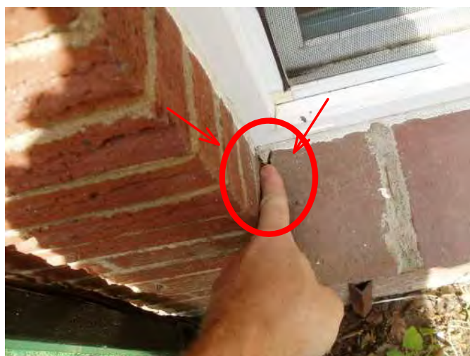
any open gaps may be added cause for high moisture in window walls noted....
