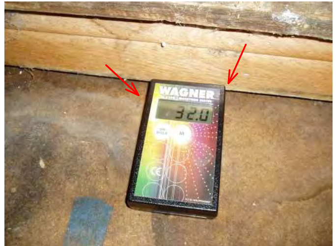
all area at cabinets at area under sink are very high moisture content...most likely wet under wood floor area at joists...
