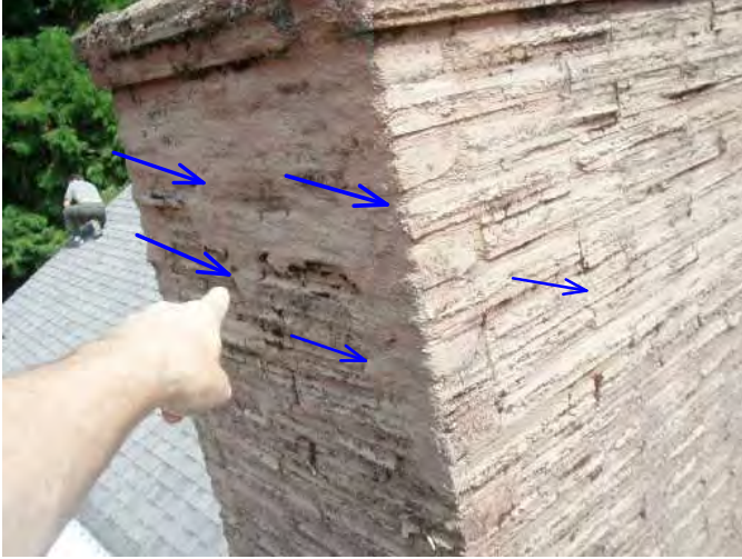
random tuck pointing needed at chimney area..not huge issue , but needs work,,,
