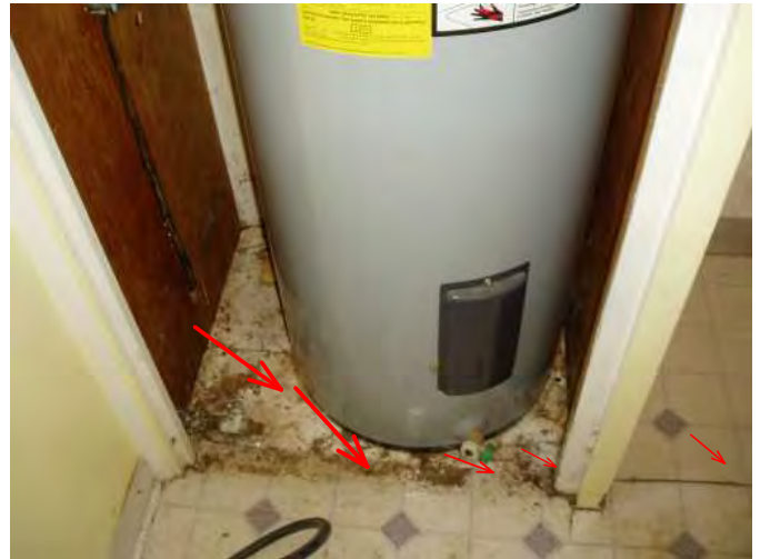
appears to be old wet area from old water heater...strap water heater...
