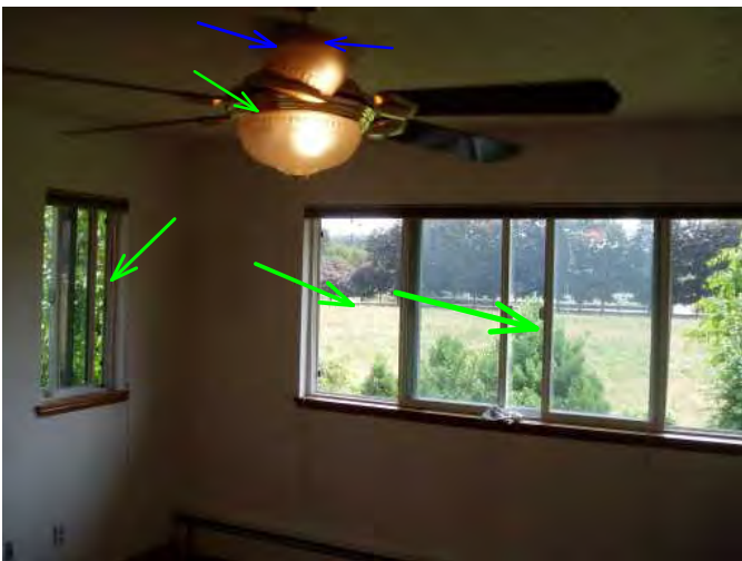
bed 2 windows and fixture and fan are operable needs trim at ceiling area..
