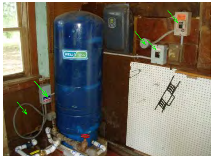
noted major cleanup of breaker boxes in pump house...very good...all cleaned out for specific use now...very good..
