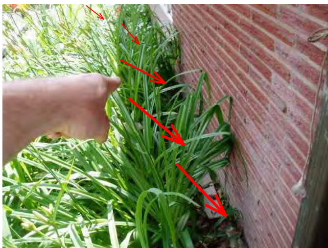
lower earth to brick contact here around planter in front of home...spalling noted...(wet brick)
