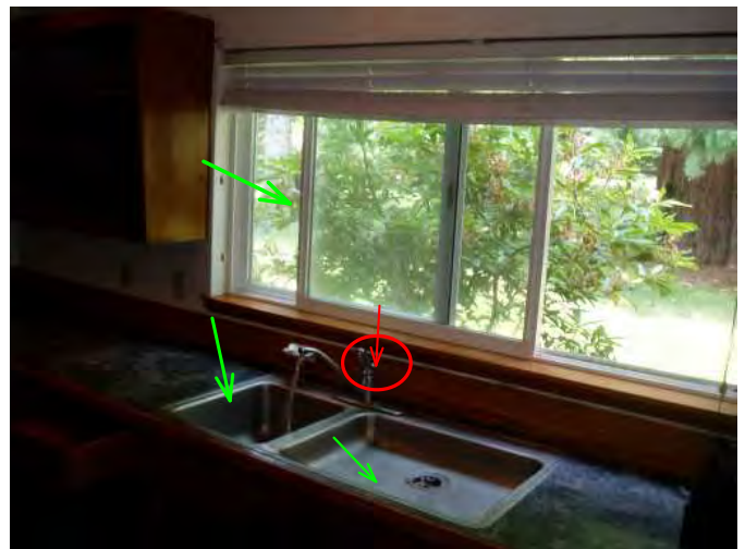
window over sink is operable...sink is operable..but faucet is reversed and on is down and off is up...really odd...
