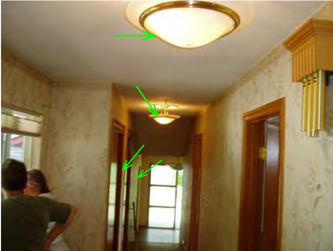
upper hall windows and fixtures and closet doors are operable...good..
