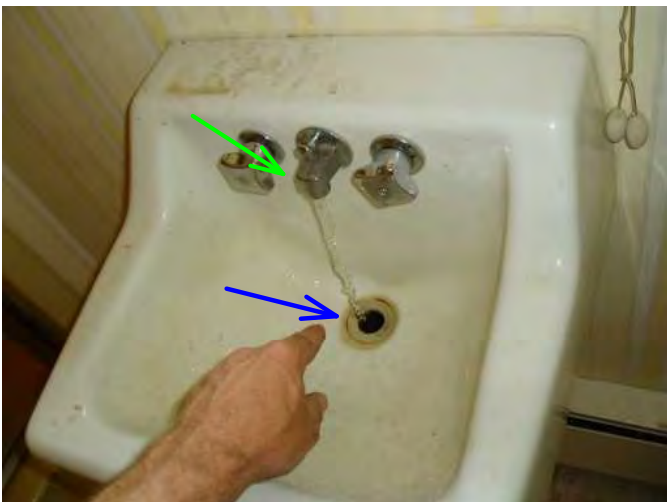
wall hung sink is operable..but needs drain stop....
