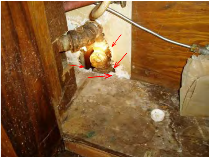
most likely vermin access entry area...seal up asap...
