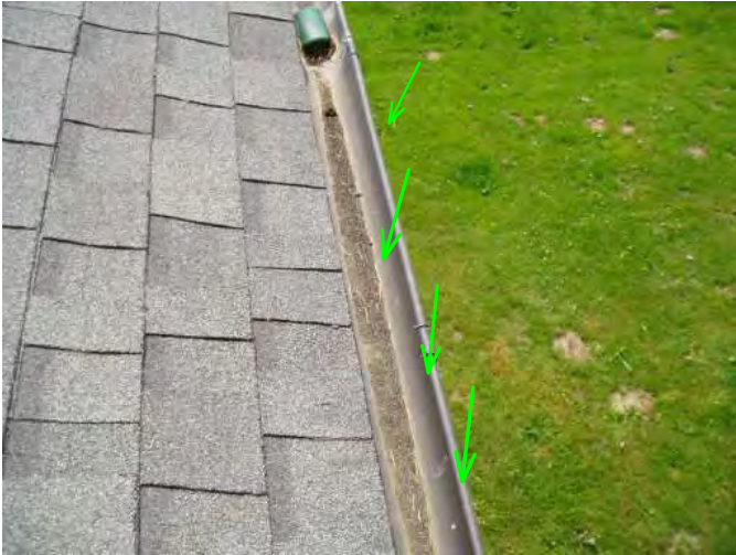
up on roof showing that not all gutters are full of debris...but this is about the only one like this...
