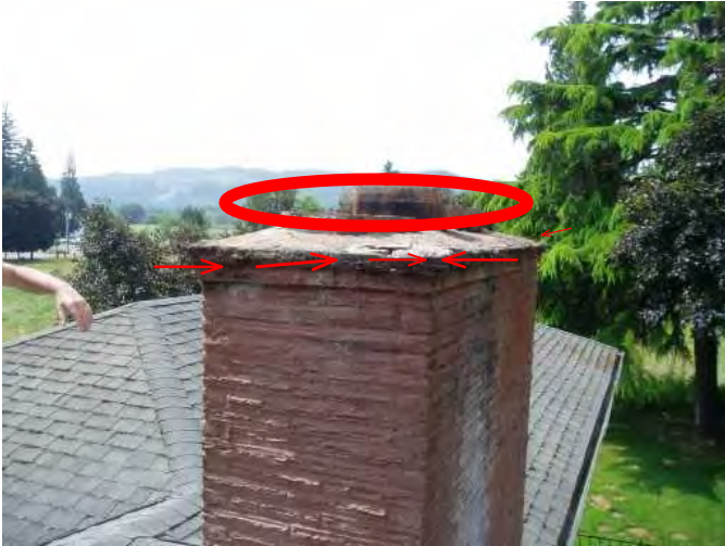
add solid rain cap with screen to keep out rain and critters...circle..arrows are pointing to needed new crown...
