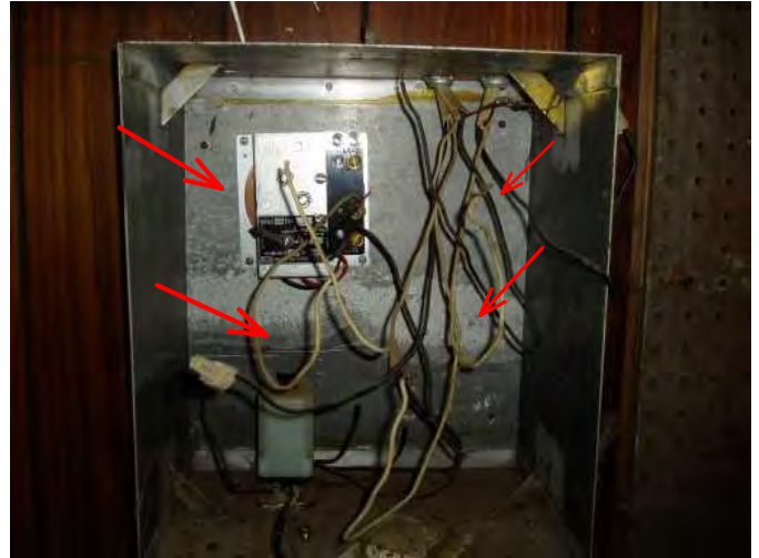
old service box is noted here in garage..not sure what to make of it..have assessed by electrician...
