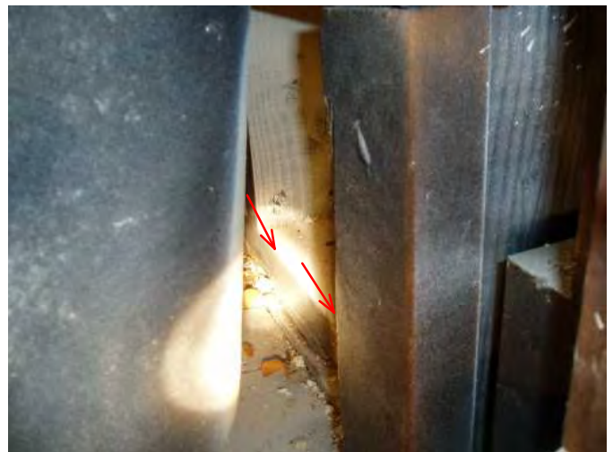
all dry....tub drain was blocked, so I did not run tub 2 hours like all other fixtures in bath and kitchen areas...
