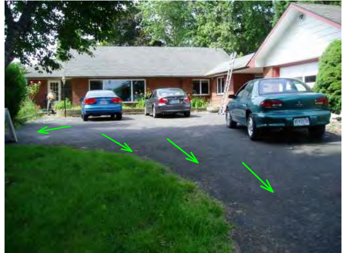
front of home has driveway that is sloped well for drainage....
