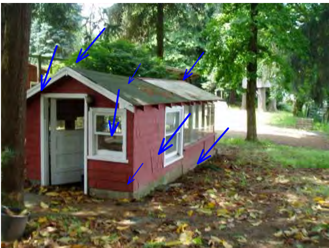
note that all outbuildings need paint and roofs cleaned and gutters and general regular maintenance....
