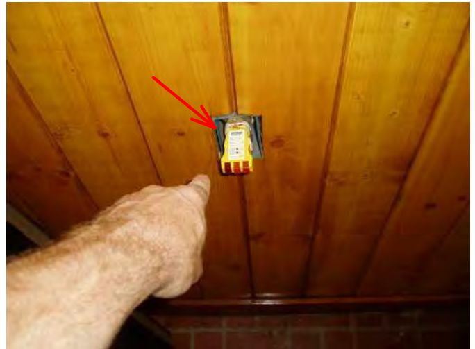
outlet in mud room is not operable...
