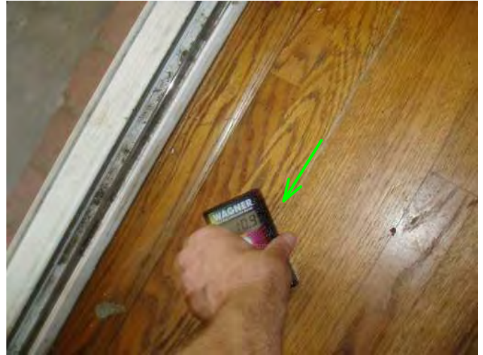
floor area at dining room slider to patio is fine...no high moisture noted....good..
