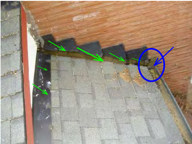
green is good step and counter flashing that are working well, blue is area that needs kickout to direct water to gutter
