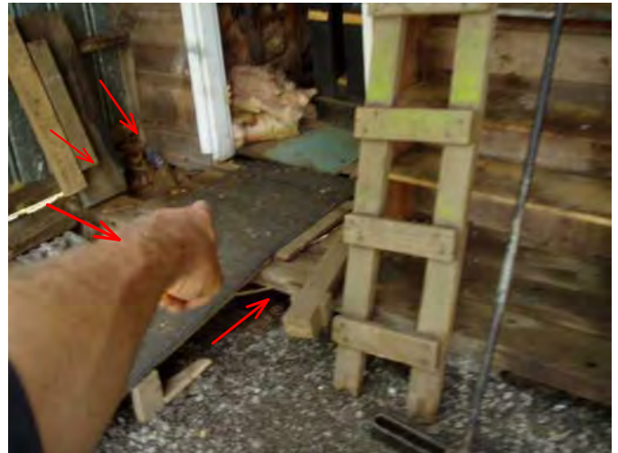
enclosed area flooring is noted here as rotting and needs repair at random....
