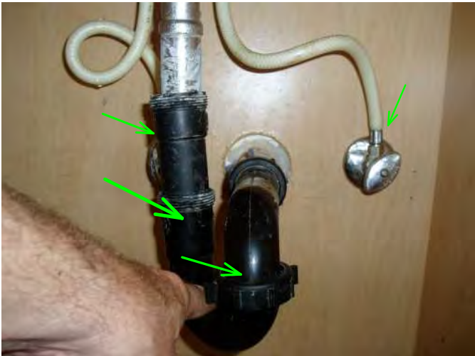
no drip sor leaks noted here under sink....good..
