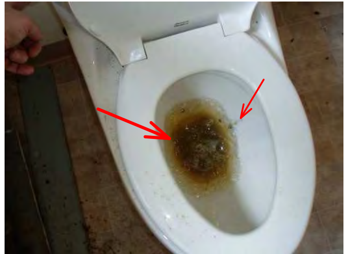
toilet is not flushing properly....repair or replace...
