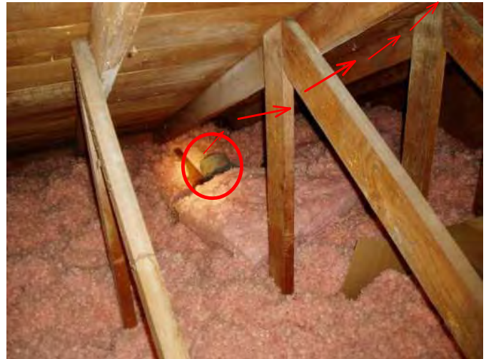
bath vent needs to be ducted to attic vent to get hot damp air out...
