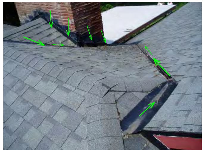
valleys and cricket here on other side of chimney are good as well...
