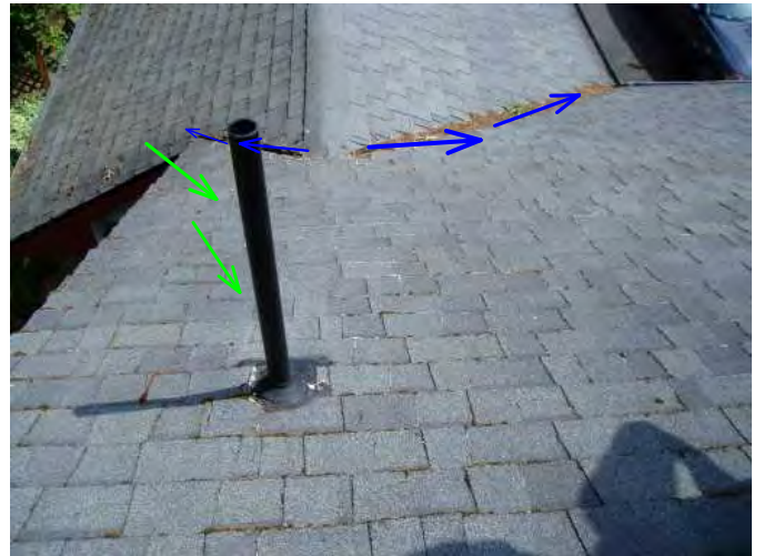
looks like abs, but is painted galvanized pipe...fine...over kitchen area....clean valleys...
