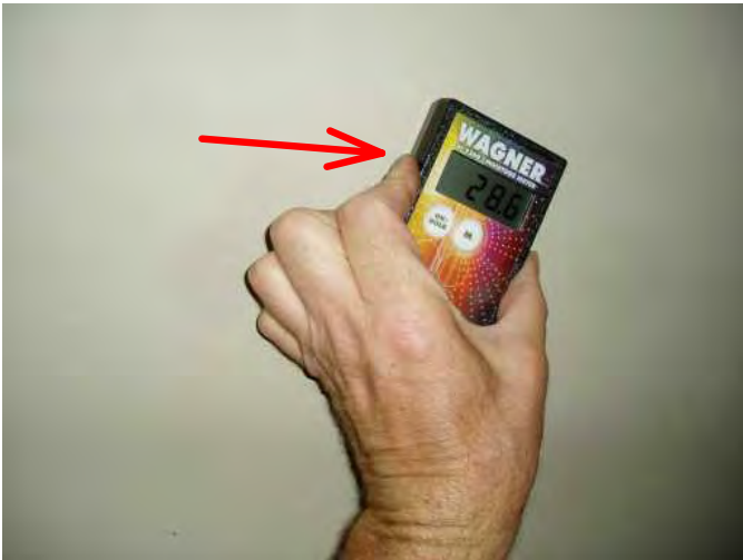
under window area in stairway is high in moisture content...will ned repairs...
