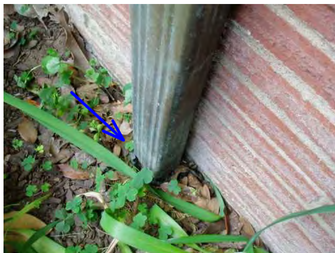
downspout at front of home under living room main window has exit to driveway...
