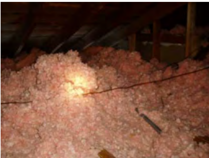
insulation is 12 inches deep...suggest adding 8 inches more for bes efficiency....
