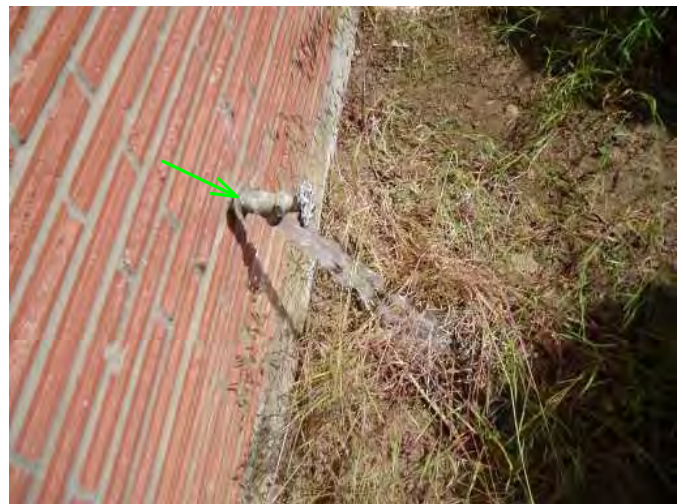
hose bib here at area works....good..
