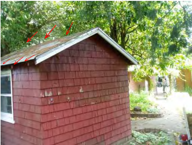
clean pump house roof and add gutters to back of roof...
