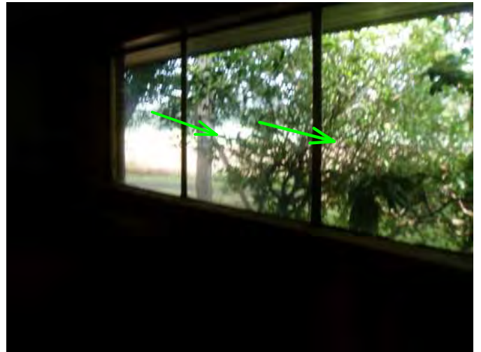
other window is operable...aluminum windows in garage noted....
