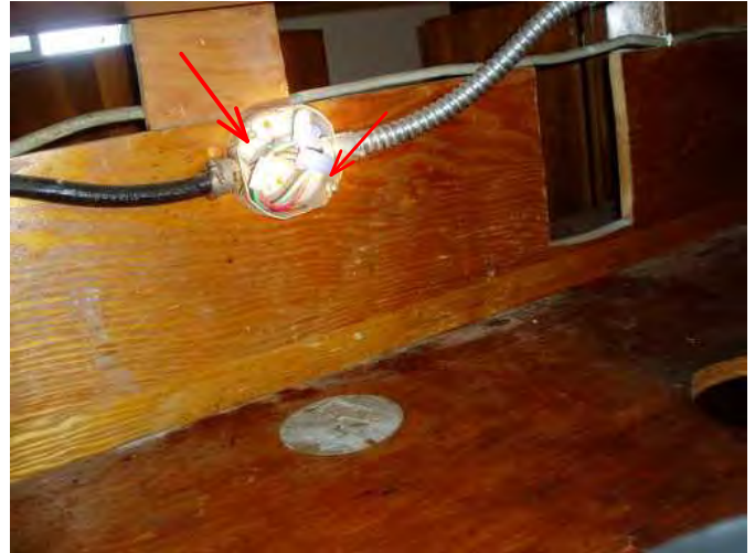
add cover plate to junction box under stove...shock hazard...
