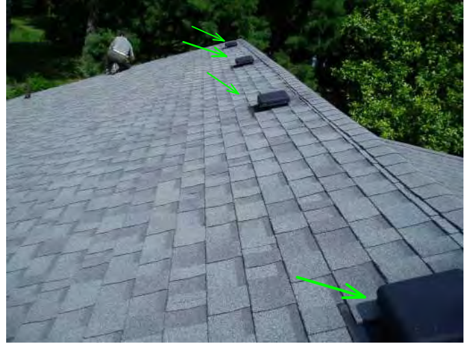
main attic roof looks good here...areas that have no moss look pretty new...areas that have moss look older...
