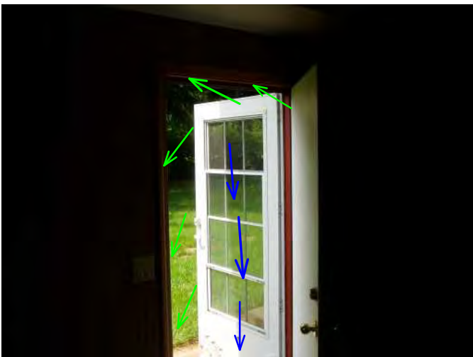
exit door is operable..weather stripping is good...storm door needs work...
