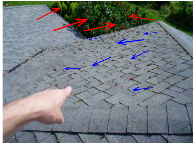
ditto here over front porch area...also noted heavy vegetation needs to be cut back to see home...(maintain)
