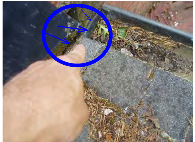
kickouts go over gutter area and deliver water into gutter and not behind siding...
