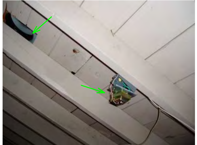
attic is well vented and low voltage door bell converter is noted here in attic for front door...
