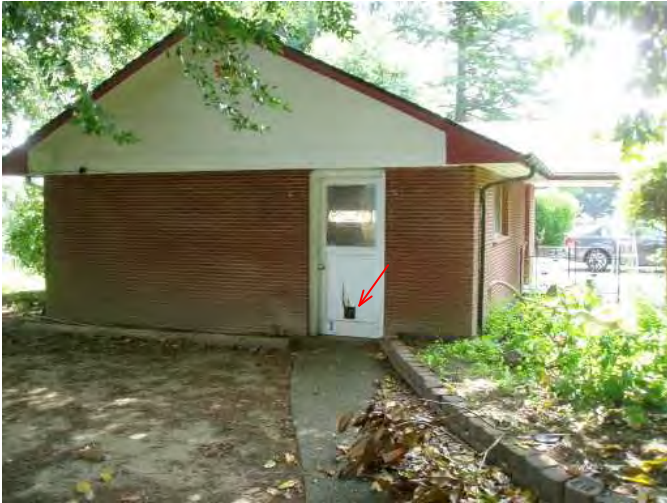
both garage doors are in poor condition...may need replaced....rest of structure is in pretty good shape...
