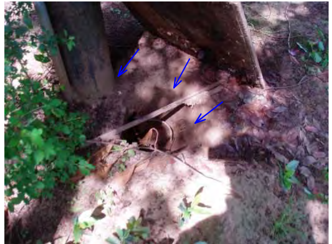
appears newer hole is here..pole is full of rot...will need replacement...
