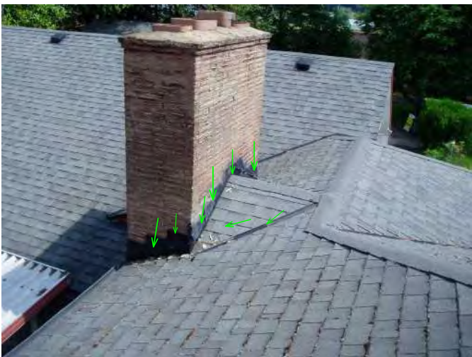
cricket and valleys around chimney are good...
