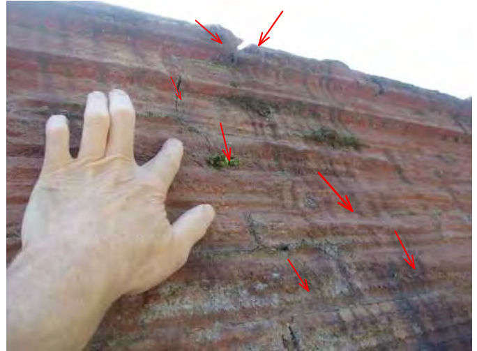
old crown is showing leaks that are staining chimney here at back over patio fireplace...
