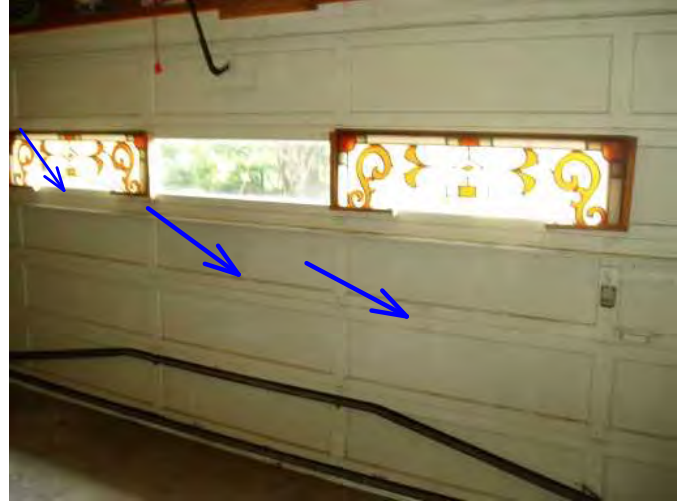
garage door is operable...but is not attached to opener...and is very heavy to operate, have repaired by door specialist
