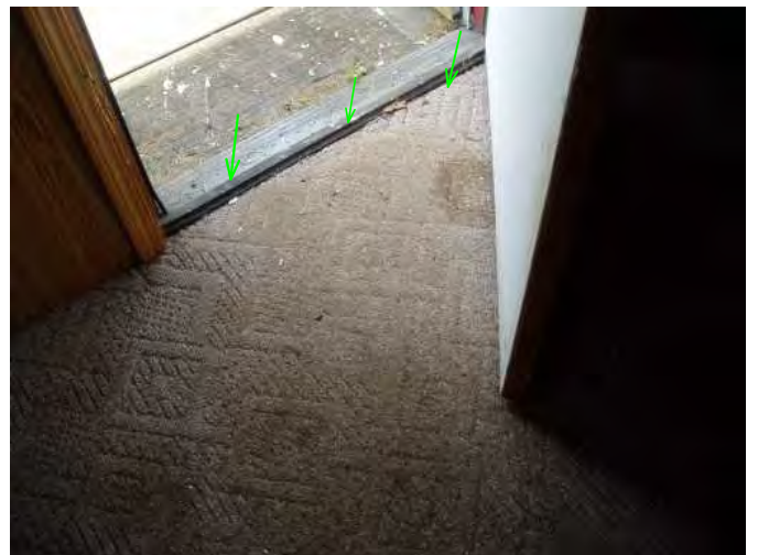
threshold is solid and sound...exit door at bed 3.....good..
