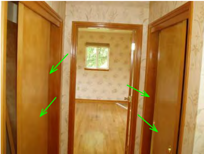
upper hallway closet doors are operable...just needs some lower tracks installed....
