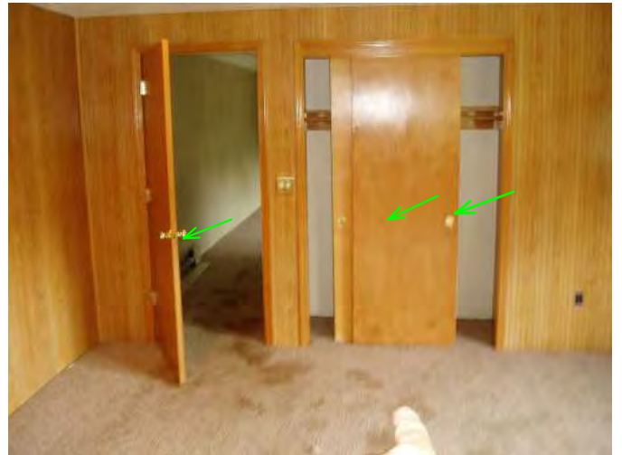
bed 3 in basement entry and closet doors are operable...good..
