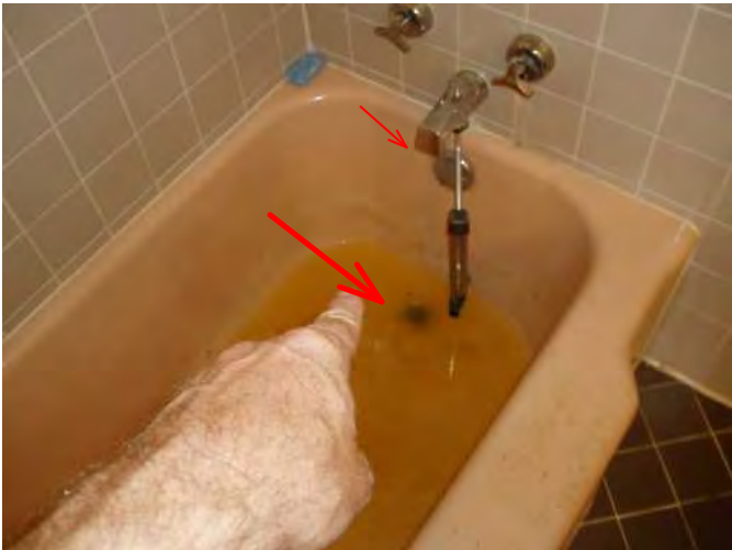
tub is blocked at drain..did not run like all others....may leak as well..not sure....
