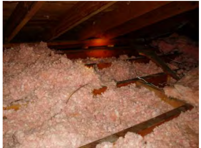
upper attic over kitchen area, has double wide ceiling joists noted for extra strength...good..
