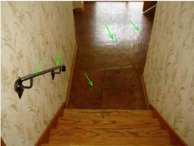
handrails are solid and entry floor is solid as well...
