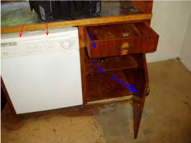
dishwasher is operable...but needs to be attached to counter...cabinets are operable..but need work...
