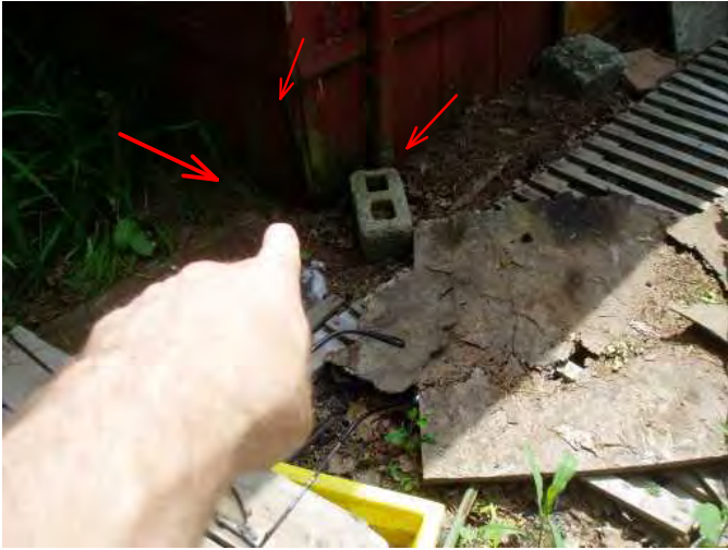
this is where downspout was and now is rotted wood area....chicken coop back area....maintain roofs...
