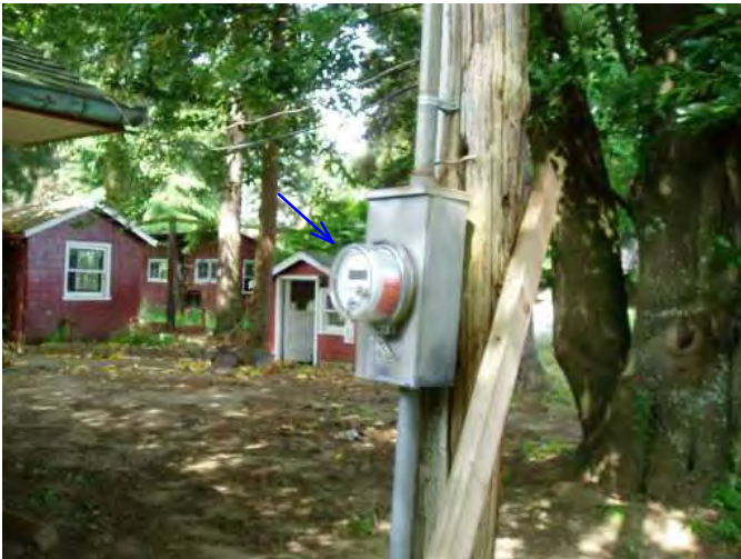
main electric is overhead and then enters into lateral service...appears to be newer meter...
