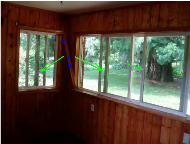
windows are operable in mud room here as well....needs trim repair...
