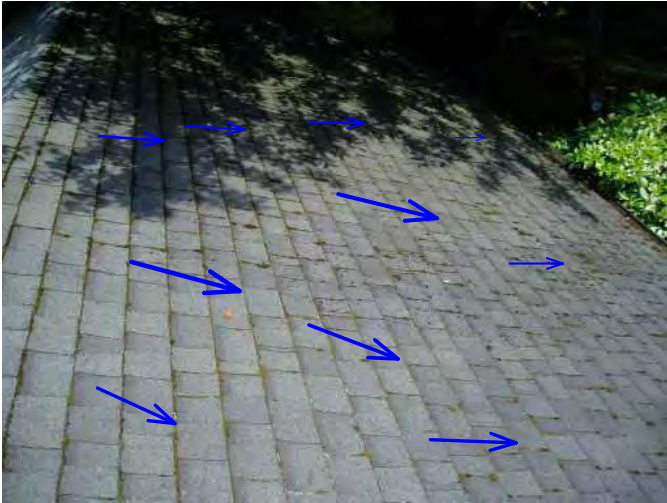
area over garage to right of front upper roof...trim back tree branches 6-12 feet above roof line...clean and de moss....
