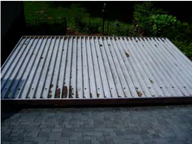
metal awning roof over patio needs cleaning..and is in good condition....good..
