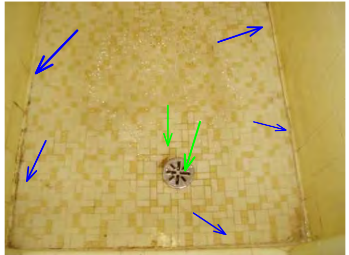
drain is operable...but ceramic tile needs grout work....
