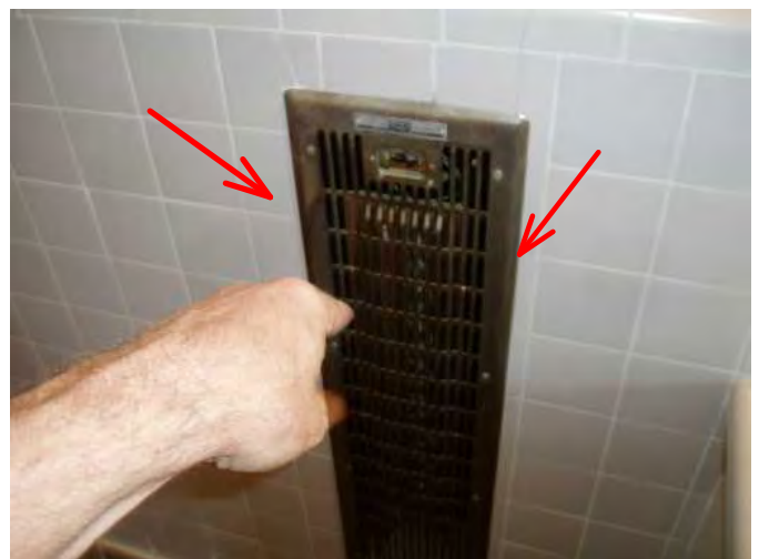
main breaker was shut off for this unit...did not turn on...may be a reason...
