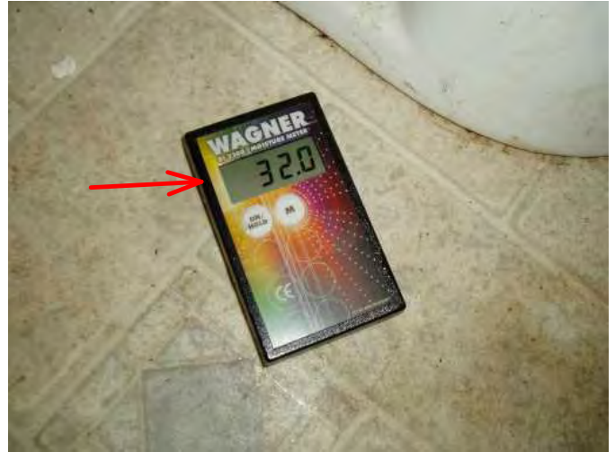
here at front of toilet is same...very high content noted....repair or replace flooring...
