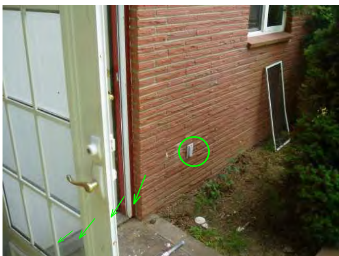
outlet at door by bed 3 exit is GFCI and is operable...porch area is sloped well and door threshold is raised...good..
