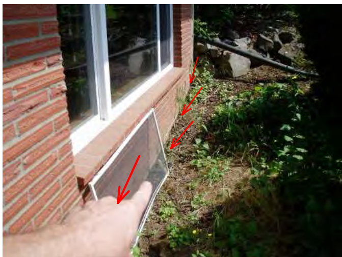
earth to brick is not good, no weep holes noted at base..not good...vapor has no way to exit
