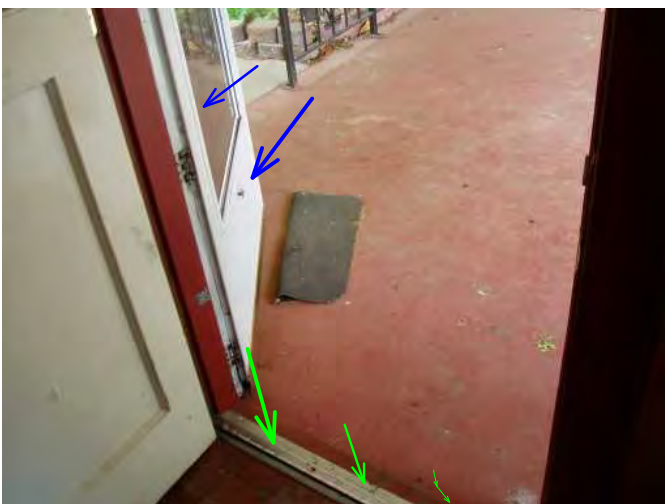
storm door is needing a bit of work to latch...threshold for mud room door is solid....good..
