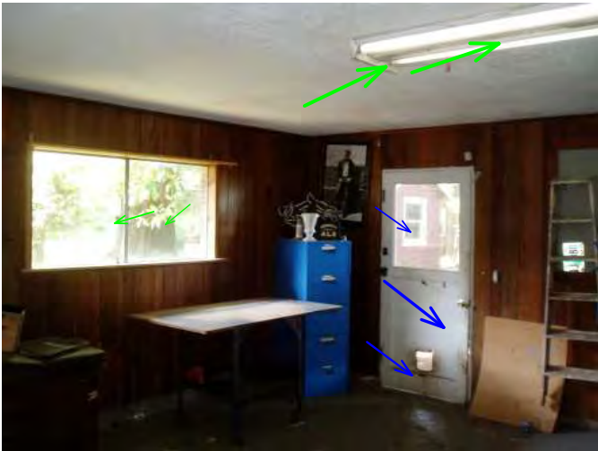
window and fixture are operable...door needs work...
