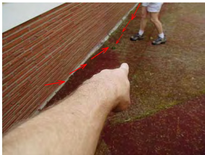
slope at patio is not good for lower area in basement room...suggest adding surface drain or curb to exit water...
