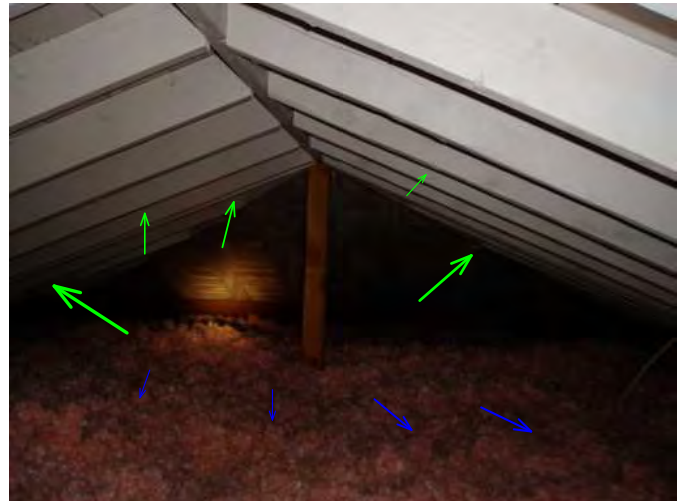
upper rafters are fine..painted from old fire some time ago...insulation could be 8 inches deeper for best efficiency...
