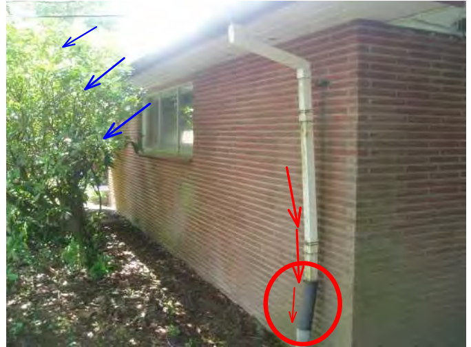
remove or pull back vegetation and not sure where this exit drain exits to...
