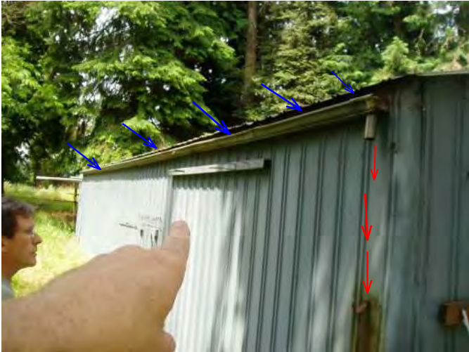
gutter at back of pole shed needs to be operable and cleaned regular...add downspout and extension...
