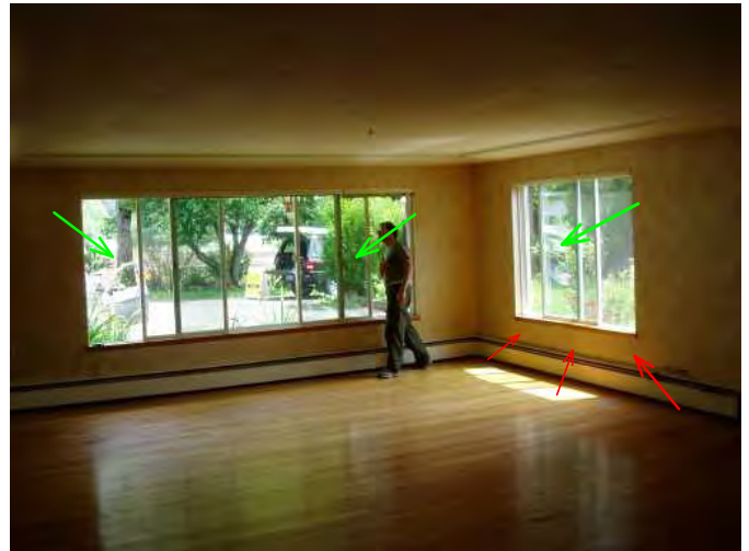
living room windows are operable...found high moisture in lower area of right window...
