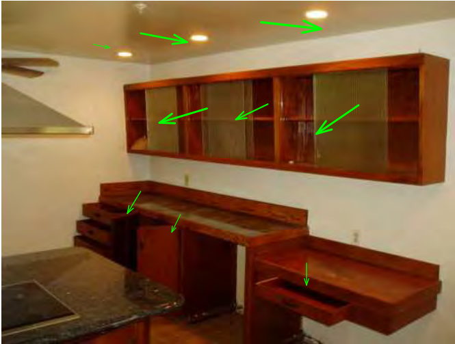
fixtures and cabinets are operable in area...good..
