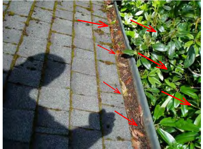
realy full gutters and trim back shrubs 12 18 inches from structure...
