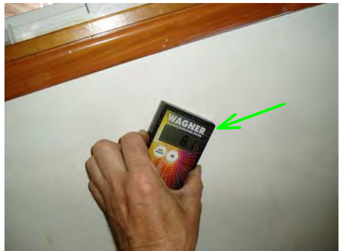
no high moisture is noted in area under dining area window...good..
