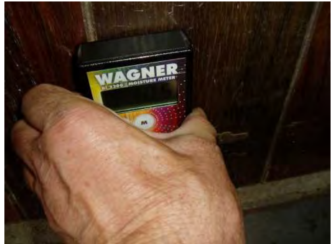
no high moisture in garage walls noted....good,..
