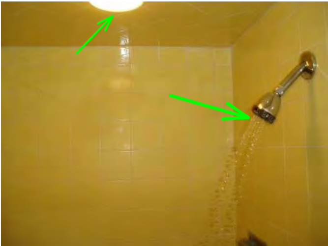
shower fixture and shower head are operable...
