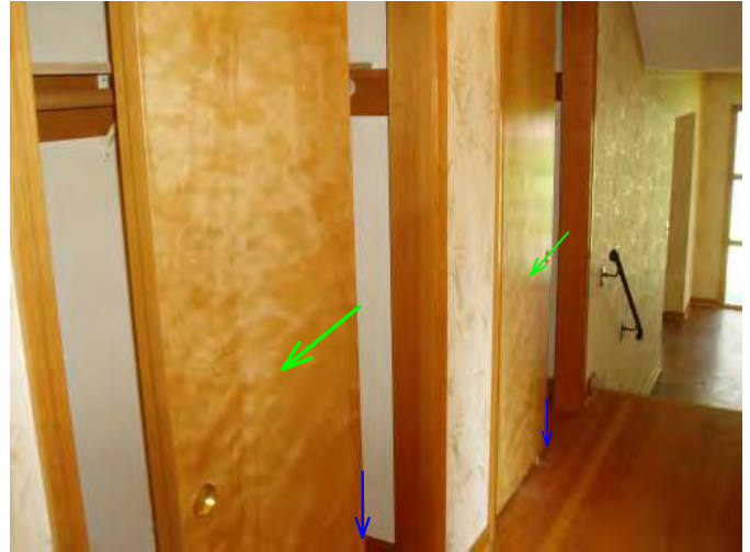
left closet doors need tracks like right one has...
