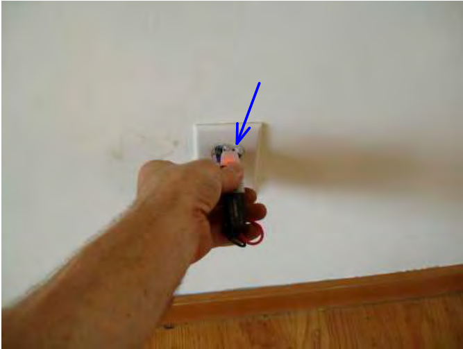
bed 2 outlets are not grounded....is common find in older homes...
