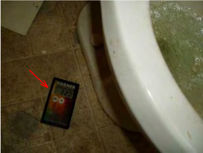
toilet is operable...but floor around toilet is very high moisture content noted....
