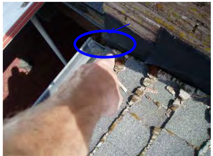
needs better kick out here as well...just stops and does not direct water into gutters...
