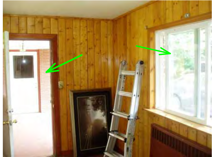
window and door in muc room are operable...
