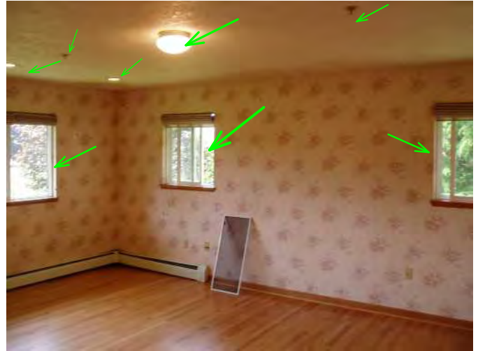
master bedroom windows and fixtures are operable..all of home has sprinkler system installed ....good..
