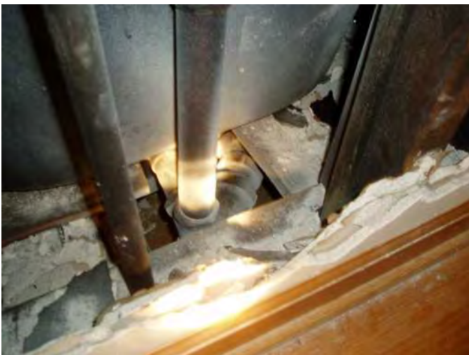
did acces into area to see if any leaks were noted...none found..but also tub drain was blocked
