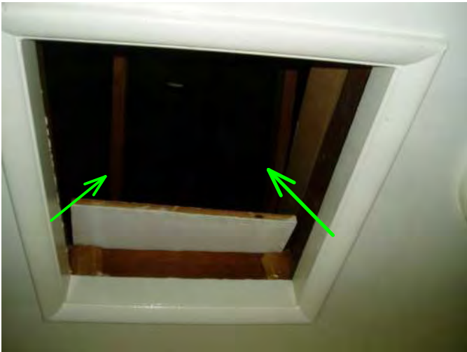
attic access to lower attic over main home area....access in laundry room area....
