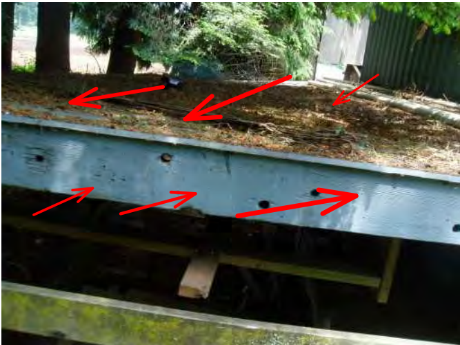
clean all roofs of outbuildings often...keep al wood trim painted to extend useful life....
