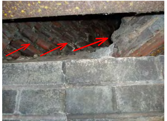
no damper noted...add top cap damper for best results...
