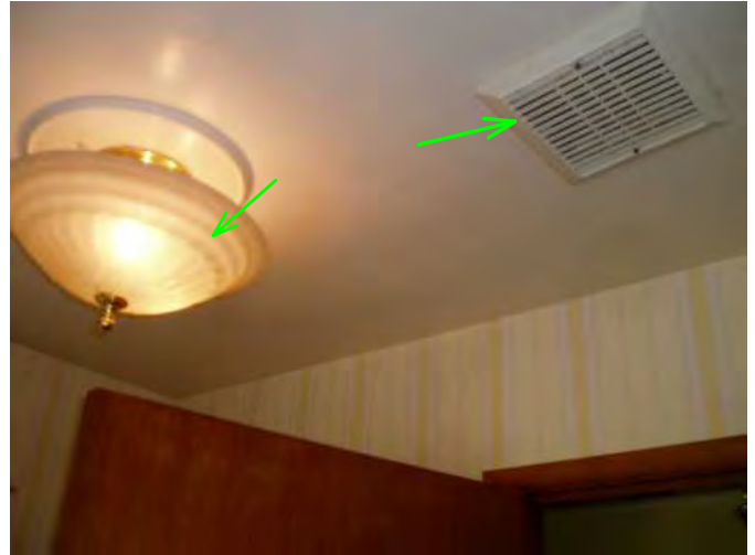
back bathrom fixture and exit vent are operable...
