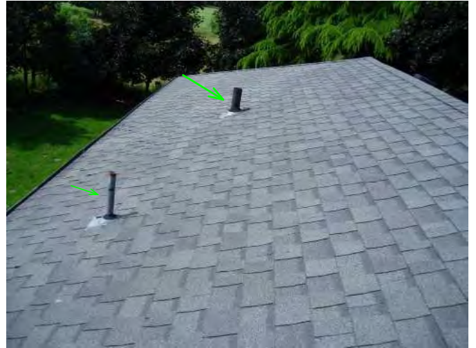
back area over upper bedrooms showing sewer vents in roof are solid...sleeves are good...roof fairly clean here...good..
