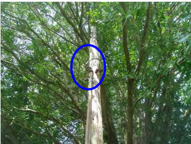
drip loops are fine...but service from street is impeded by tre branches....
