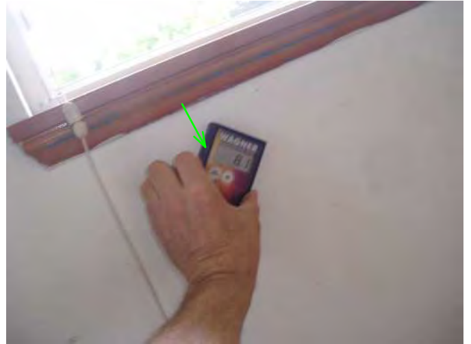
noted low moisture at bed 2 under windows....good...
