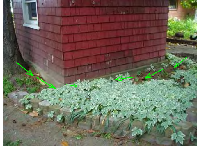
good foundation note here at pump house...
