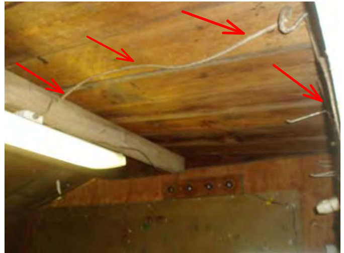
add any wiring into conduit...for shock safety...
