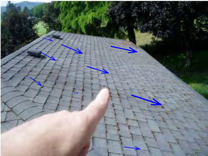
other side (back) of roof needs cleaned and de mossed...
