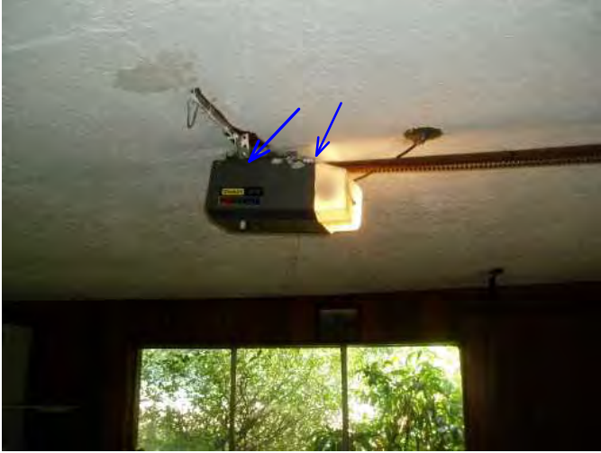
garage door is operable...but needs new wall switch and needs repair to attach to door...
