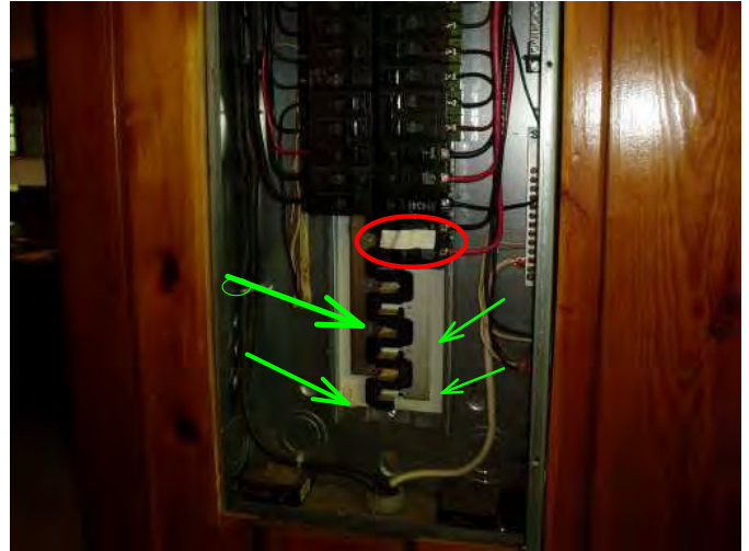
remove tape and identify breaker or remove breaker...after upsizing service, you will have lots of room for growth...
