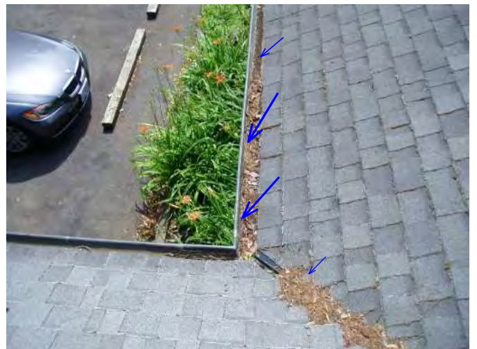
more full gutters mean leaks into home....clean gutters often...
