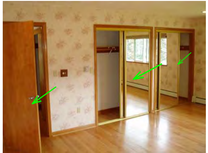
master entry and closet doors are operable...good...
