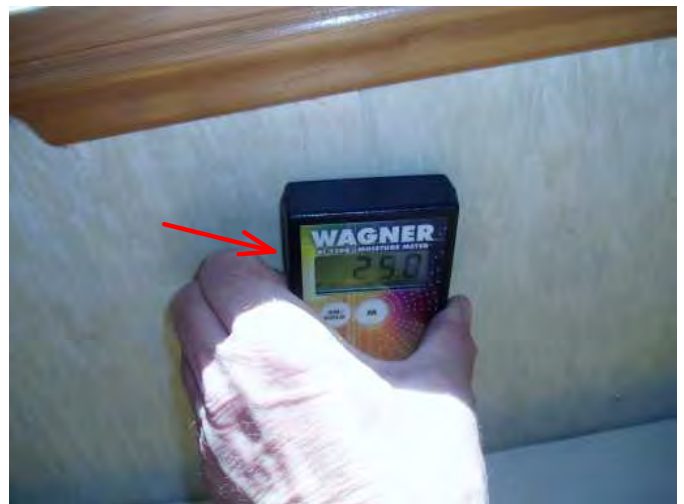
area udner window is noted here as high and needs assessed....
