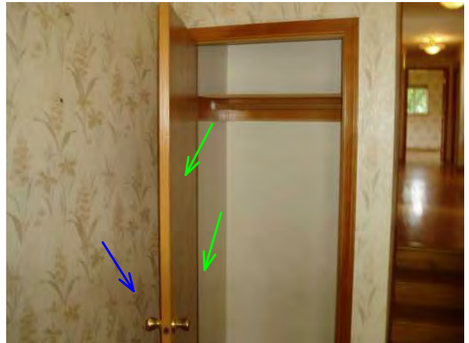
entry hall closet door is operable..but needs door stop...
