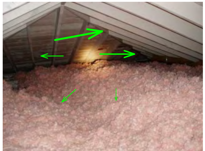
roo fover bedrooms is hip type...rafters are solid and sound....good...painted after fire in past...
