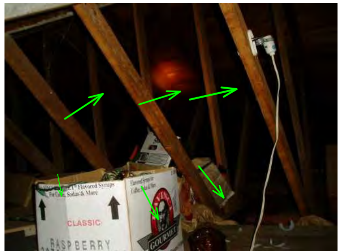
upper attic over garage is noted with flooring for storage.....good..
