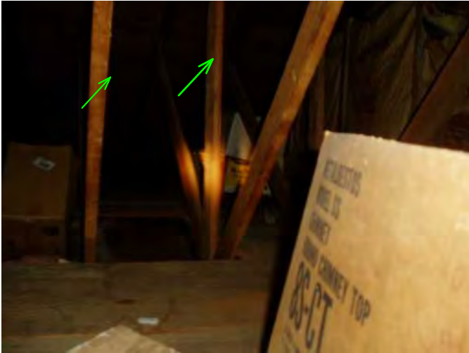
2 x 6 rafters and 2 x 4 truss supports noted in attic...good..no staining on sheathing noted...good..
