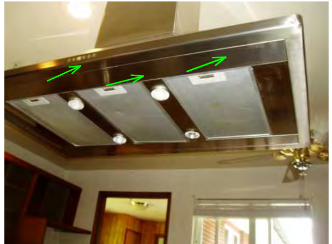
over stove hood is operable and is solid to ceiling...good..
