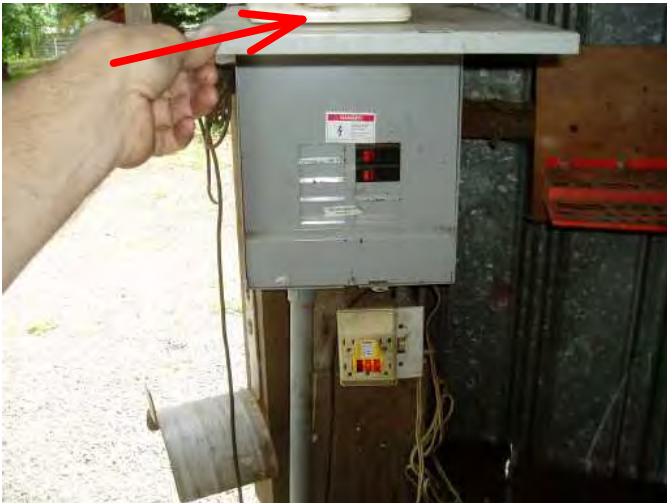
mini breaker panel at pole shed is noted here....sugest removing hand sanitizer from cover....
