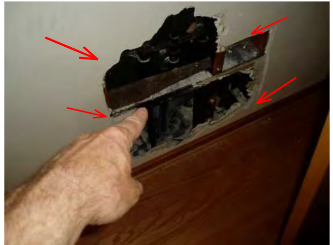
large hole in closet was found..not in home before...not sure why..no leaks noted...
