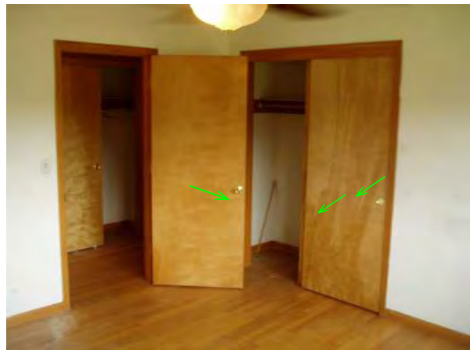
bed 2 entry and closet doors are operable...good..
