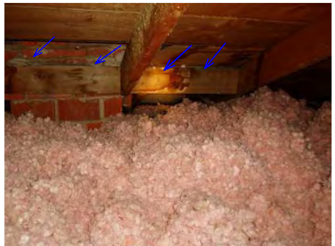
old inactive staining noted here over chimney in main attic from past...most likley why newer roof is on now...
