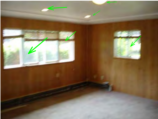
basement bedroom windows and fixtures are operable...noted random missing screens needed....
