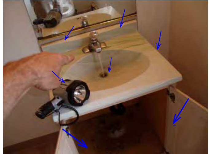
this counter is installed over old counter..and cabinet is showing lots of moisture issues...replace...
