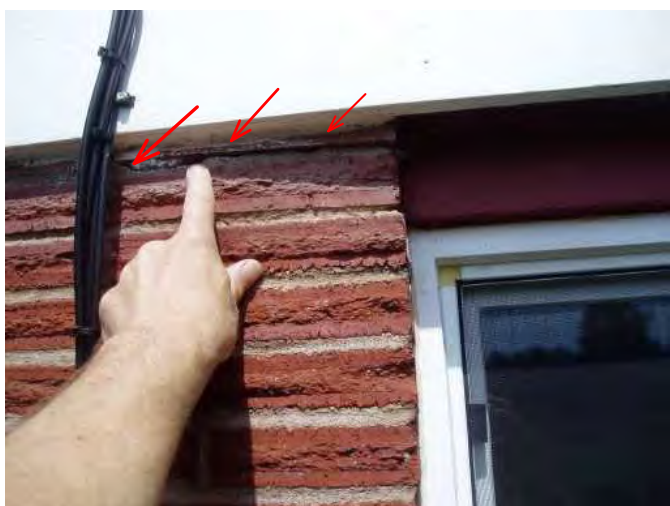
noted upper area of brick around window that has high moisture under window area is open here...re-seal...
