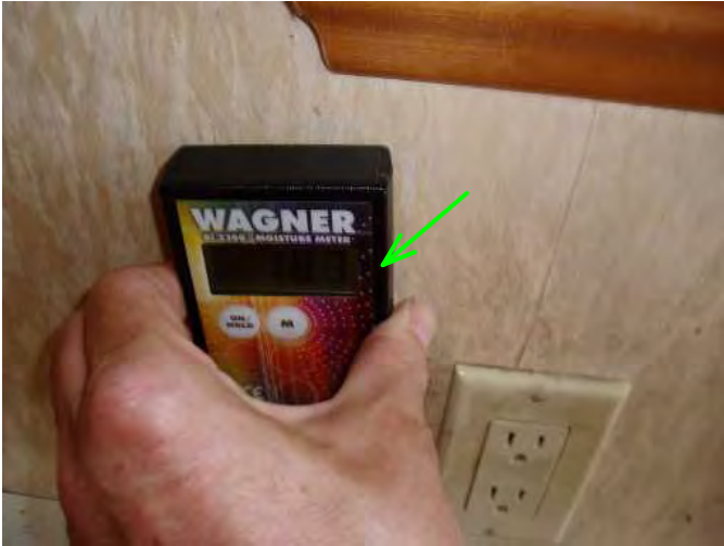
area under left main window is fine....good..
