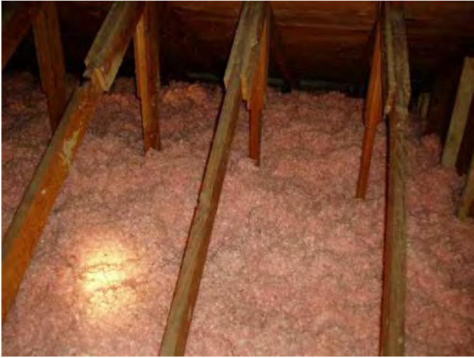
strength is noted all through out attic area...good..
