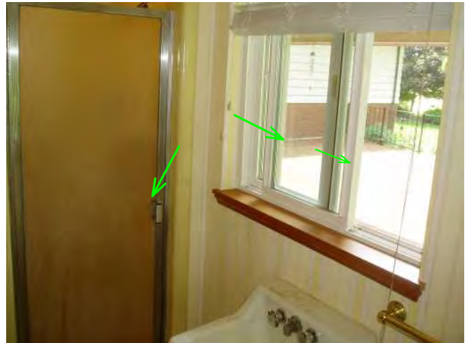
shower door and window at side of bath are operable...
