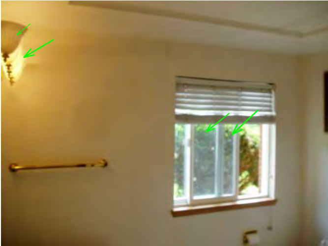
windows, fixture and entry door are operable in basement bath....good..
