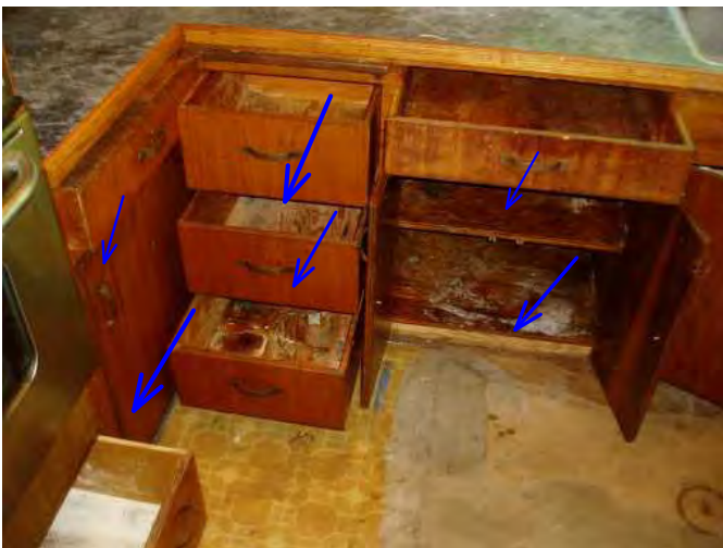
lower cabinets in kitchen area are full of debris and hoted vermin droppings...
