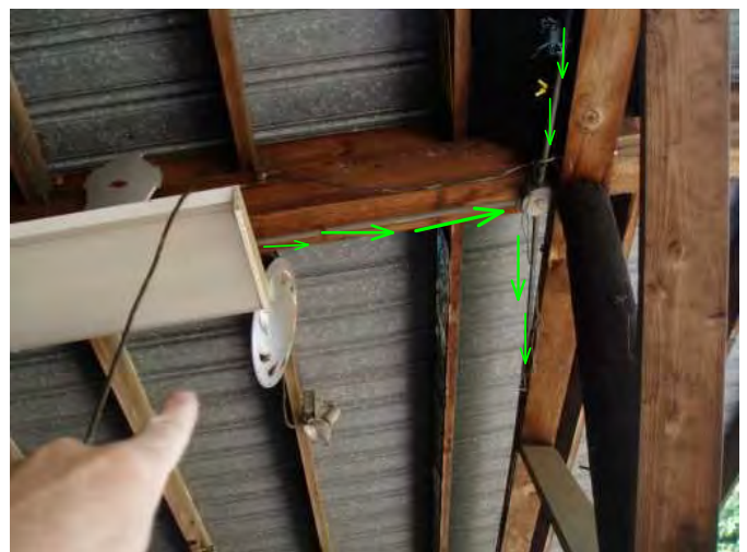
conduit is noted here...good..
