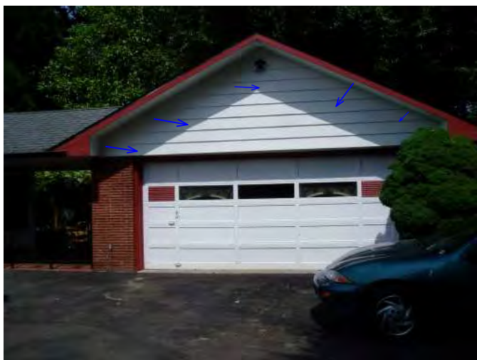
front of garage is noted here and lights are operable...siding just needs a paint job...garage door is not operable yet...
