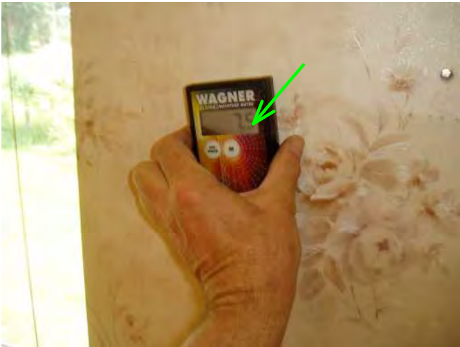
checking all exterior walls for moisture...good here in master...
