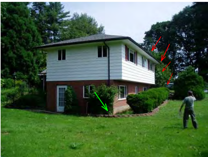
all other downspouts are connected to exits...good..upper siding needs to be painted..trim back all vegetation from home
