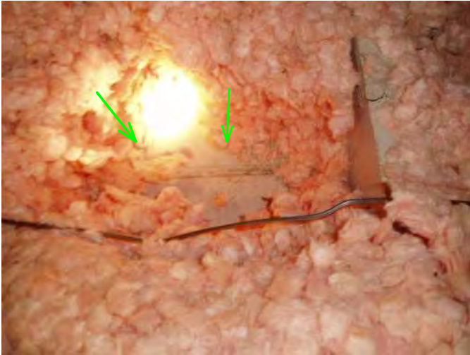
drywall under insulation noted here....good..
