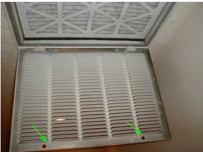
upper furnace filter and return air vent cover...two easy twist screws to open and change...
