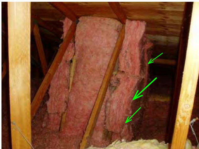
back bathroom skylight is wrapped...good..keeps moisture from accumulating...
