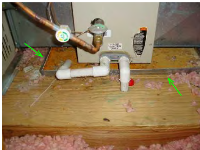
this is drip pan that feeds to outdoors...good...
