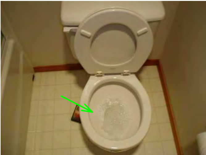
toilet flushed well...no flow changes in shower were noted when flushed...
