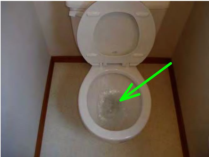
toilet is operable...no flow change noted at shower when flushed...
