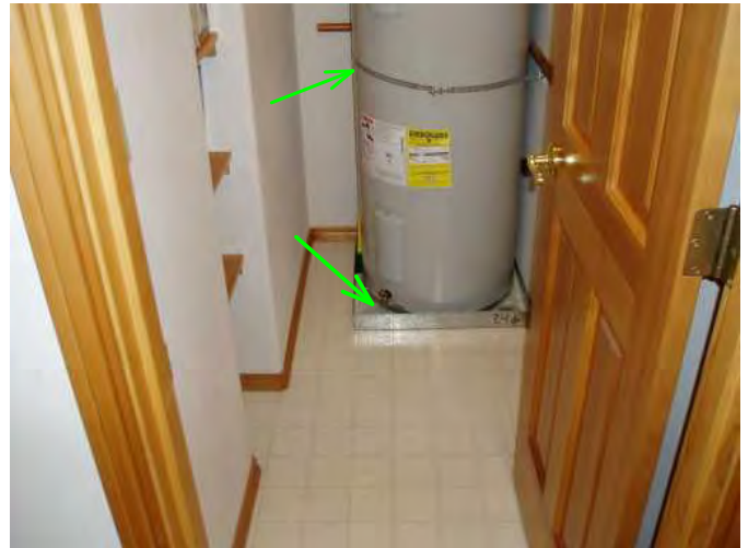
water heater is strapped and in drip pan...good...
