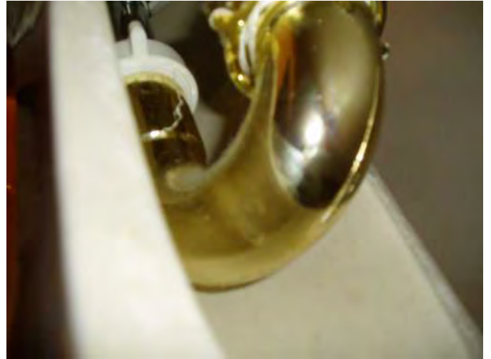
no drips at trap under pedestal sink is noted...good..
