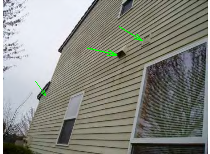
venting or kitchen, bath on first floor and laundry are noted here....good...
