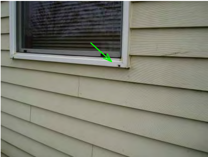
all windows have weep holes in proper place...good...just be sure and clean windows sills inside once a year...
