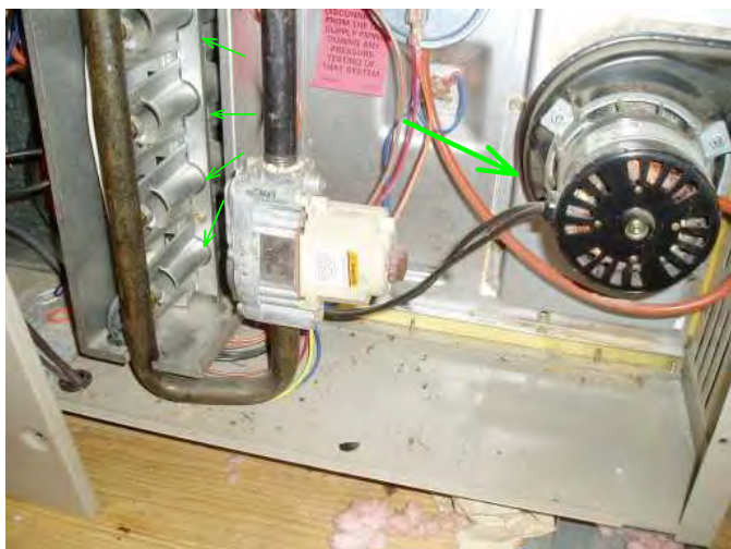
4 burner system is operational...in furnace...good...has draft inducer...good..
