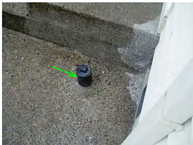
sewer cleanout is at back patio ...good...
