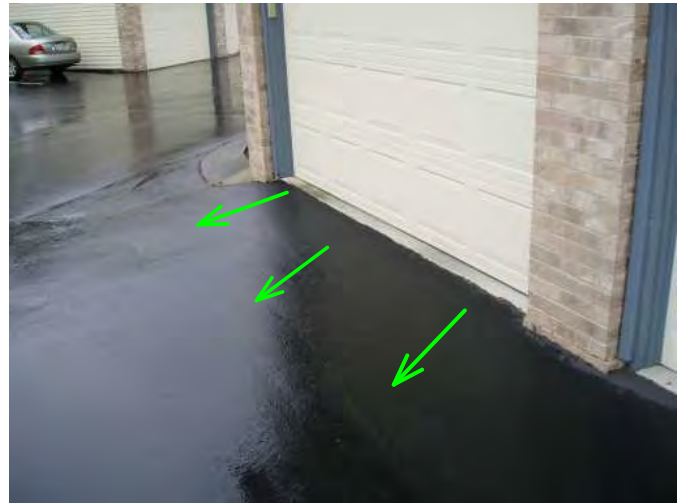
garage has good slope at door for water drainage...
