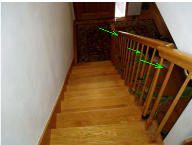
lower handrails are solid and steps are even to first floor...
