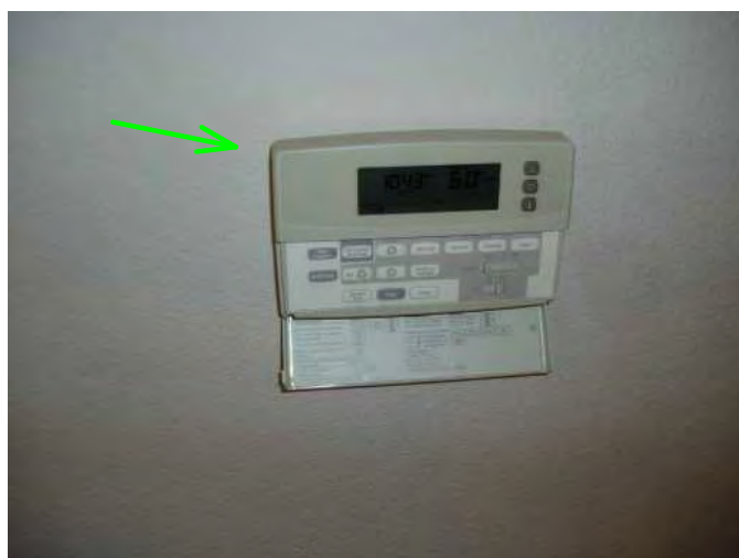
thermostat is operable..on first floor by bathroom...
