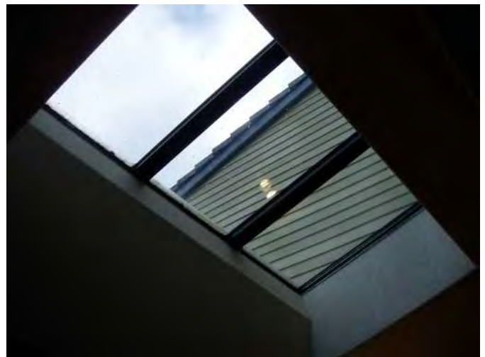
skylight is operable...no staining noted at walls...
