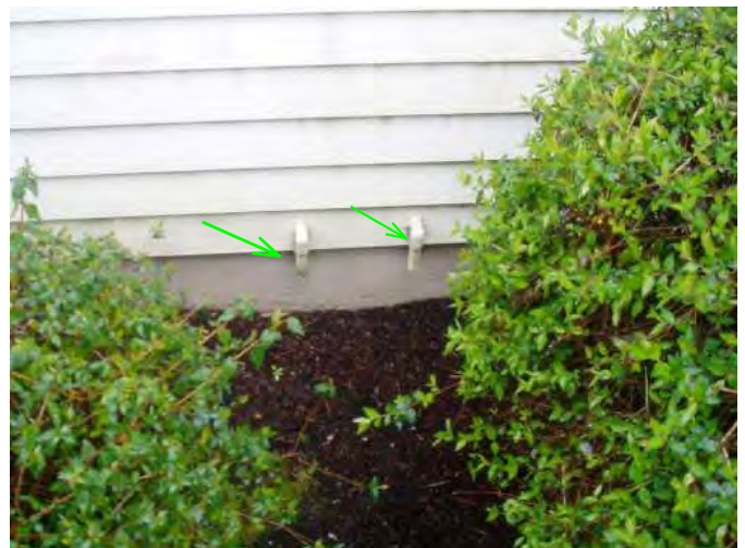
these are for drainage from attic furnace...good..side of exterior of home...
