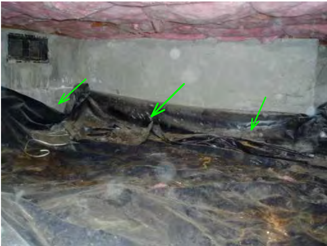
vapor barrier is on all areas of crawl space...good...
