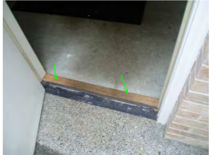
garage entry door is weather stripped and threshold is solid...good..
