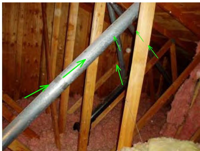
up in attic showing venting to roof from bathrooms...good..
