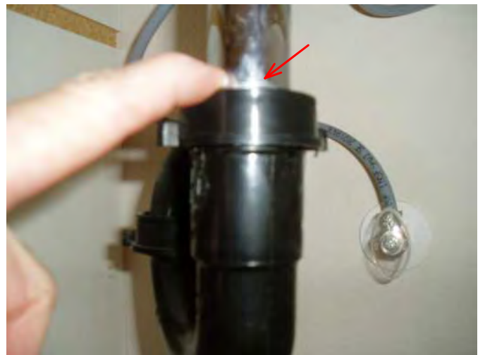
smal leak noted at trap...run all faucets for 2 hours to detect any future issues..here is one...
