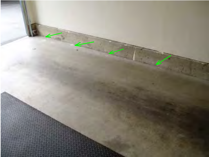
garage has good slope for drainage to outside...good..
