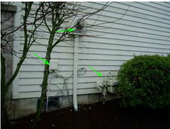
phone, electric meter and gas entry are all noted here at side back area of home...all good...
