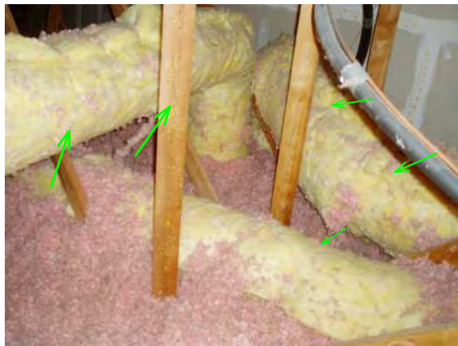
all ducts are insulated in attic....good...
