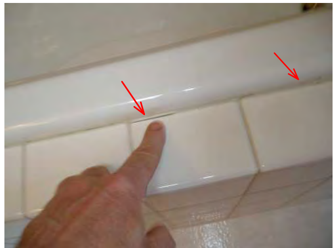
minor grout repairs needed to keep out water at joints noted...
