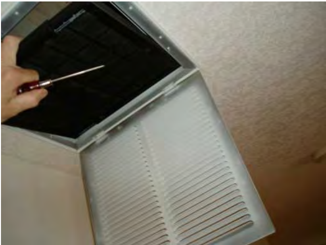
this retrun air has re-usable filter...good..
