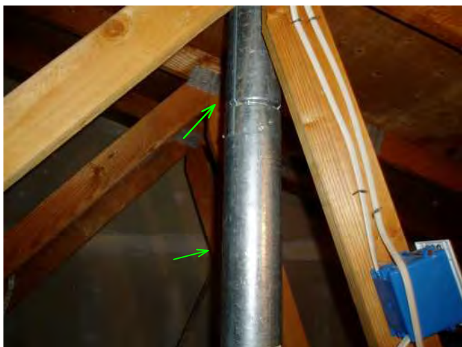
furnace flu in attic is solid and no staining is noted at roof line...good..
