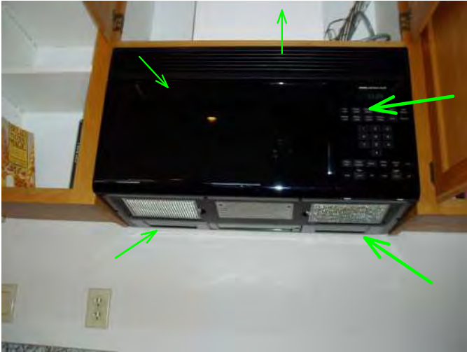
microwave and over stove exit fan are operable...and vented to outdoors...good...
