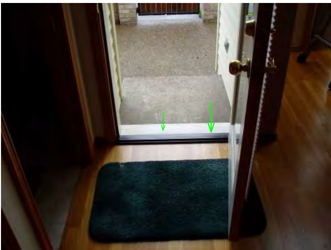
threshold is solid and no moisture issues noted...
