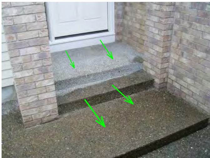
entry stoop is sloped well for drainage...good..
