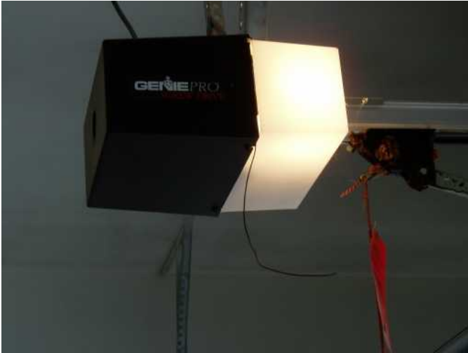
garage door operation is fine....
