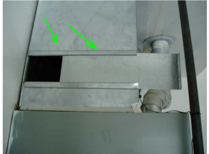
furnace filter is accessible on upper side access slider cover....
