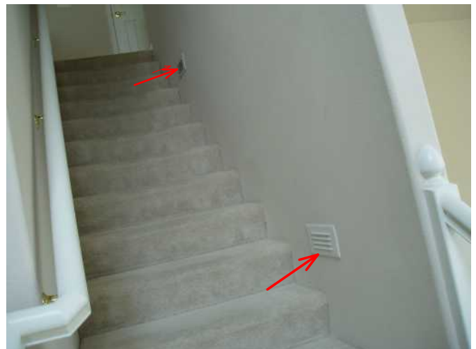
stair safety lights works fine....
