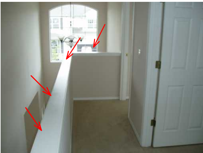
hallway railing to bed 3 is solid and sound...
