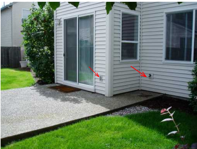
back patio has good slope/ electrical outlet works fine/ hose bib works fine as well...has backflow protection...
