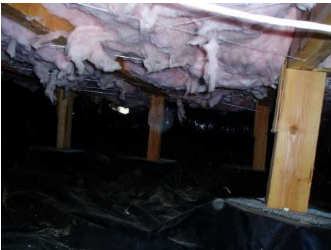
post and beam system in crawl space means a very well built home...sub floors are plank diagonal tongue and groove...
