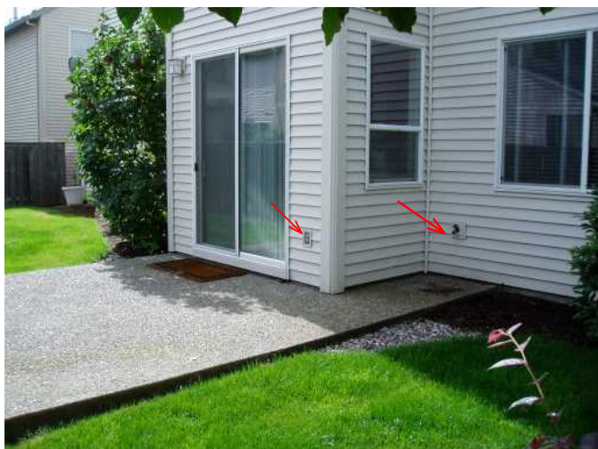
back patio has good slope/ electical outlet works fine/ hose bib works fine as well....has backflow protection...
