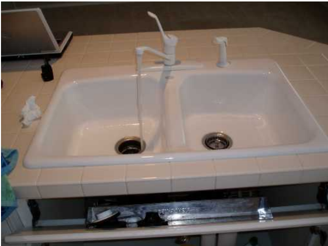
did flow test at kitchen sink and ran dishwasher through complete long cycle..all good no leaks noted...faucet is good.
