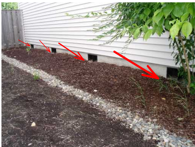
vents to crawl...do not add any more barkdust...will cause water entry to crawl...keep even or below...
