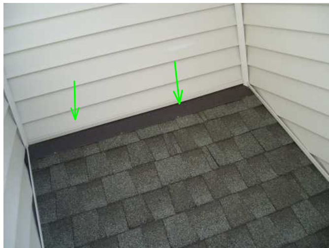
very good flashing here as well in front of main bathroom...
