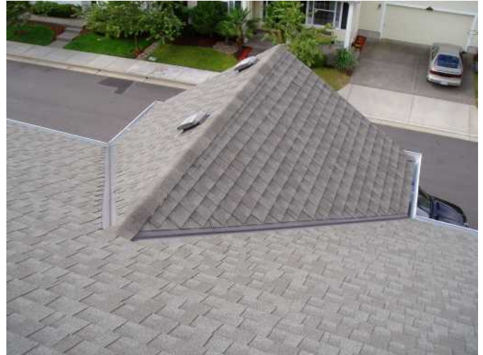
front of roof is vented well ...valley are good...gutters are clean...monitor season to season...
