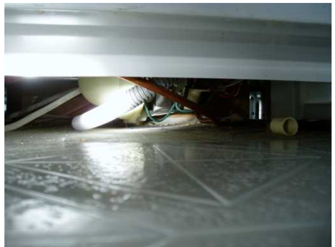
under dishwasher is dry and tight...
