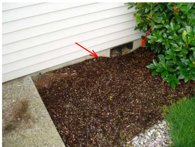
this is vent with too much barkdust and will allow rain water entry to crawl space...keep even or below vent opening
