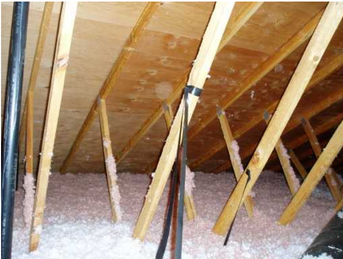
no moisture stains noted in any areas of attic...
