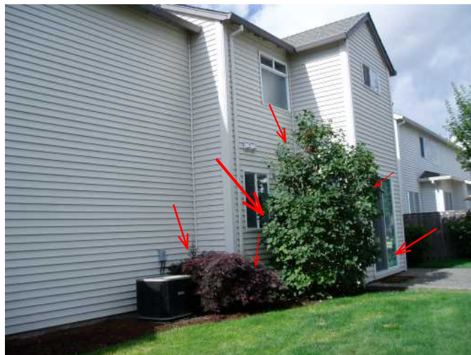
backside of home looks good..air conditioner is on level pad..good...again..trim back shrubs..to close...
