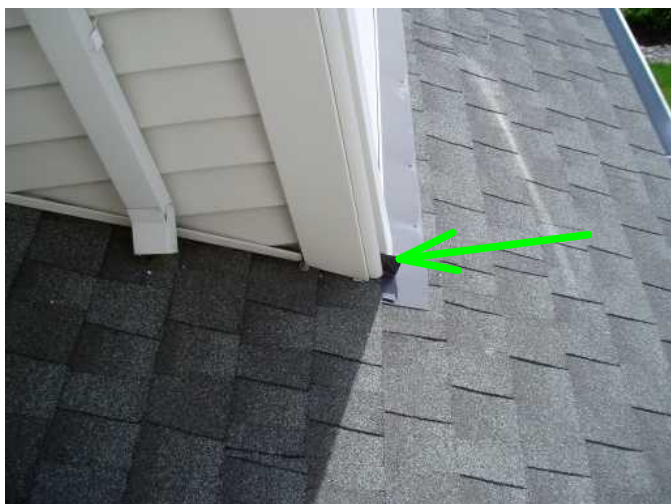
good kickout to keep water from entering under shingles in this area....
