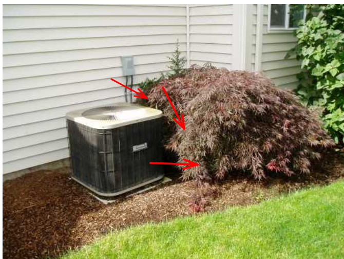
a/c unit was installed after home was built..runs fine..trim back shrub here is to close to unit to make it work harder.
