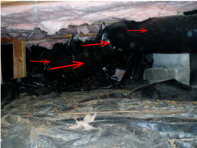
more duct work going to family room..area...good...
