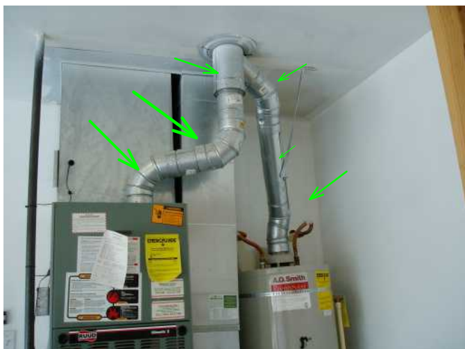
exit flus are installed well and solid....
