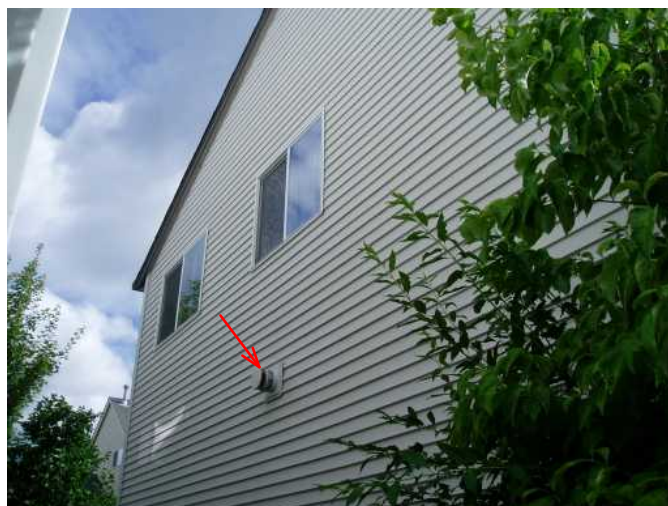
fireplace exit duct...good..siding in great shape...left side of home....
