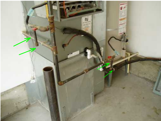
gas service to furnace and water heater are installed well and solid..have two drip legs to catch impurities in the line
