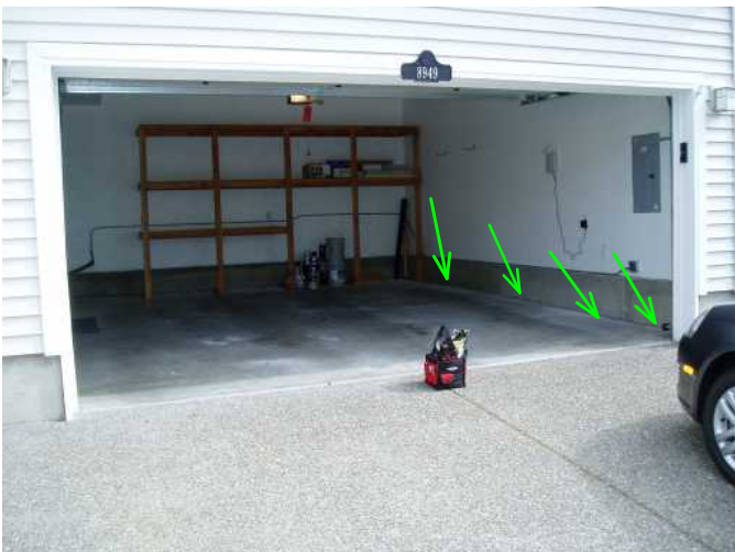
garage entry is good..see slope of floor towards front..very good...
