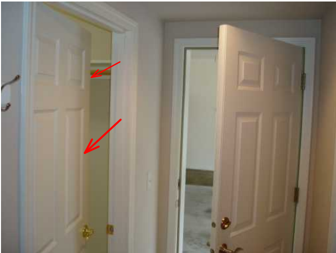
laundry room door is in good order...
