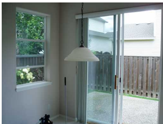
dining area windows (2) and slider are operable....
