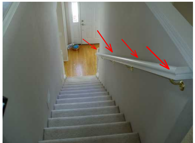
handrails to first floor are solid and sound...
