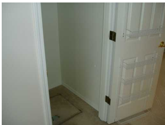
access to under stairs closet and scuttlehole to crawl space....
