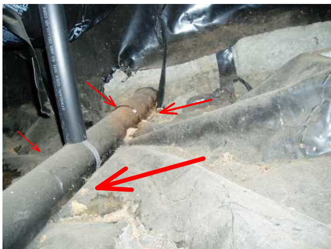
main sewer exit pipe goes out the front of home under dining room...
