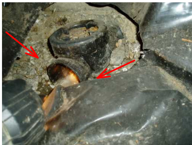
this is exit gate at low corner of crawl floor to let out any water that may enter crawl space..very good...
