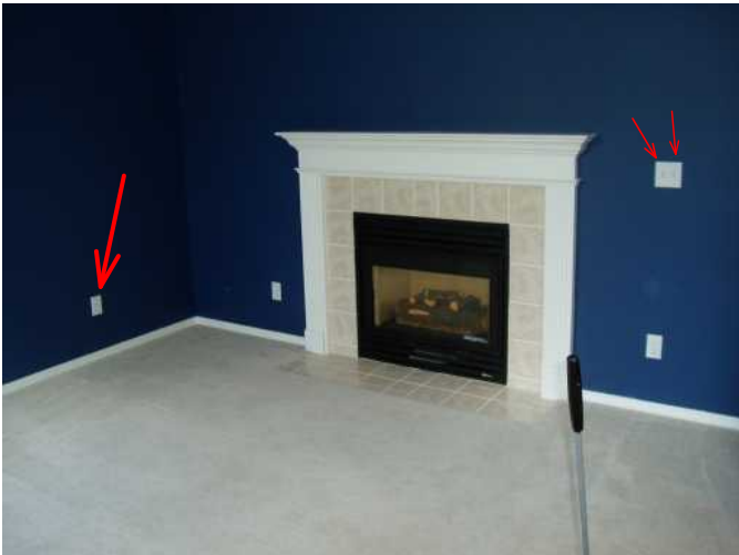
see through fireplace is operable...works fine...is wired for fan, but doesn't have one installed..outlets are switched
