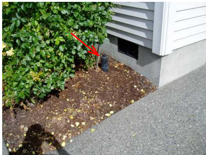
main sewer cleanout..good..
