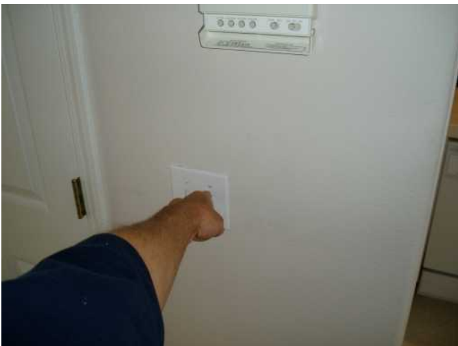
this is to remind me to tell you that when you have dimmers on three way systems they have to be on to run the other one
