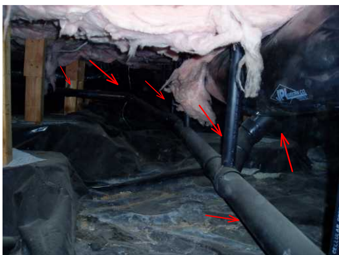
main sewer exit pipe is solid and sound with no leaks noted....
