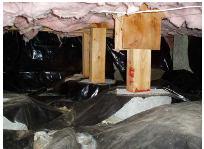
more post and beam and insulation and moisture barrier over earth to keep dampness out of your home...very good
