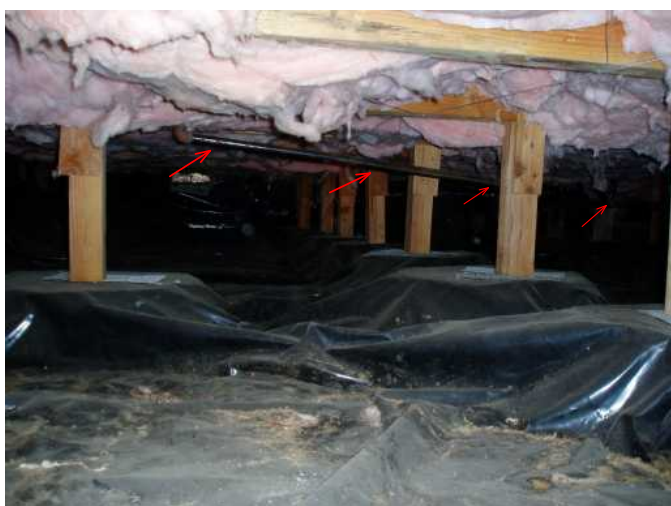
gas service to fireplace is hard piped...
