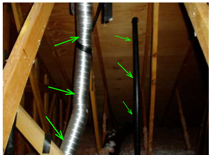
attic is plywood sheathing and 2x4 truss system...bath venting is good from both baths...one sewer vent pipe noted here.
