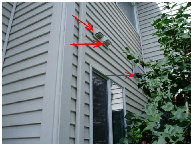
left two vents are laundry vent and bath vent/ right vent is over stove exit vent..all working fine...
