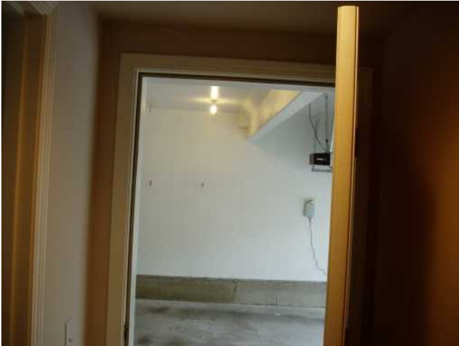
weather seal around garage door is in good condition...
