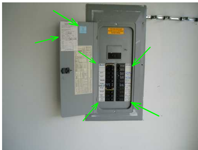
electric panel open showing well marked for zones and has permit sign off and blue tag for a/c installed later....good
