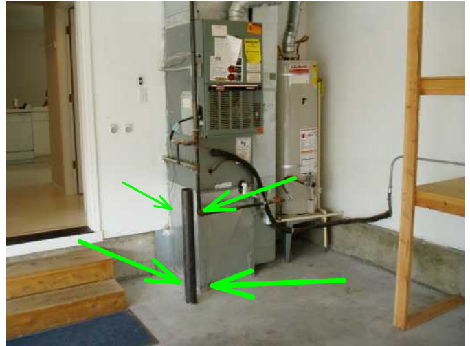
furnace and water heater have post protector in place...very good...
