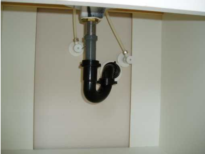
under sink had no leaks ...right master
