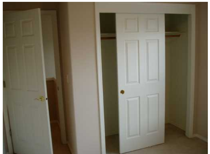
bed 3 exit door and closet doors are in good order...
