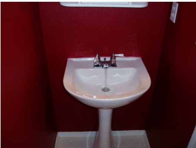
pedestal sink has no drips noted...faucet works fine..overflow works as well...
