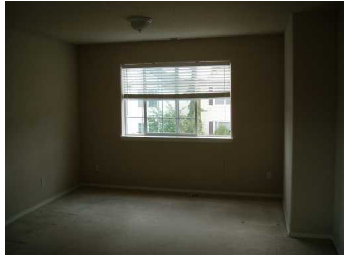
front window of great room works fine...
