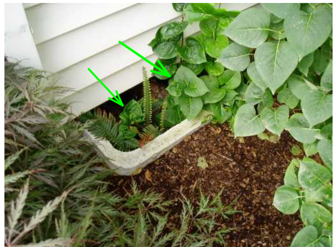
one vent in rear of home needs a little cleaning out...no big deal...
