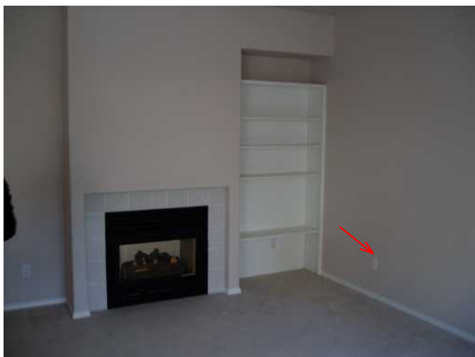
family room fireplace and shelving unit...outlets are switched for lamps...(2)
