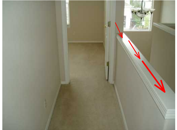
hallway to bed 2 railing is solid and sound...
