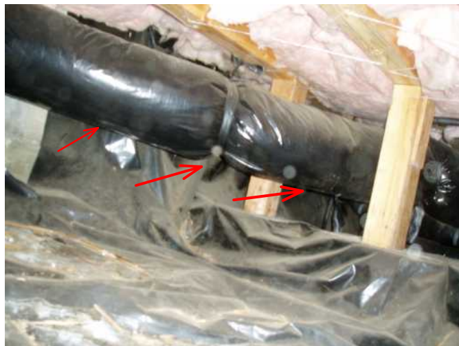
all insulated duct work is in tact and connected and performing well....
