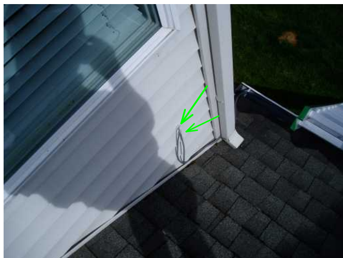
dish type television cables are installed well with grommetts to keep out water....
