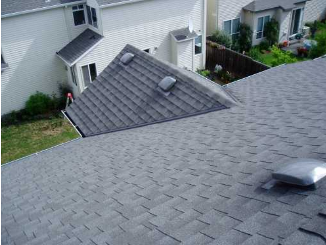
back of roof is vented well...valleys are good...
