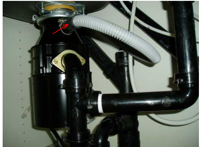
air gap for dishwasher..good...no drips here...
