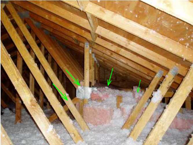
vaulted ceiling above master bedroom has batt insulation...rest of attic is blown..very good job...
