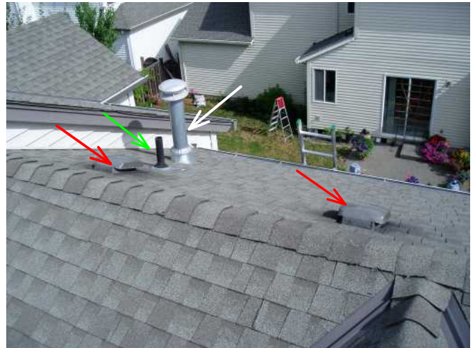
red more roof vents ...good...white ...exit flu for furnace/water heater...good...green..sewer vent pipe in action..good
