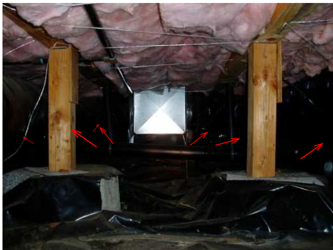
main distribution of furnace/a.c system at garage side with insulated duct running throughout crawl space....good...
