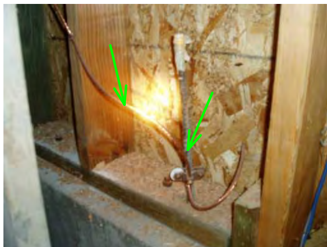
grounding is noted here at re-bar to foundaion for electric system...good is also bonded to gas lines...good...
