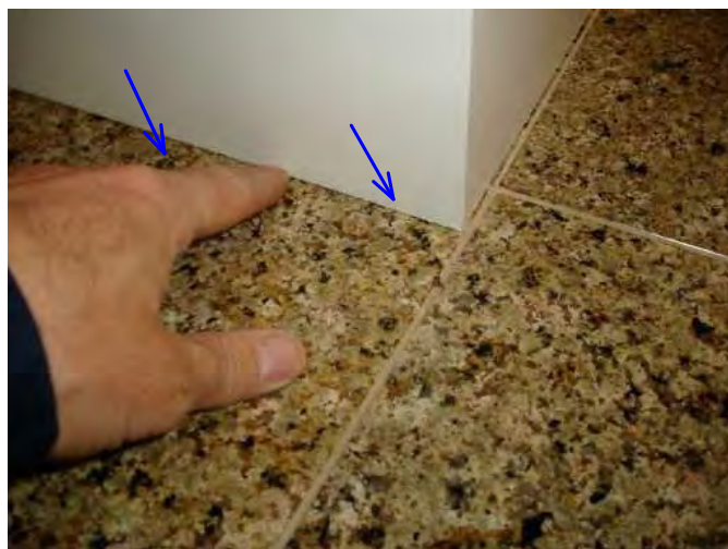
suggest caulking around wood trim at counters to avoid water entry and grime build up....
