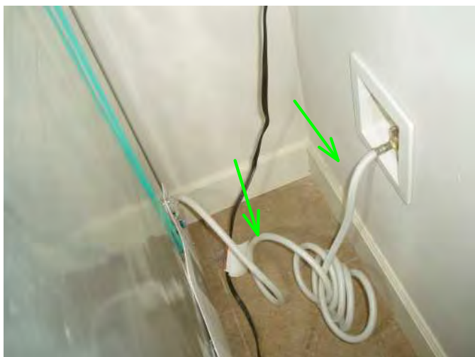
no drips or leaks noted at connections at back of refrigerator...good..
