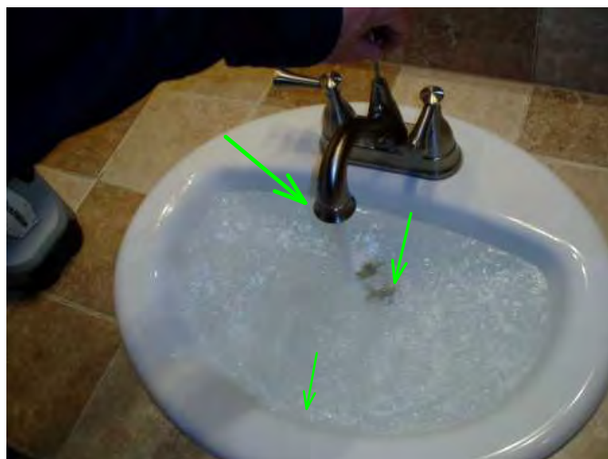
sink faucet and drain and overflow are noted operable ....good...
