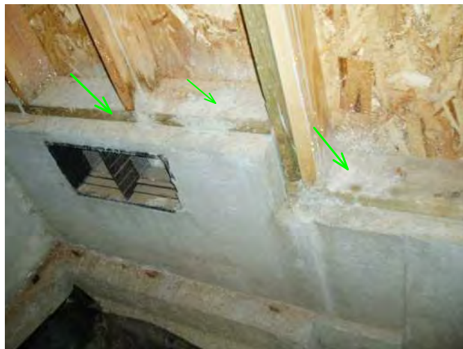
noted all rim mud sill plates are treated wood and are bolted to foundaion for earrth quake protection...very good...
