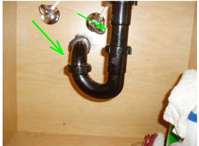
right sink drain trap is noted operable as well...good..
