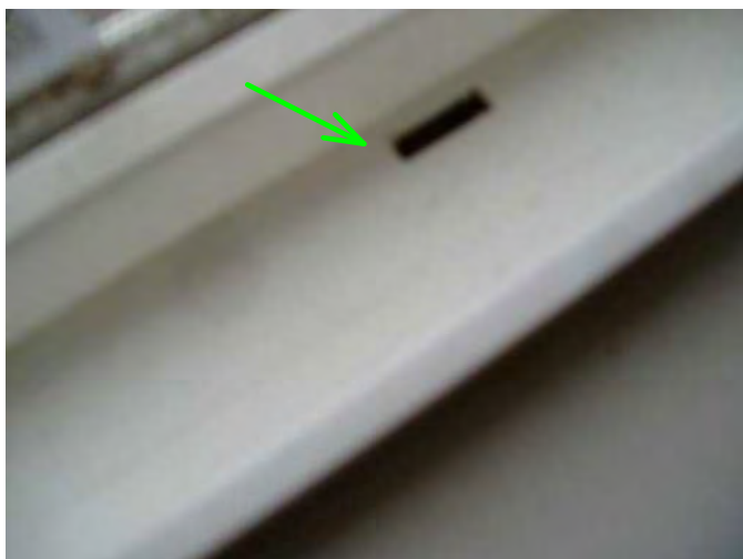
checked all windows to ensure they are installed properly....weep holes at front bottom...good..
