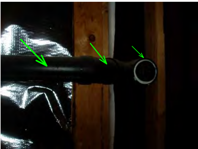
plumbing sewer pipes are noted with good slope to lower area of exit and cleanouts are noted as well...good...
