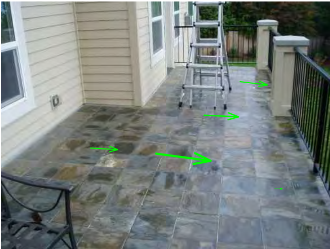
balcony is sloped well for drainage...monitor grouting and re-grout as needed...re-seal balcony every spring...
