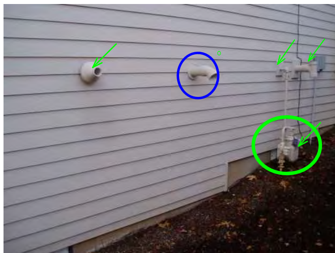
main gas meter is solid to home...PVC flues are noted for both furnaces and water heater...one needs to be re-sealed...
