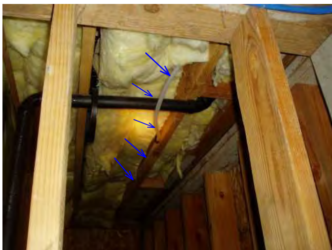
seeing random areas that pex water supply lines need to be insulated....
