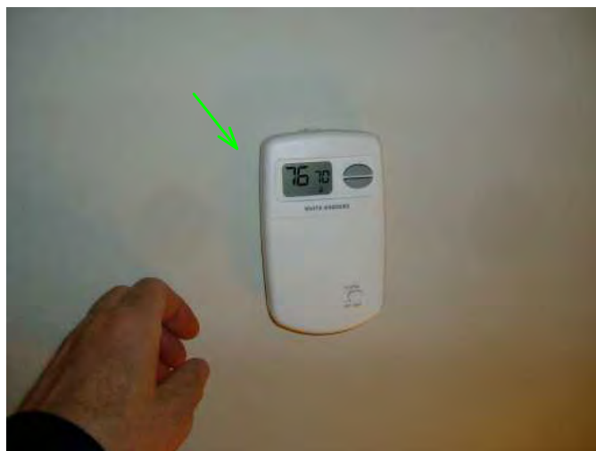
thermostat for hydronic floor heating is noted here in family room ..is operable...good..
