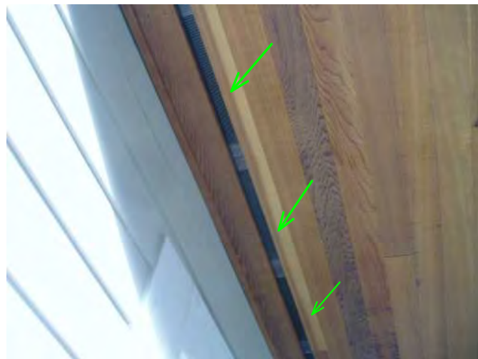
gap under balcony is noted as venting to allow any potential water that is in area can dry out...good..
