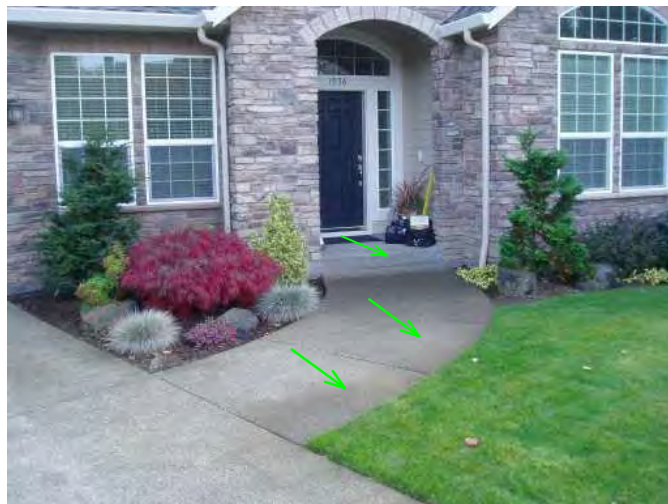
front porch and walks to porch are noted sloped well for drainage...good..
