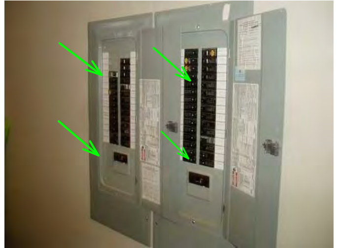
two breaker panels are noted in garage...very good...200 amps x 2 is very nice...
