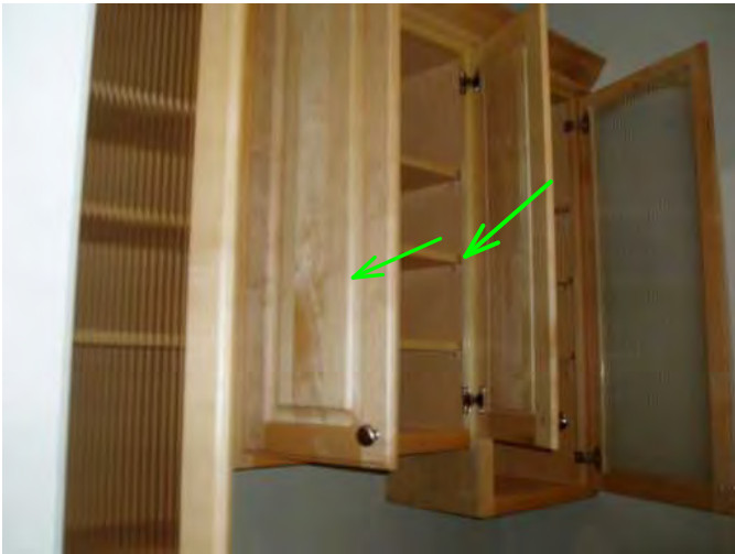
upper cabinets in butlers pantry are noted solid to walls..good...
