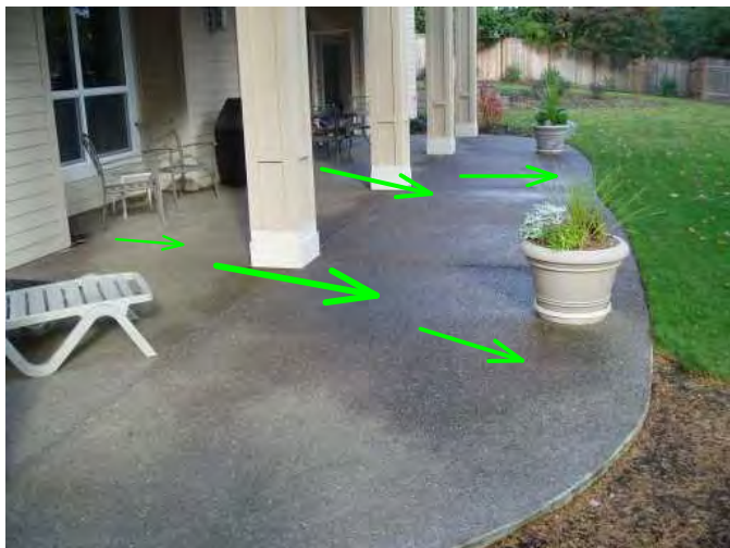
good slope of patio noted here at lower area of back yard...good..
