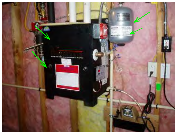
munchkin hydronic heater is noted here and is operable...good...expansion tank is noted to control water noise
