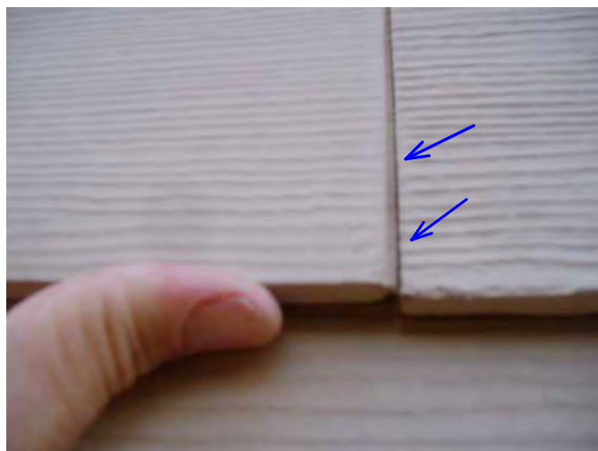
noted at random siding butt joints are loose and small gaps are forming to let in water, re-caulk as needed,ongoing item
