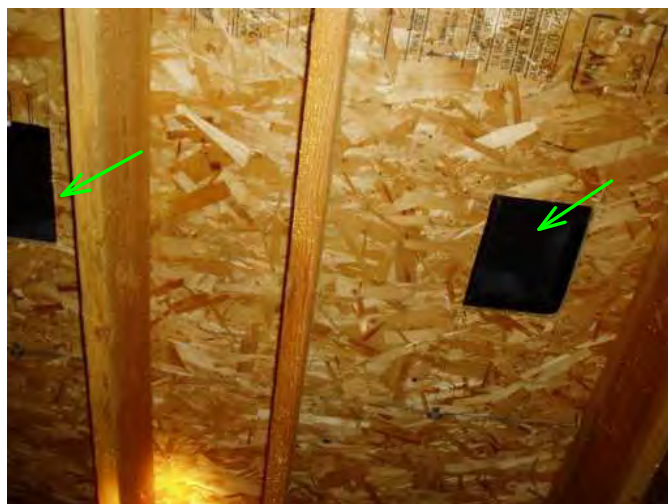
vents are noted here and are fine...good...this is upper attic area over main home area...
