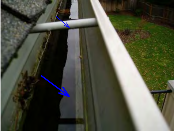
back gutter is noted full of sludge and has standing water....clean all gutters..
