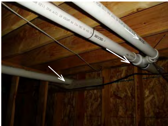
pvc flues are run to side of home and are solid to joists...good...
