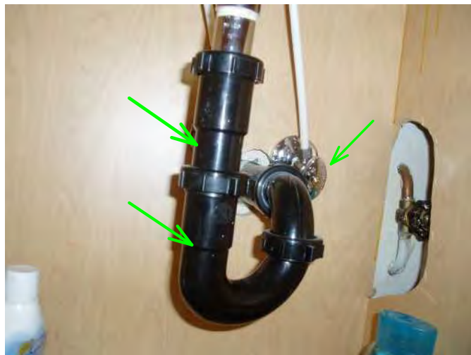
left sink trap is noted with no drips or leaks...fine...
