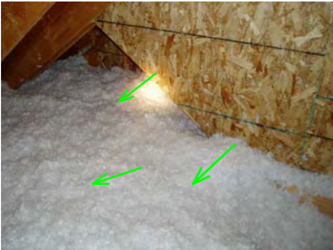
front area over dining room is noted here well insulated...good..
