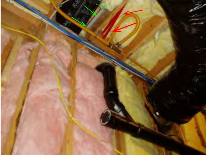
red pex is to in floor heating system in basement area...pex clear is needed to be insulated...see at green arrows...
