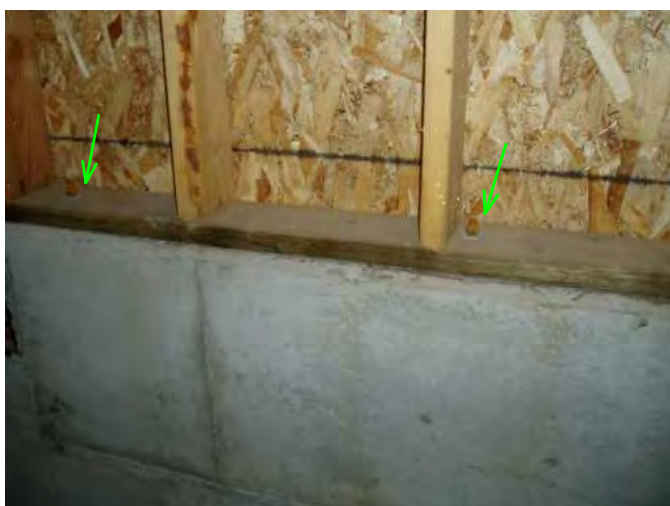
noting mud sill is treated wood under dining room area and is bolted to foundation for earth quake protection...good..
