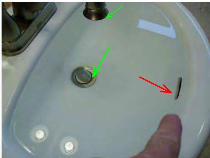
right sink at master bath overflow does not work and will overflow if left..correct drain and faucet are operable....
