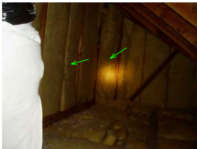
walls in attic here at noted insulated as well..good..
