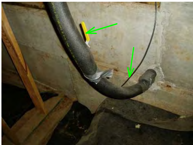
main water entry is noted here and is pex service lines...with shut off noted here...good...
