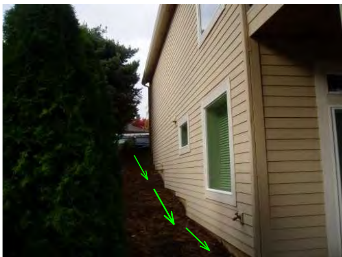
right side of home is sloped well for drainage...good..siding is noted solid to structure...monitor joints for caulking...
