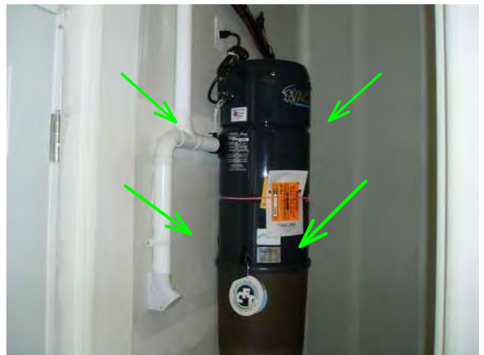
in basement area noting vacuum system is in place...and is on and operable at outlets throughou thome..no attachments
