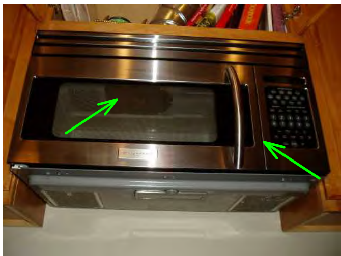
over stove microwave and exit vent are noted operable and vented to outdoors...good...
