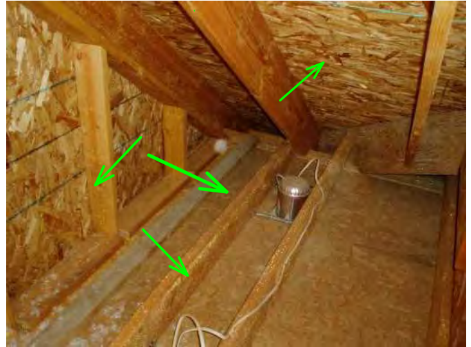
area over porch is not insulated as it is not needed...you can see recessed lights here....fine..
