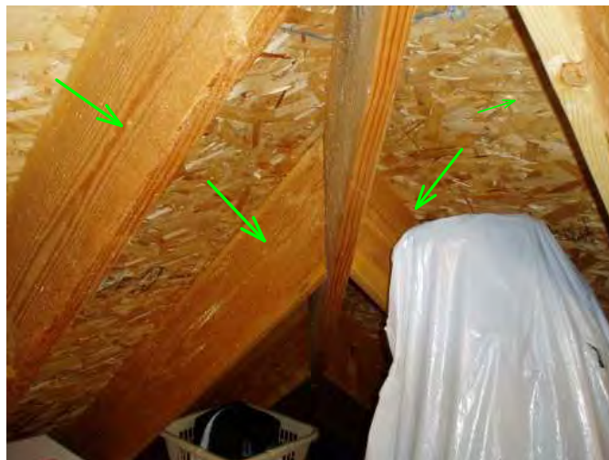
all attic rafters are 2 x 12 and are solid and sound....good..
