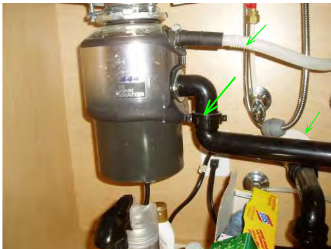
no drips or leaks detected in trap under sink area...and garbage disposer was run and is operable..good..
