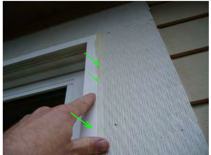
there are areas noted that gaps between trim and windows has been caulked...monitor and caulk any gaps found...
