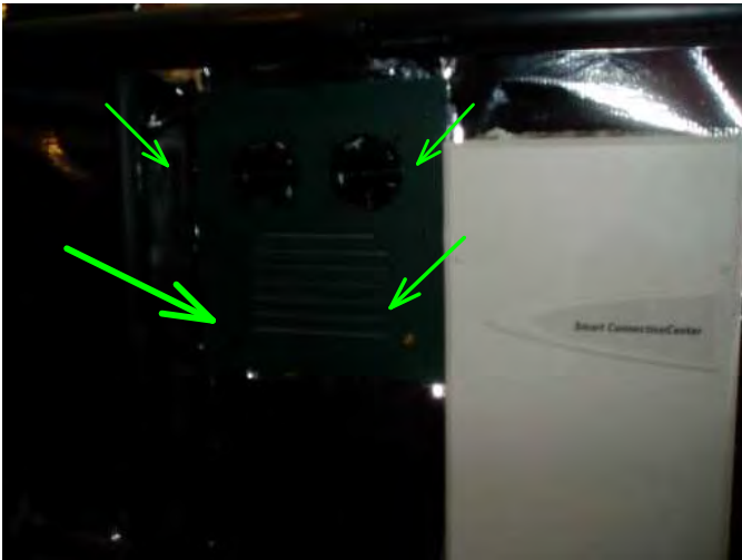
dark photo, but trying to show wine room air control system is venting into crawl area..if used..open crawl vents
