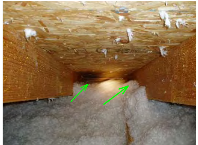
baffles are installed to keep insulation from filling in at vents at soffits...good..
