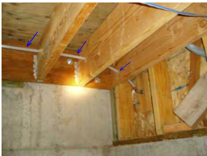
pottable pex system should be insulated....
