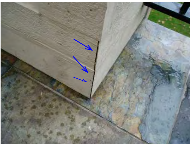
here is gap noted at column at balcony area..the wood cures and shrinks in time...monitor and seal all gaps...
