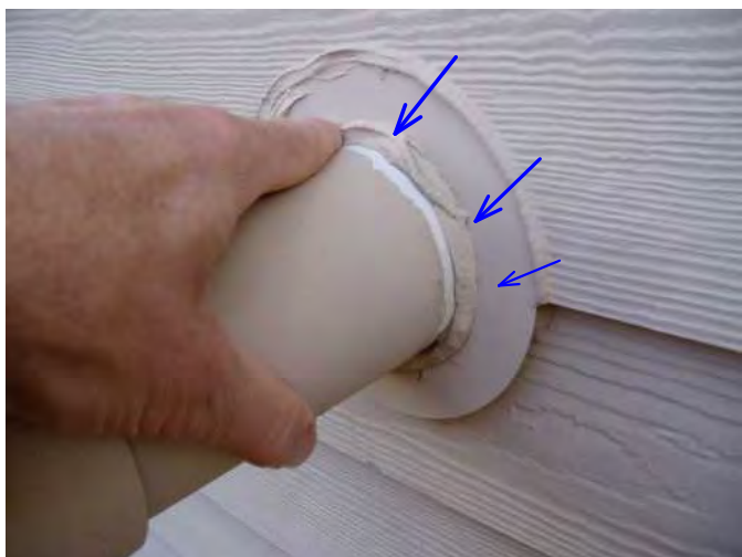
close up of affected flue that needs to be re-sealed to keepout water entry...
