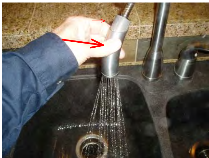
faucet is operable, but sprayer is noted stuck in faucet and needs repair....
