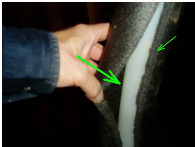
pulled back service line and showing is pex...fine...
