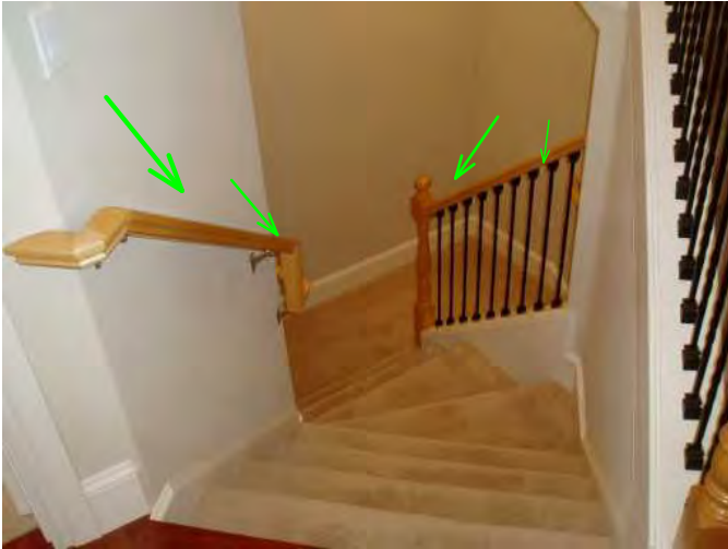
handrails to basement stairtower are noted solid to wall and in center area...good..
