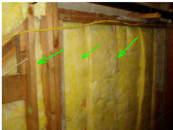
walls to basement area are insulated fine...good...
