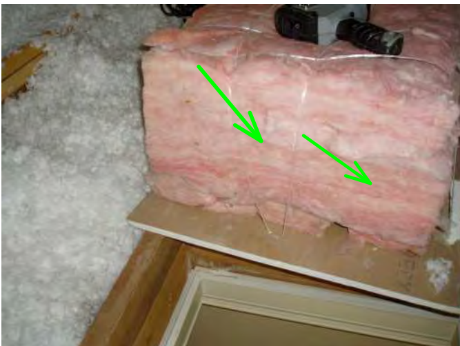
access hatch is noted with batting insulation at about 12 inches....good...
