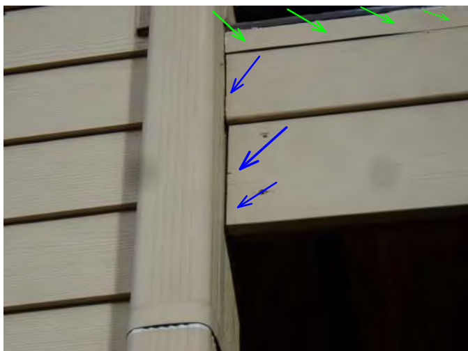
blue needs sealed at gaps...green is flashing at balcony edging and is good...
