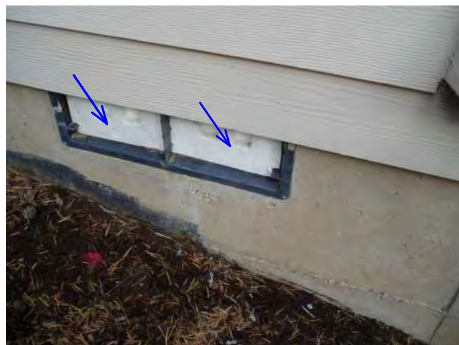
crawl vents should be left open to allow crawl area to breathe and air flow through...
